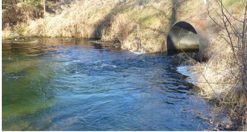
Figure 12.1 Examples of perched and high velocity conditions at culvert outfalls
