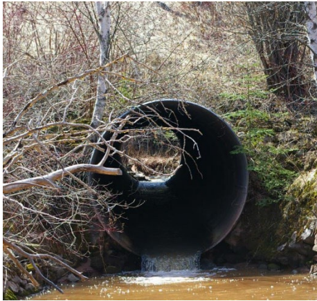
Figure 12.1 Examples of perched and high velocity conditions at culvert outfalls
