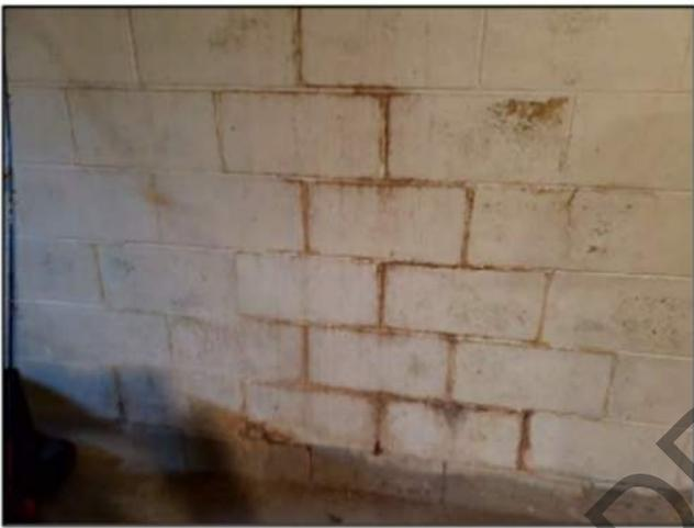
Step cracking in foundation wall
