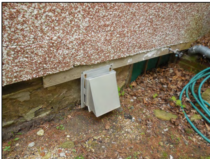
Vent for boiler
