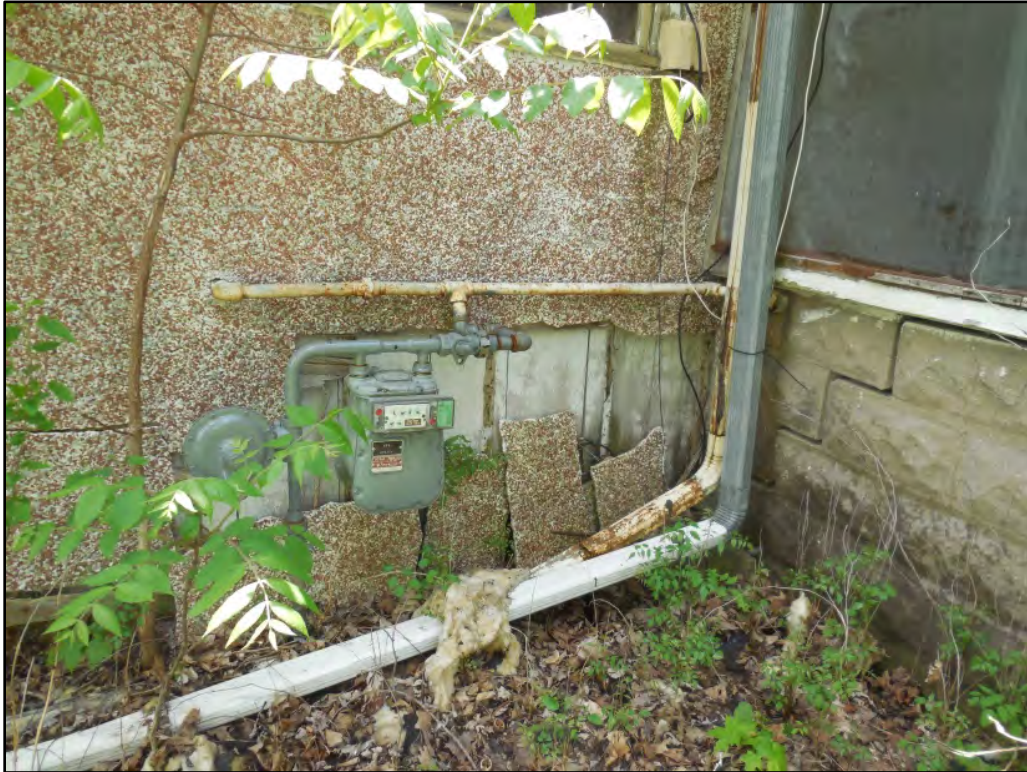
Gas meter and Stucco damage.
