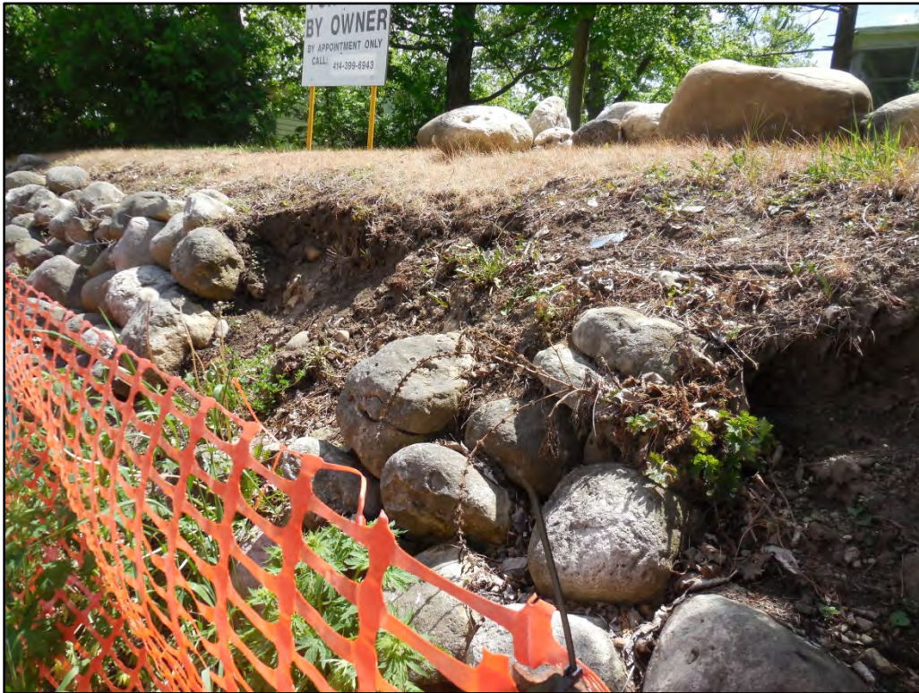
Rock retaining wall collapse along street frontage.
