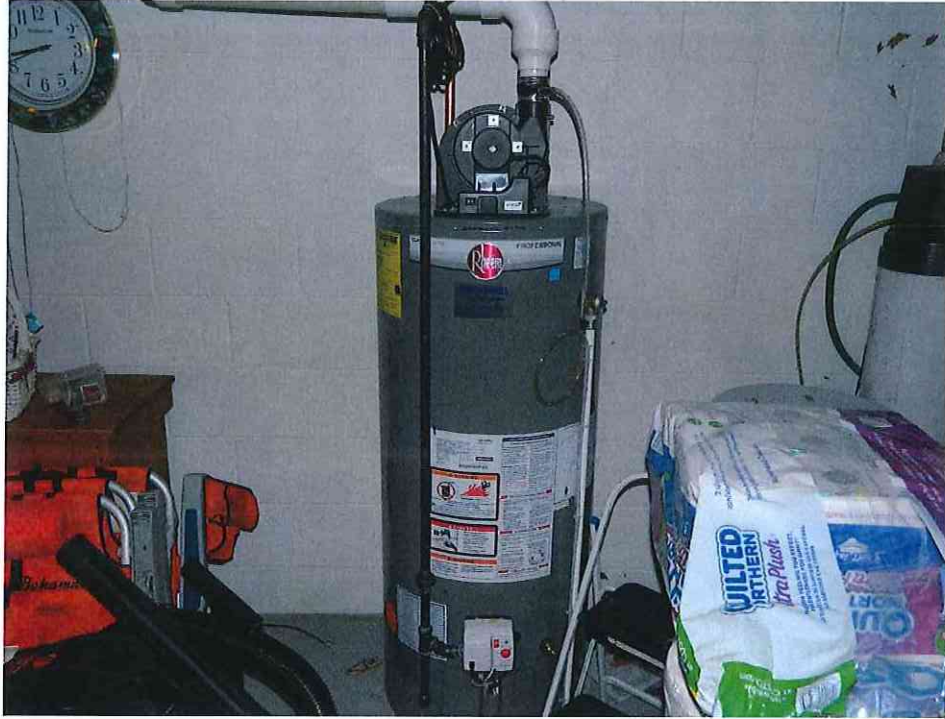
Photo 25 – New power vented water heater.
