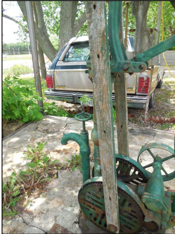
Well with pump that is motorized. Owner states the water previously pumped to a basement cistern located under the kitchen.
