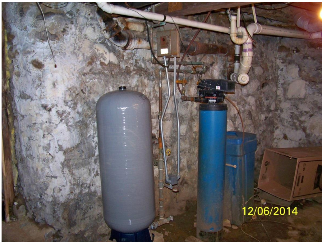
New presser tank and softener (not working per renter) in main part of basement.
