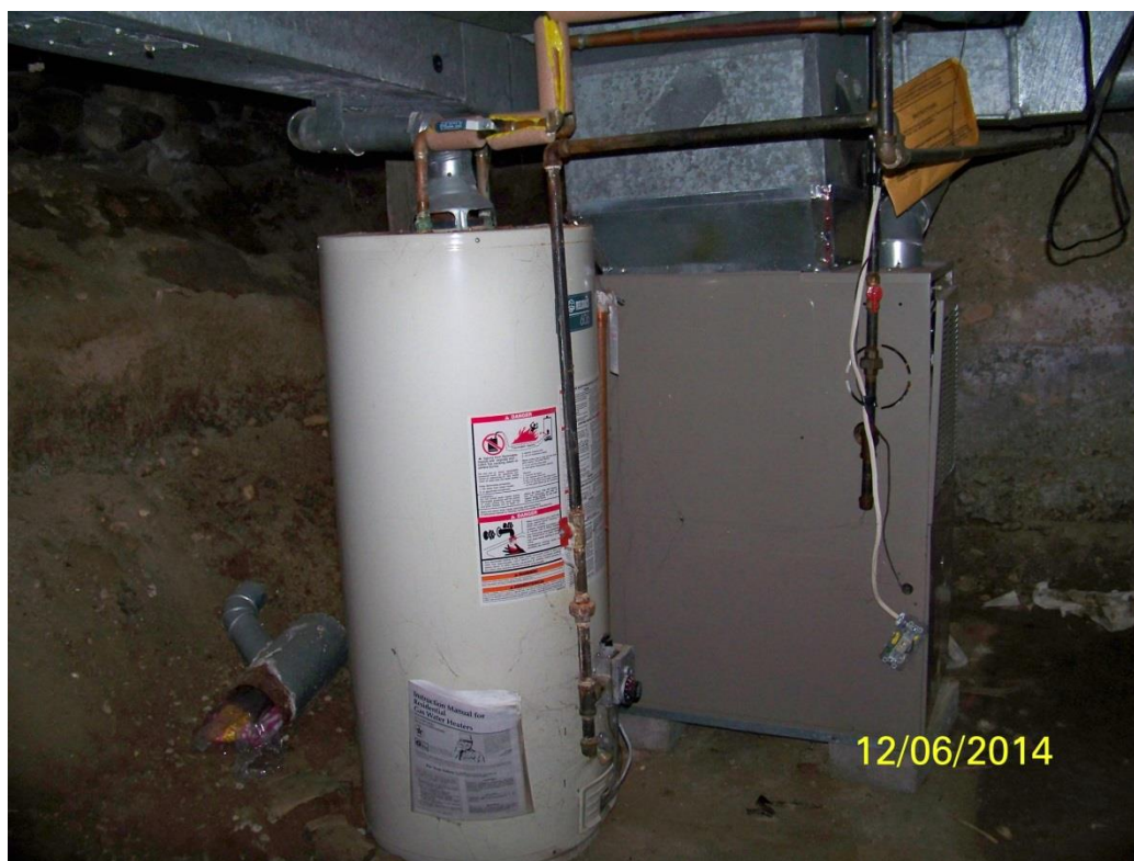
Water heater and furnace in south part of the basement.
