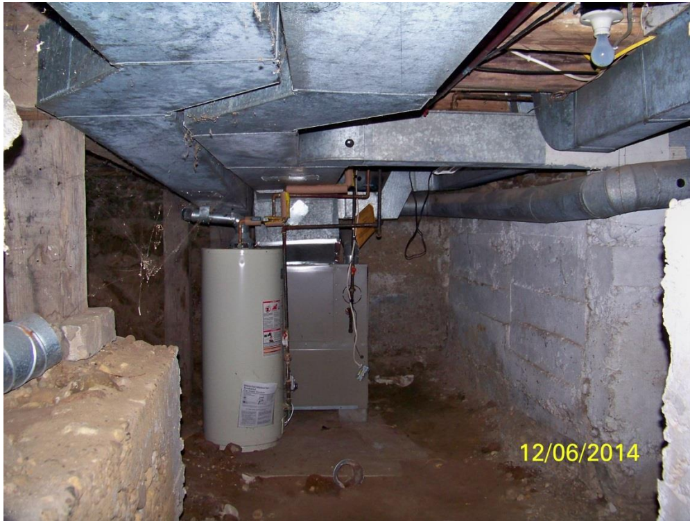
Southern part of the basement looking south towards water heater and furnace. Note-Dirt floor.
