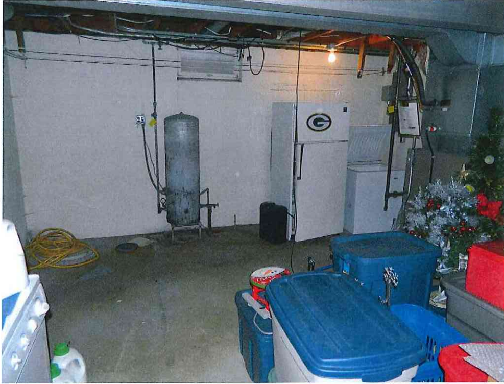
Photo 27 – Basement and Well pump/tank (4).
