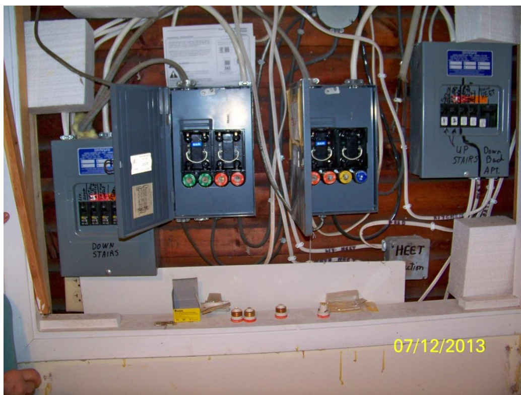
Electrical service on the north wall. Each unit has separate services of 60 amps (fuse) with subpanels of breakers.
