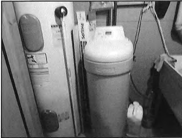
Water heater and water softener
