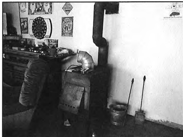
Inside garage. Wood burning stove. Vent pipe may not be to code.
