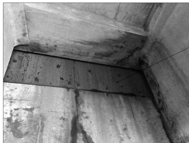
EXISTING 3/4" PLATES AT F.F. ABUTMENT, SUPPORTING ASPHALTIC FILL AT EXISTING JOINTS. REMOVE DURING JOINT REPAIR. 2 @ NORTH ABUTMENT, 1 @ SOUTH ABUTMENT. INCIDENTAL TO "JOINT REPAIR" BID ITEM.
