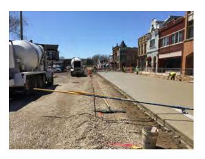
Construction started on March 4 and will last until November 1. Stage 1 is nearing completion with the final touches all underway for concrete pavement, curb and gutter, and sidewalk. Stage 2 is underway with the underground water, sanitary sewer and storm sewer. In the Spring of 2020 construction will resume to complete the final stage of construction.
