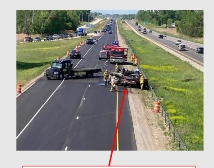
**End of Queue Crash – smart work** zone was not moved with the lane closure. The crash could have been prevented
