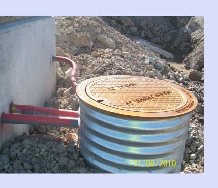
Galvanized steel covered pipe with manhole frame and solid cover.
