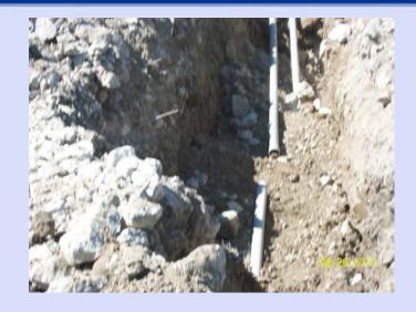
Conduits need to be protected against entry of foreign material during installation. Water can carry dirt and stones into the conduit. When back filling dirt and stones can also enter the conduit. This can cause damage to the wires when they are installed and may cause damage months or years later. During construction be sure to keep the end of conduits covered or plugged to avoid soil or rocks from entering.
