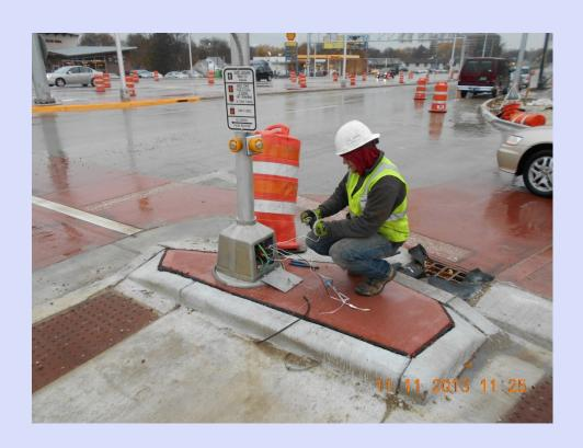
The access door of the base must be oriented away from traffic to allow maintenance personnel to see the intersection while servicing the base.
