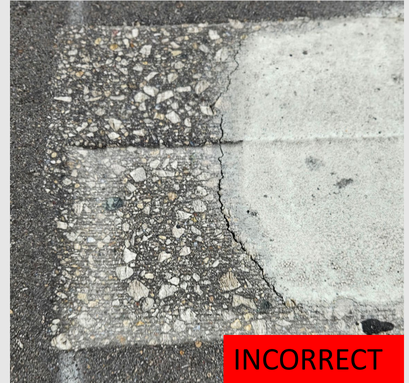
Uneven Grooves. Grooves should be consistent from one side to the other.
