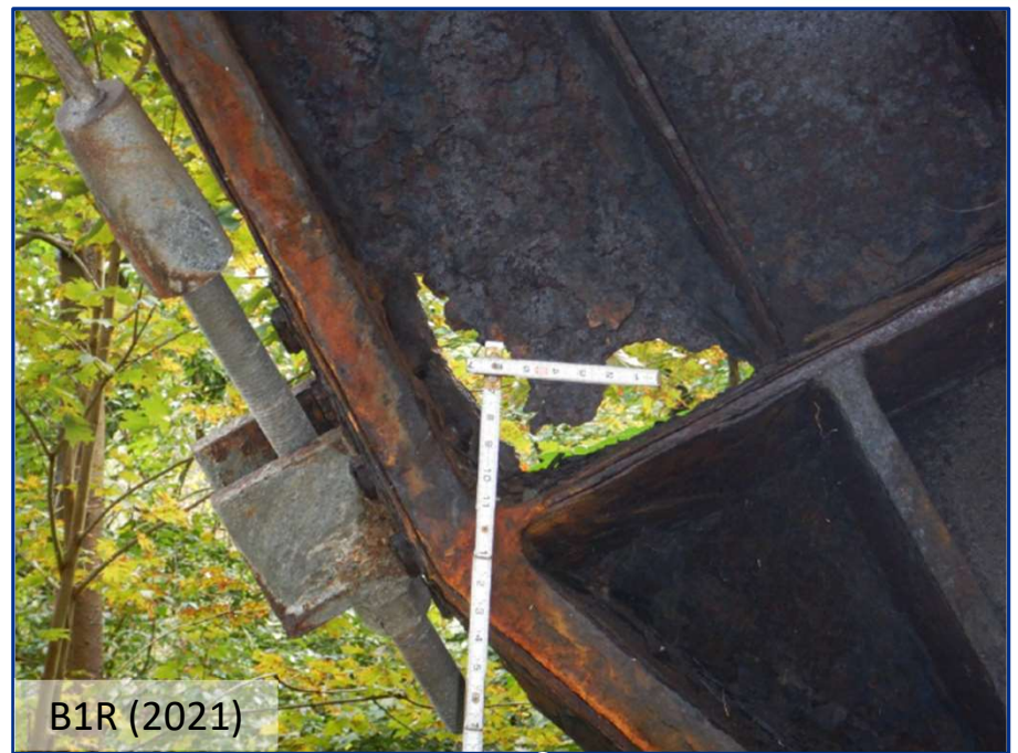
Web hole above B1R tie plate, 2013 vs 2021
