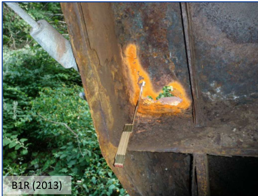
Web hole above B1R tie plate, 2013 vs 2021
