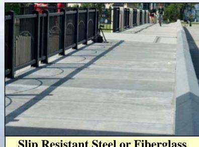
Slip Resistant Steel or Fiberglass Plate
