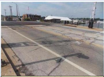
**Deck over Machinery & Counterweight Pits**
