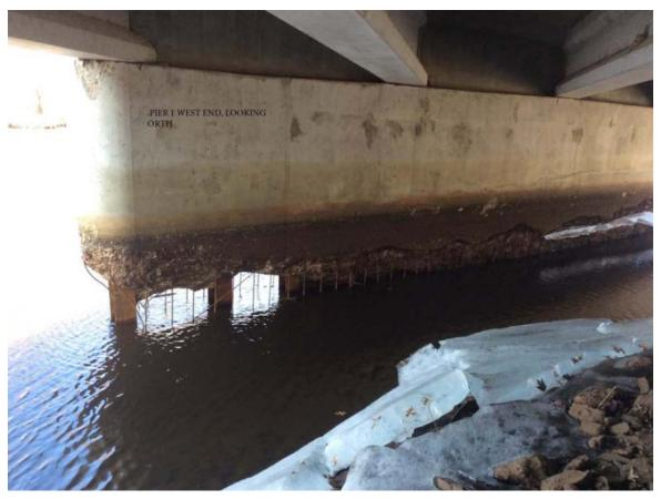
Pile Encased Pier – Tremie Poured (Assumed Unprotected)
