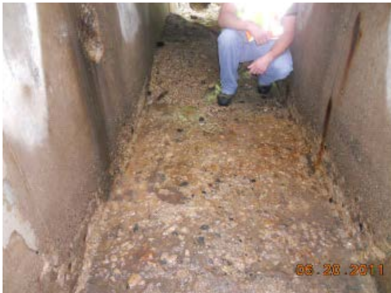
Degradation of Floor Concrete below Roadway Inlet
