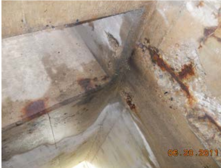
Spalls and Exposed Rebar below Roadway Inlet
