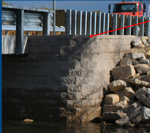
90-deg corner (LET Plans) Curved corner – (WisDOT accepted shop drawings)
