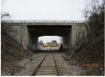
In general, rigid frames are distinguished from arches by their design. Arches are designed for compression along the entire cross-section. Rigid Frames are designed for bending and have negative moment steel incorporated in the transition from the vertical walls to the horizontal slab. An example of an arch structure is on the left, and a rigid frame structure is on the right.
