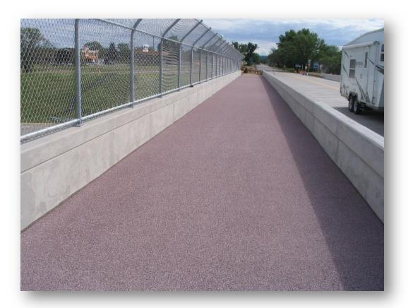
In situations where only the TPO is applied on a multiuse path separated by a barrier code both the wear surface of the traffic and one for the multiuse path separated by a barrier should be included in the inspection.
