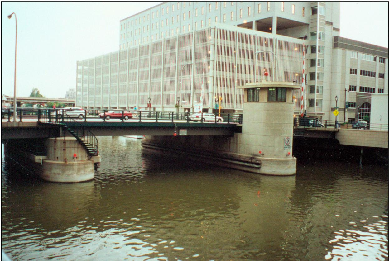
**Figure 3.3.5.1-1:** Balanced Pit Drive Vertical Lift, Michigan Street Bridge in Milwaukee.
