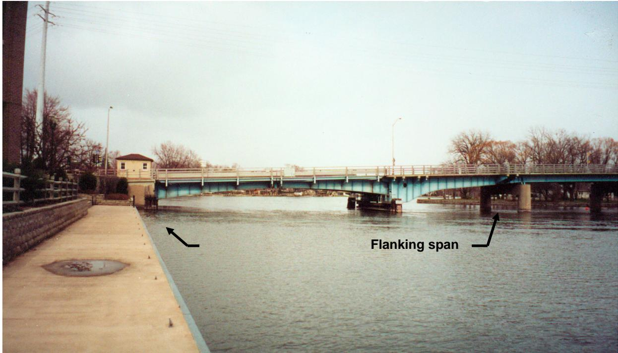
**Figure 3.2.3-3:** Double-Leaf Rolling Lift Bascule, Racine Street Bridge in Menasha.
