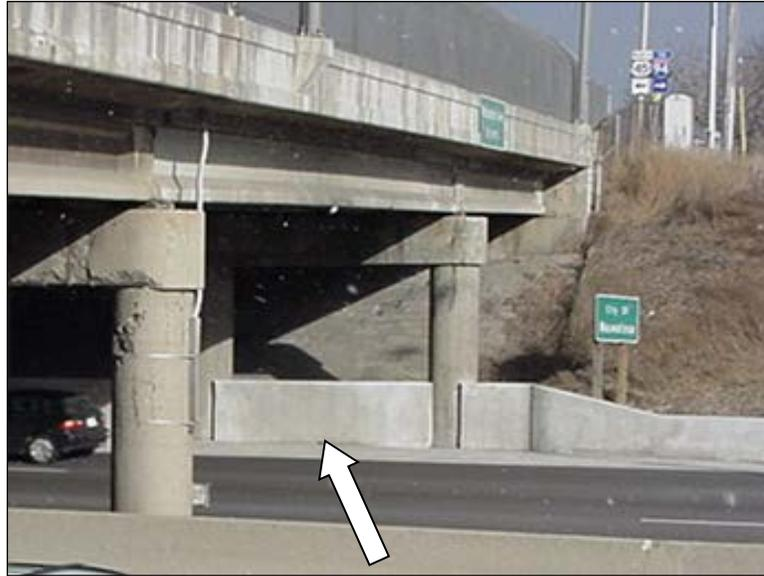
**Figure 2.9.3.5-1:** Concrete Crash Wall Along an Overpass Bridge Pier.
