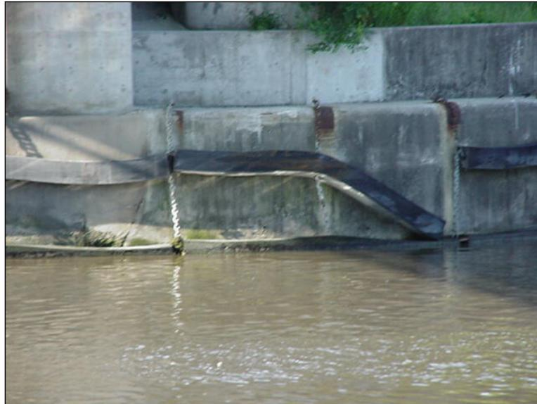
**Figure 2.9.4.3-1:** Failed Rubber Fender System.
