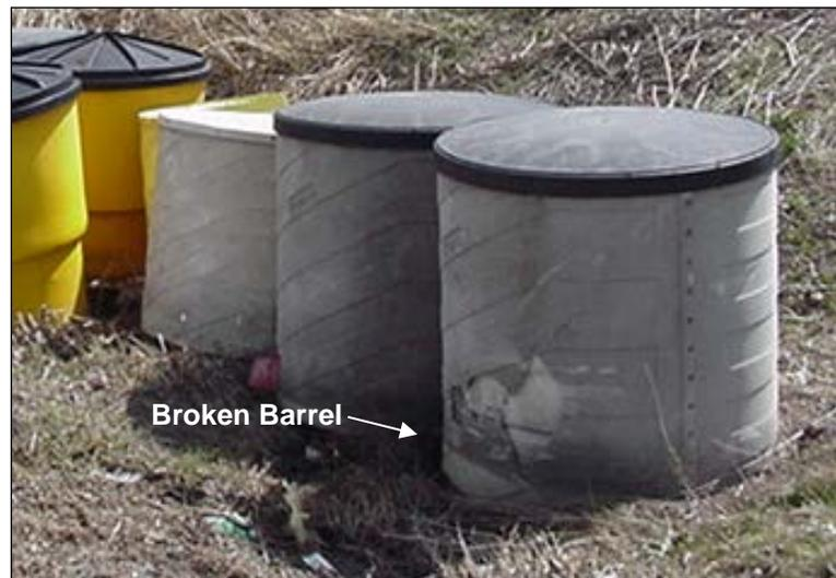
**Figure 2.9.5.3-1:** Damaged Impact Attenuator.
