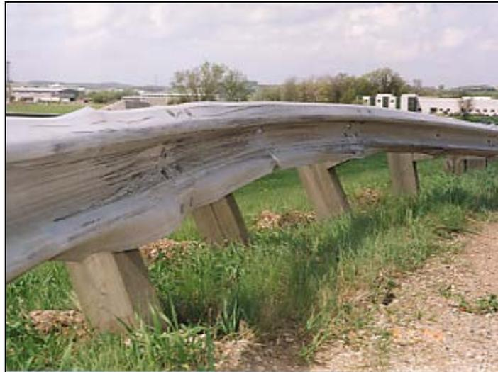
**Figure 2.9.5.2-1:** Beam Guard that was Damaged During a Collision.
