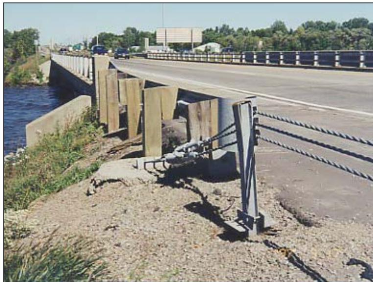
**Figure 2.9.5.1-1:** Cable Guard Next to a Beam Guard.
