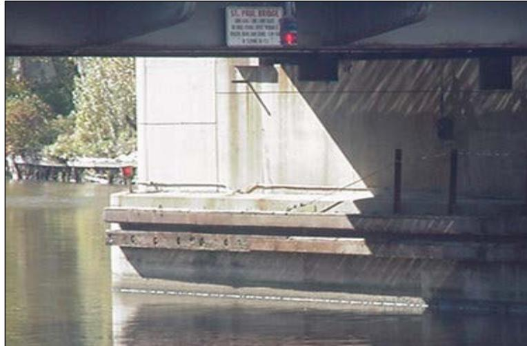
**Figure 2.9.2.3-2:** Substructure-Supported Timber Fender System.
