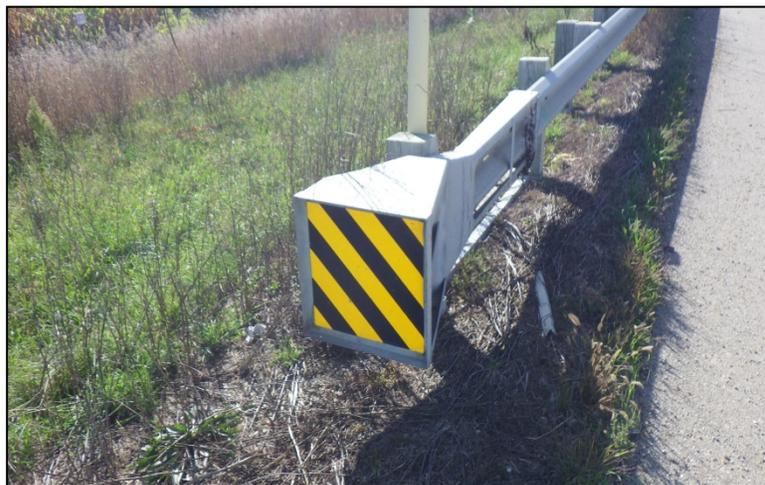
**Figure 2.9.3.2-1:** Newly Installed Beam Guard.
