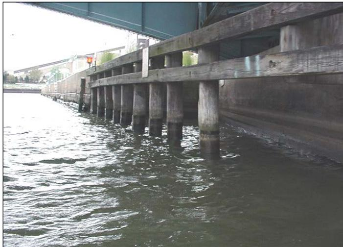
**Figure 2.9.2.3-1:** Independently Supported Timber Fender System.
