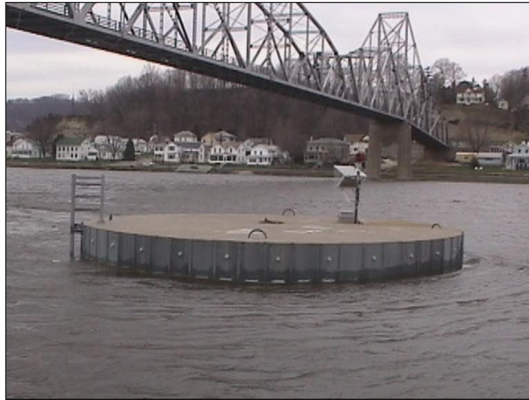
**Figure 2.9.2.1-1:** Cell Dolphin During Flood Conditions.
