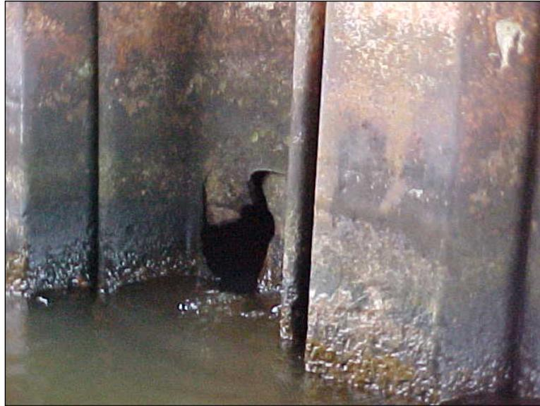
**Figure 2.9.4.1-1:** Cell Dolphin Deterioration.
