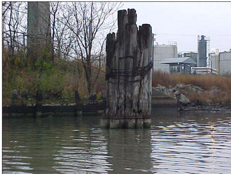
**Figure 2.9.4.2-1:** Pile Cluster Dolphin Deterioration.
