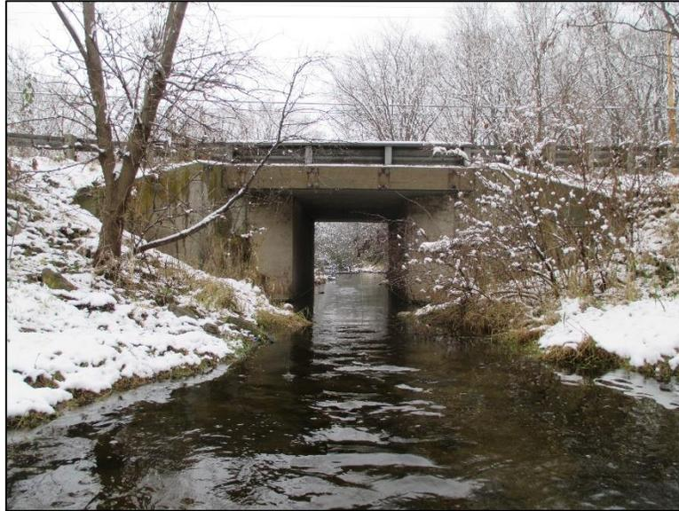
Figure 4.6.3-2: A bridge like structure with total length less than 20 ft. This structure is designated as a small bridge in HSI, and inspected with bridge elements.
