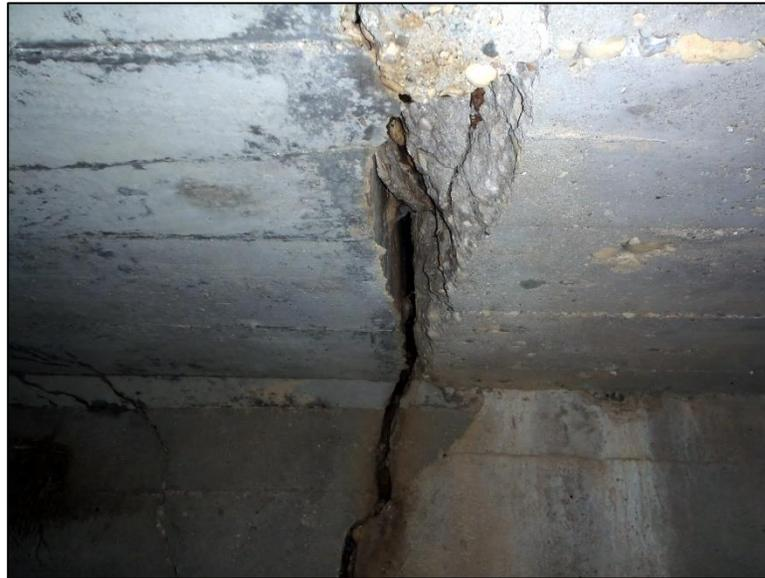
Figure 4.6.6-9: Joint Separation Between Pipe Segments – Settlement Condition State 3.
