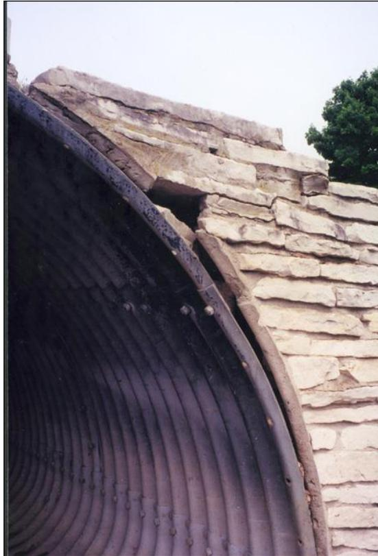
Figure 4.6.7-2: Masonry headwall separating from the barrel.
