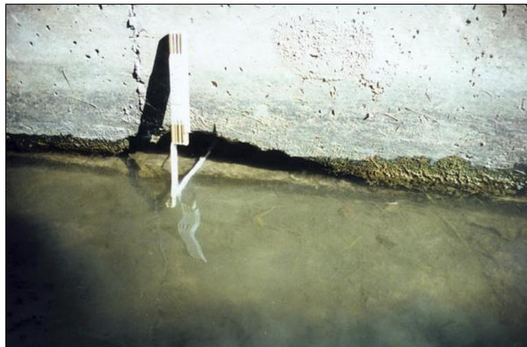
Figure 4.6.7-3: Through thickness section loss at water line of wall separating two cells.
