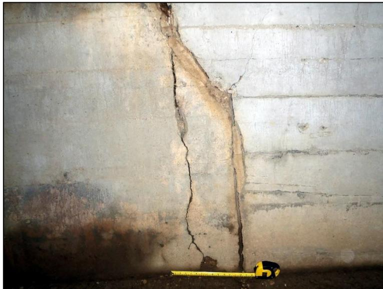
Figure 4.6.6-8: Differential Settlements Between Box Segments – Settlement Condition
