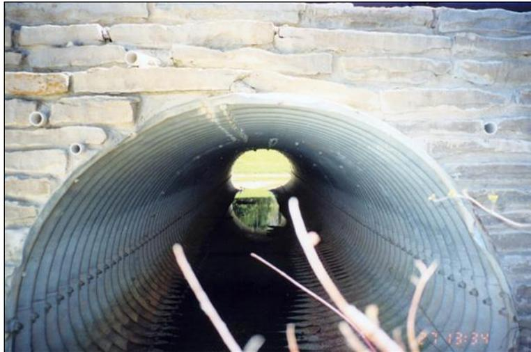
Figure 4.6.6-1: Barrel with good alignment - Condition State 1.
