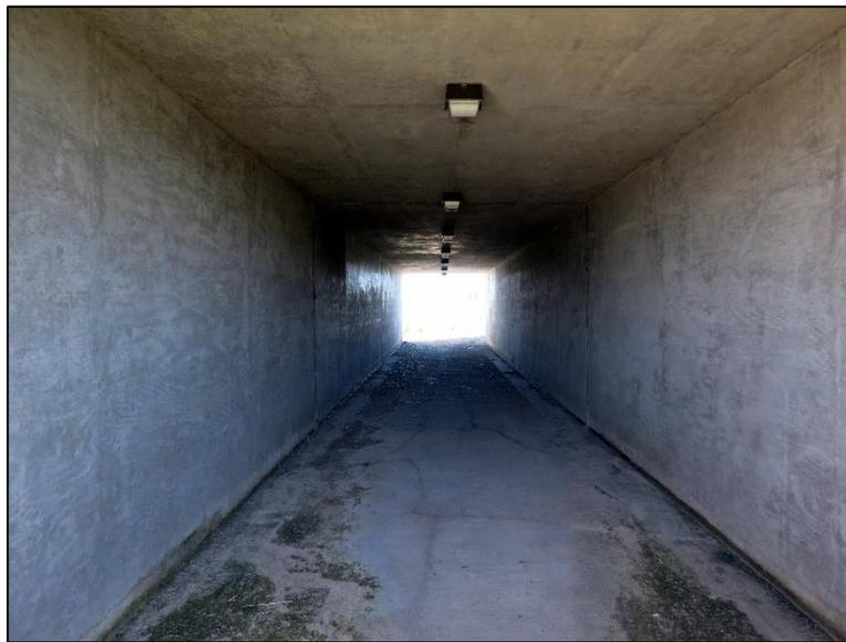
Figure 4.6.6-6: Reinforced Concrete Culvert - Condition State 1.
