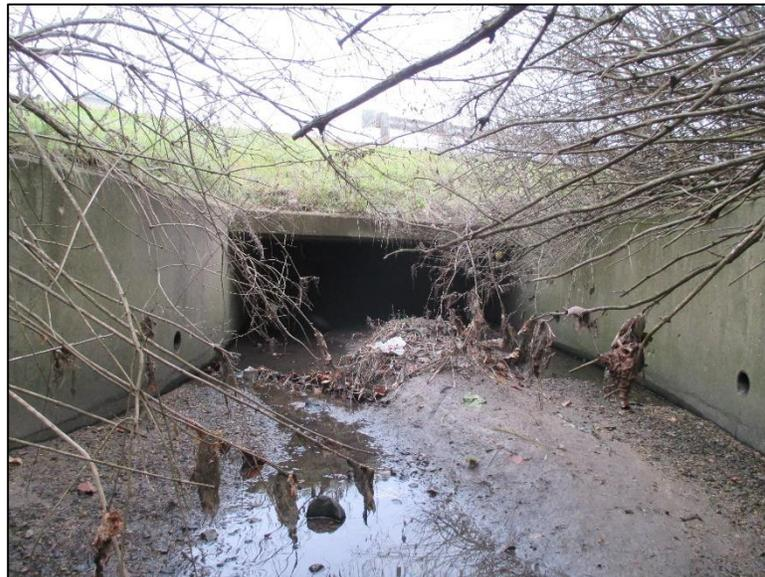
Figure 4.6.6-13: View of Retaining walls extending beyond limits of integral wingwalls.
