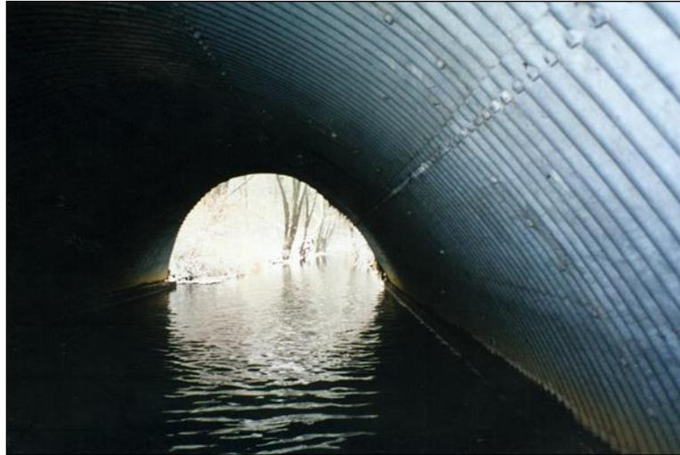
Figure 4.6.6-5: Severely distorted barrel – Distortion Condition State 4.
