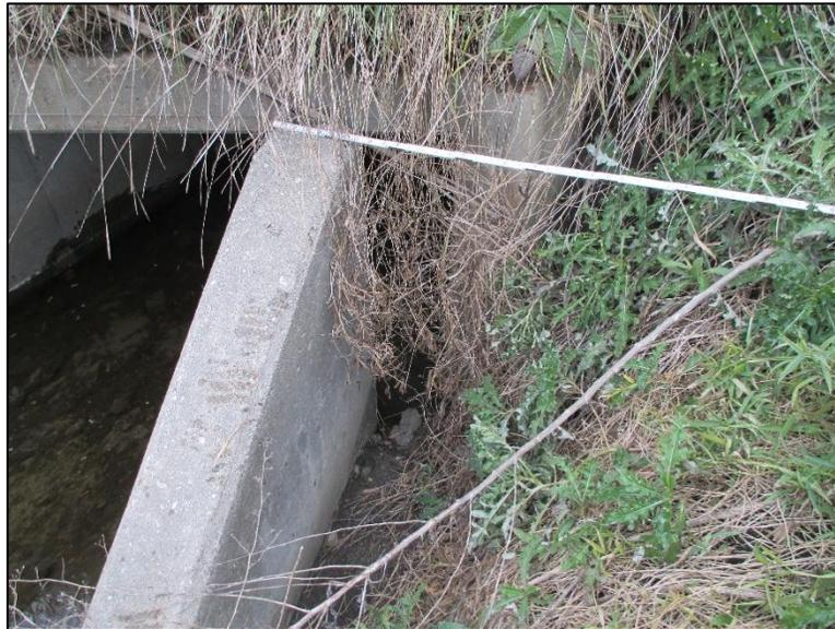
Figure 4.6.6-14: View of Wingwall Movement. Note loss of fill behind wingwall and culvert barrel – Condition State 3.
