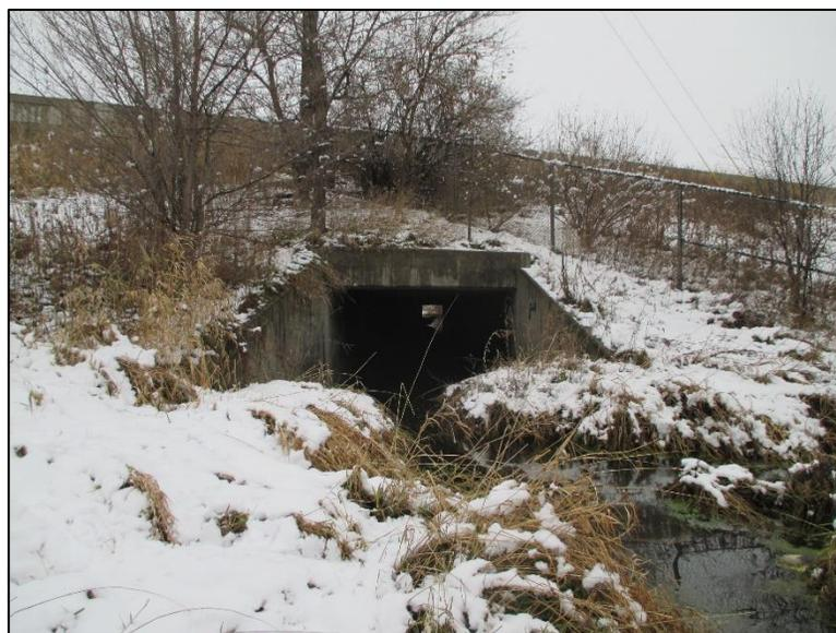
Figure 4.6.4-3: View of a single cell reinforced concrete box culvert.
