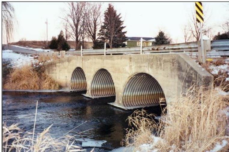
Figure 4.6.6-2: Surface corrosion near the waterline – Corrosion Condition State 2.
