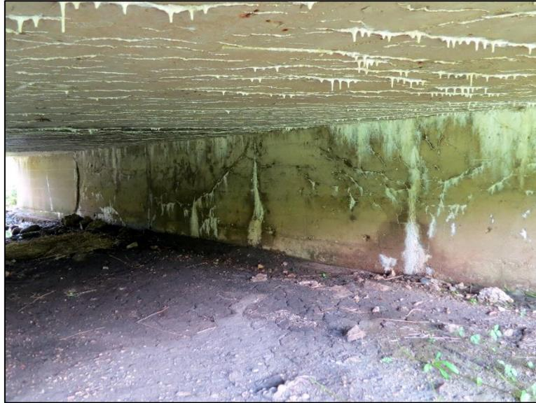
Figure 4.6.6-7: Deterioration on Culvert Wall – Heavy Density Cracking with Efflorescence
