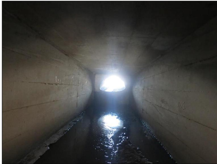
Figure 4.6.4-5: View of reinforced concrete single cell box culvert with corrugated steel pipe arch extension
