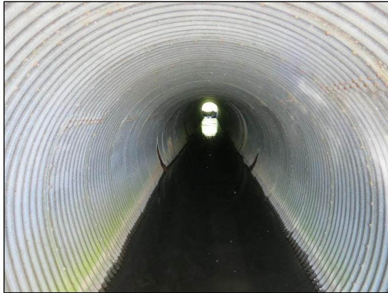
Figure 4.6.4-1: View of circular structural plate pipe culvert.
