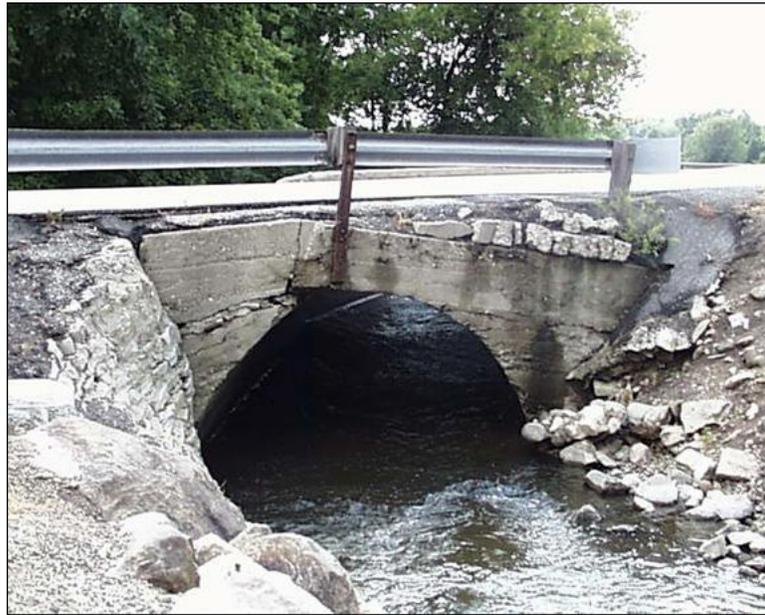
Figure 4.6.7-1: Concrete headwall failure. Note: Headwall deterioration would be captured under Assessment 9248 – Culvert End Treatment
