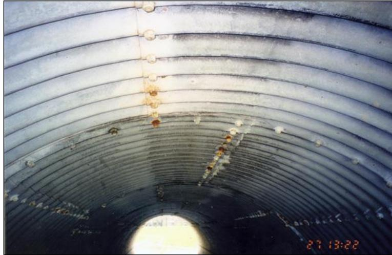
Figure 4.6.6-3: Light to moderate bolt corrosion – Connection Condition State 2.
