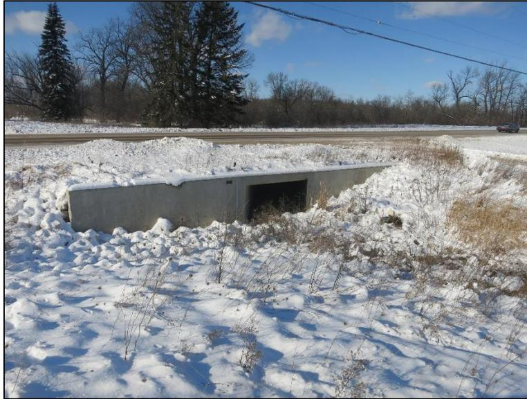
Figure 4.6.6-12: View of Integral Wingwalls Parallel with Roadway.
