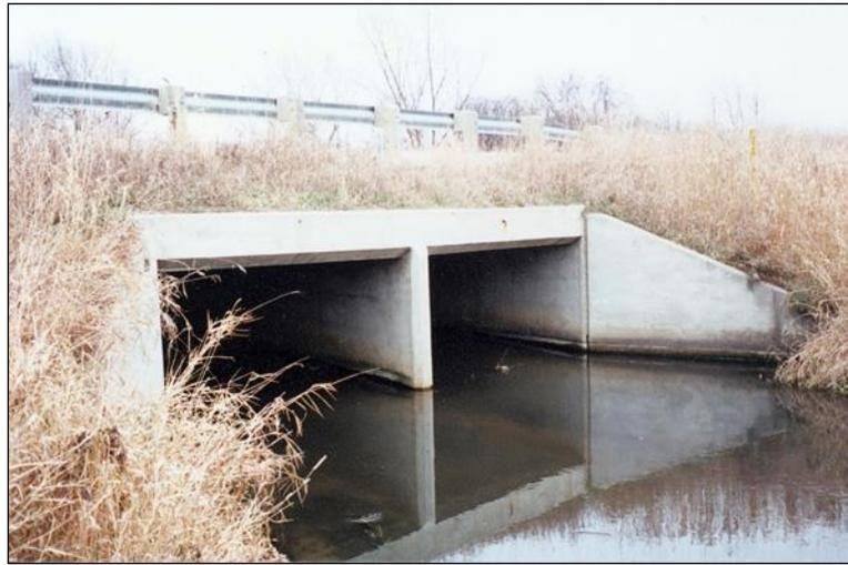
Figure 4.6.4-4: Two-cell reinforced concrete culvert.
