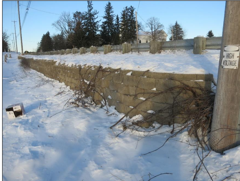
Figure 4.4.4-5: Segmented Modular Block Gravity Wall.
