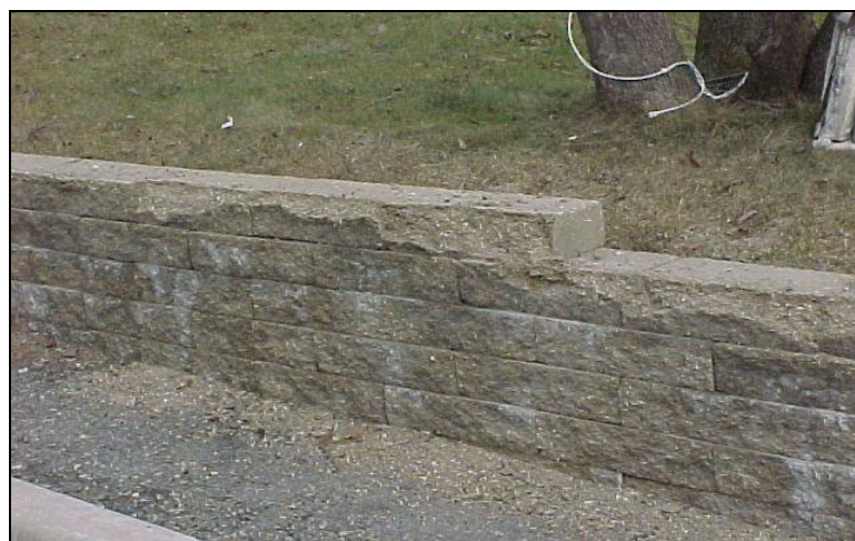
Figure 4.4.2-16: White Precipitate Formed due to Efflorescence.
