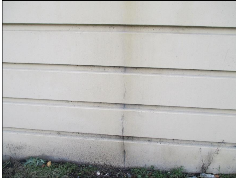
Figure 4.4.2-21: Vertical Crack Through Precast Concrete Panel.
