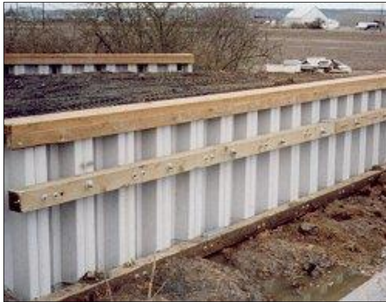
Figure 4.4.4-17: Vinyl Sheet Piling Retaining Wall.
