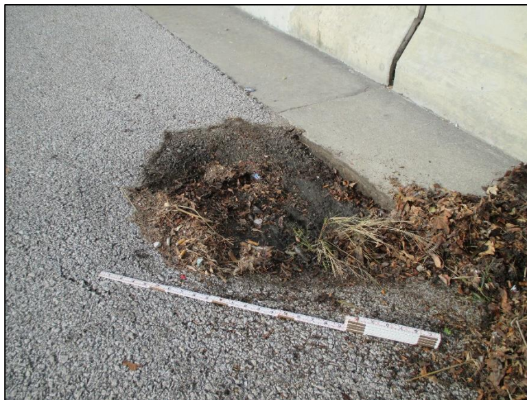
Figure 4.4.5-12: Pothole Due to Loss of Fill Within Shoulder Gutter Pan Along Top of Retaining Wall.
