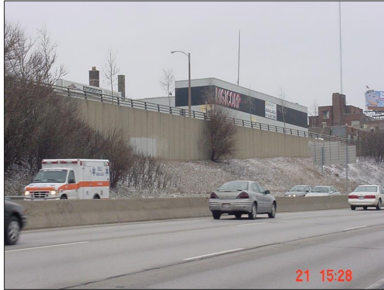
Figure 4.4.4-2: Cast-in-Place Concrete Cantilever Wall.
