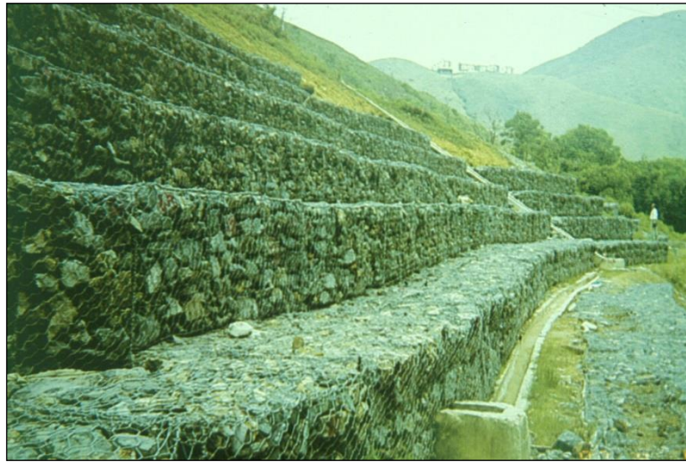
Figure 4.4.4-4: Tiered Gabion Gravity Crib Wall.
