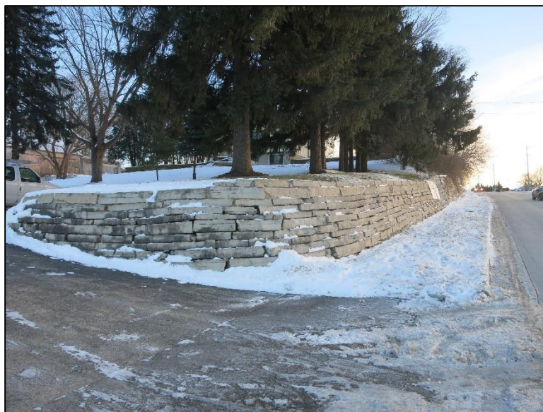
Figure 4.4.4-6: Lannon Stone (Limestone) Block Gravity Wall.
