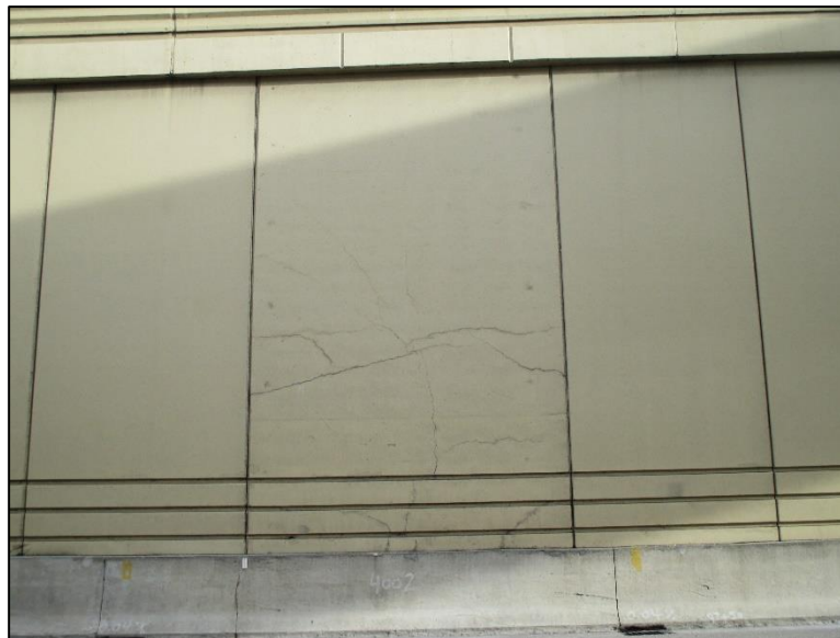
Figure 4.4.4-16: Excessive Cracking within Secant Wall Facade Concrete Panel.
