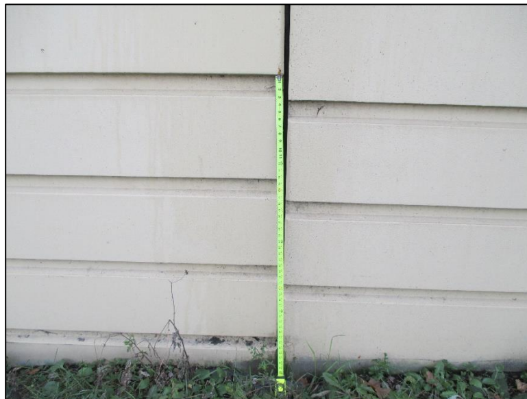
Figure 4.4.2-8: View of Differential Settlement between Precast Concrete Panels. Note Misalignment in Rustication.
