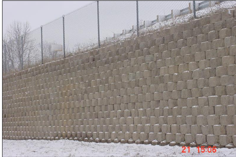
Figure 4.4.4-7: Segmented Modular Block MSE Wall.
