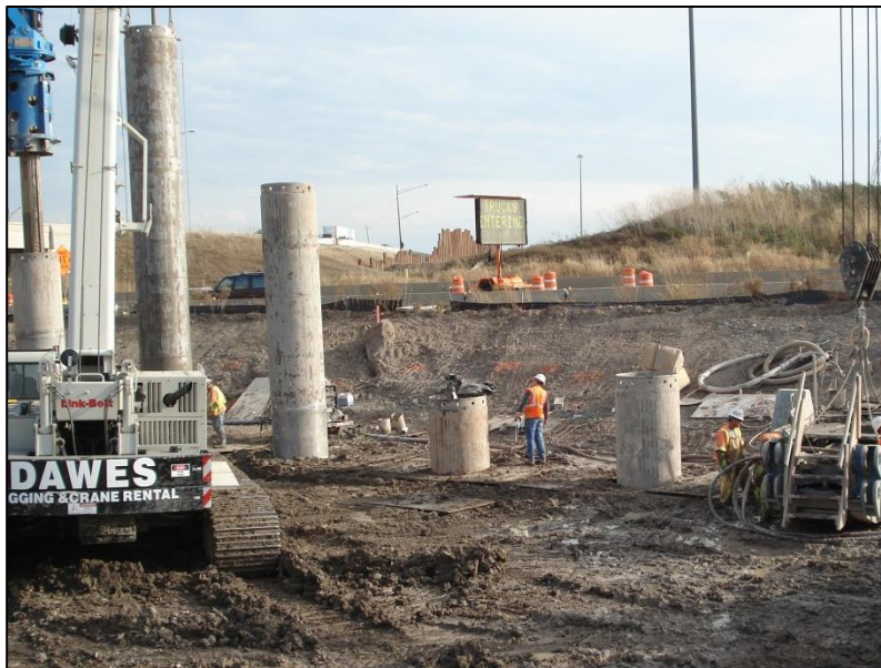
Figure 4.4.4-14: Secant Wall Construction.
