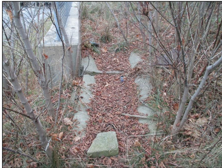
Figure 4.4.5-1: Concrete Flume at End of Wall. Condition State 2 (Fair) – No Erosion Evident, with wide crack.
