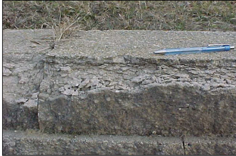
Figure 4.4.2-18: Freeze-Thaw Damage at a Corner.
