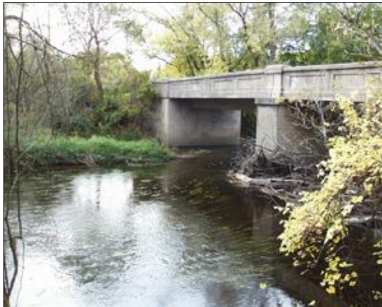
Figure 2.8.2.2-2: Aggradation in Front of Abutment and Debris Buildup in Front of Pier.
