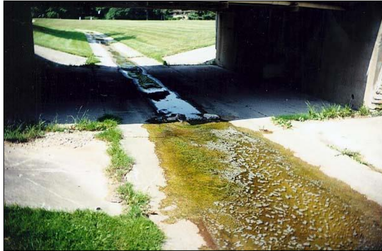
Figure 2.8.2.1-3: Concrete Channel Lining Protection.
