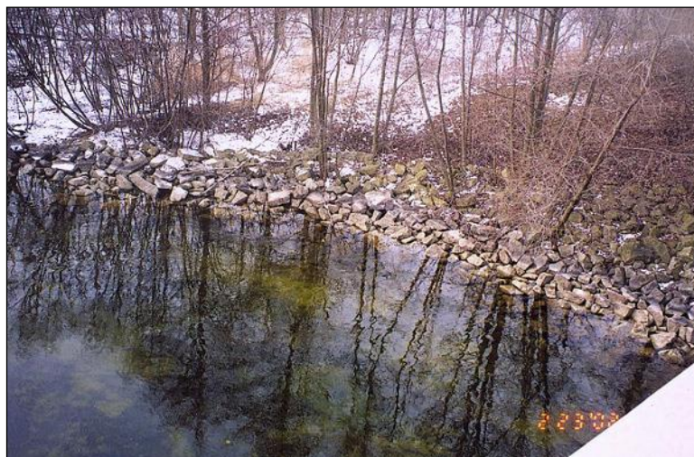
Figure 2.8.2.1-2: Riprap Channel Protection.
