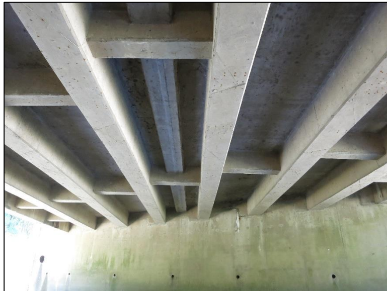
Figure 2.7.1-14: Assessment 9168 – Concrete Diaphragm.
