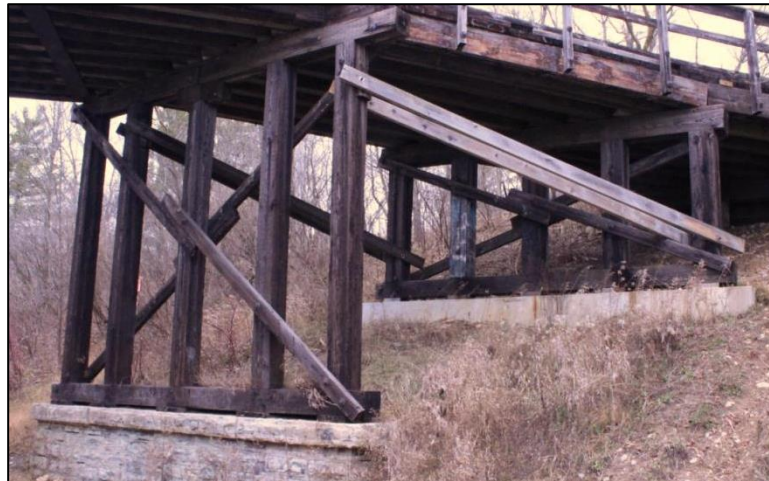
Figure 2.7.1-17: Assessment 9250 – Crash Walls/Web Walls/Cross Bracing or Struts.
