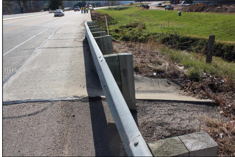
Figure 2.7.1-1: Assessment 9001 – Approach Drainage. Note concrete flume.
