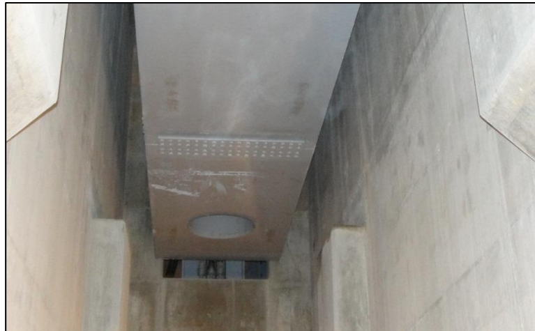
Figure 2.7.1-5: Assessment 9020 – Movable Bridge Counterweight.
