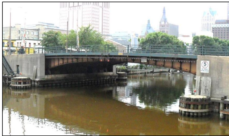
Figure 2.7.1-18: Assessment 9290 – Dolphin or Fender System.
