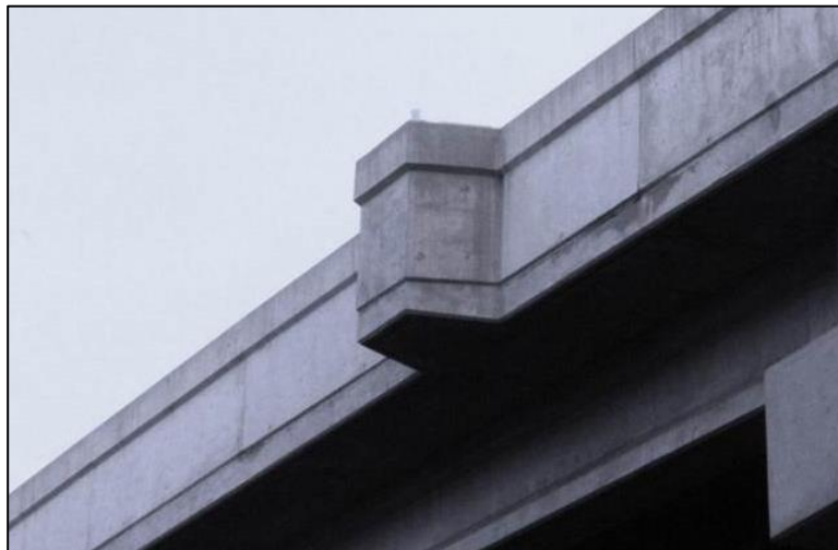
Figure 2.7.1-24: Assessment 9336 – Luminaire Bases.
