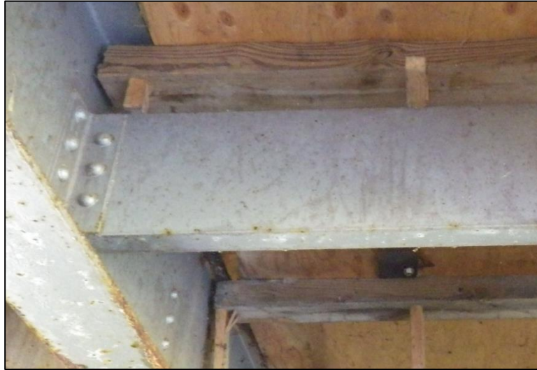
Figure 2.7.1-13: Assessment 9167 – Steel Diaphragm.
