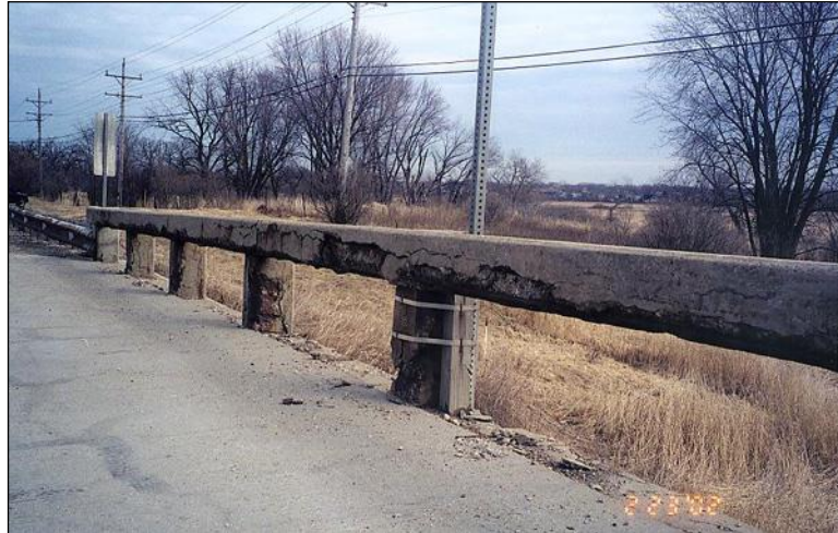
Figure 2.6.8.2-5 Concrete Bridge Railing - Condition State 4
