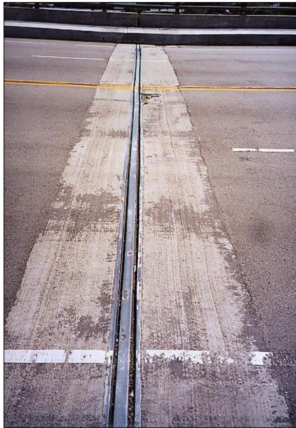
Figure 2.6.5.4-1 Modular Expansion Joint – Condition State 1
