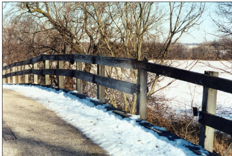
Figure 2.6.8.3-3 Missing Timber Bridge Rail Beam – Condition State 3
