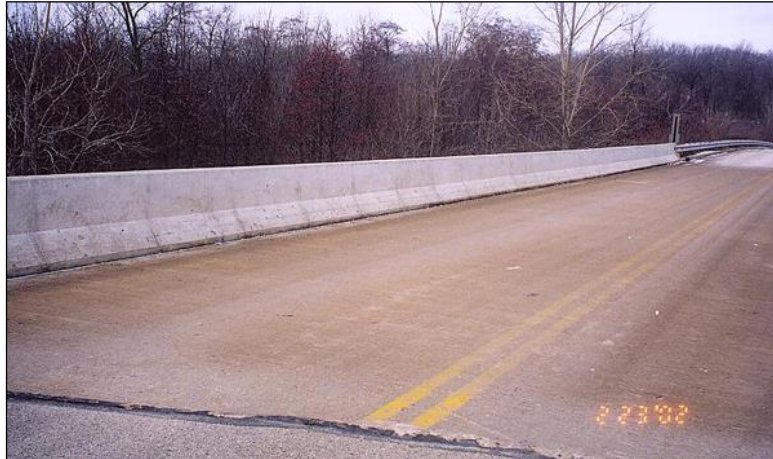
Figure 2.6.8.2-1 Concrete Bridge Railing - Condition State 1
