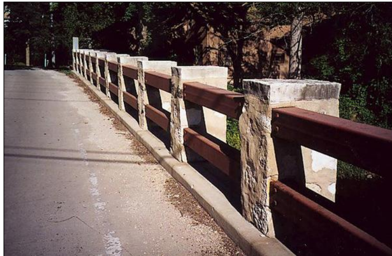
Figure 2.6.8.1-1 Metal Railing with Masonry Posts – Condition State 1
