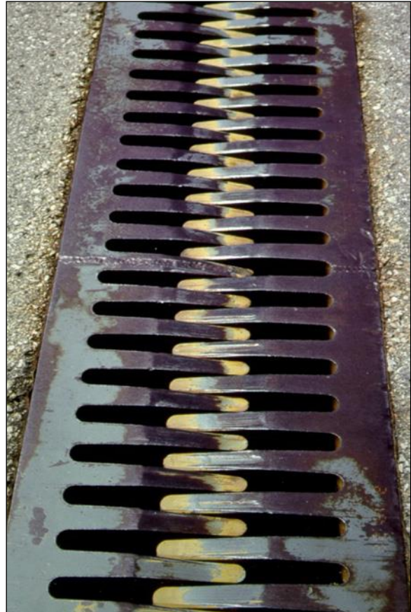
Figure 2.6.4.6-2: Finger Plate Expansion Joint – Condition State 1.
