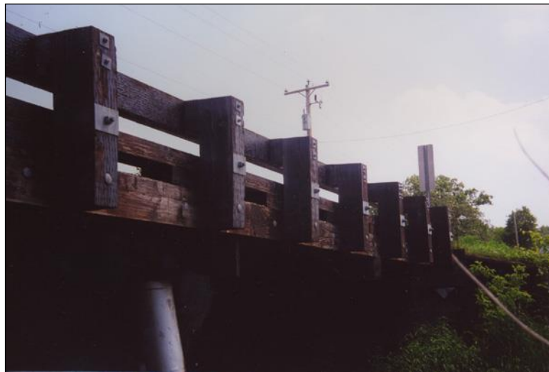
Figure 2.6.8.3-1 Timber Bridge Railing - Condition State 1
