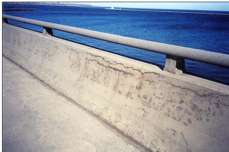
Figure 2.6.8.2-6 Concrete Railing with Decorative Rail Assessment – Condition State 3
