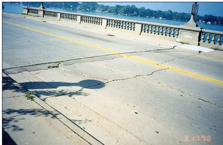
Figure 2.6.2.2-1 Concrete Approach with Wide Cracks – Condition State 3
