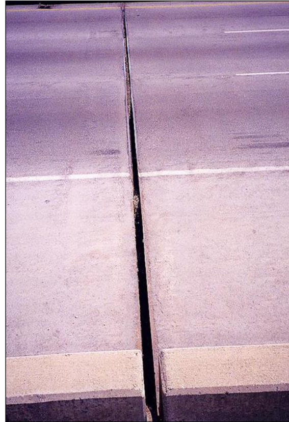
Figure 2.6.4.3-2: Compression Seal Pushed Down Into the Joint Opening - Condition State 3.
