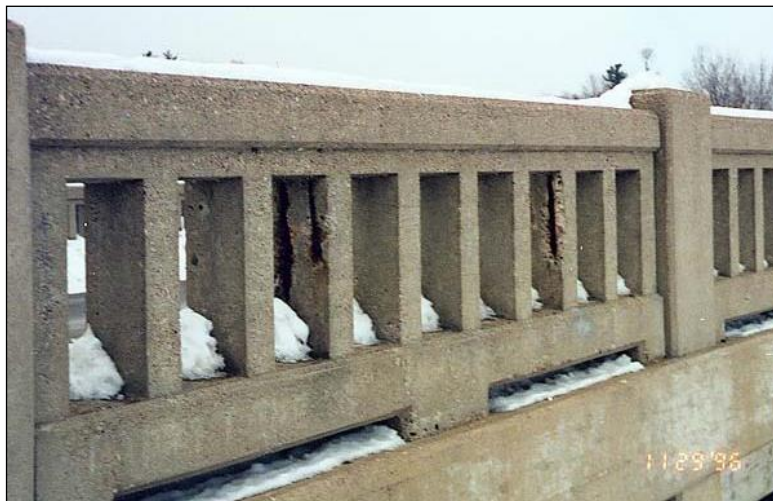
Figure 2.6.8.2-2 Concrete Bridge Rail – Most in Condition State 1 - Two Areas Condition State 3.
