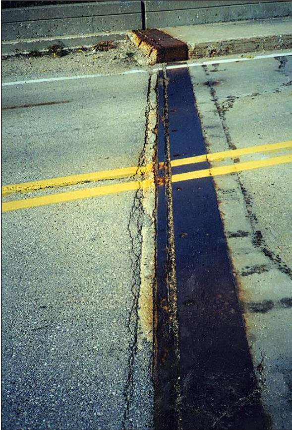
Figure 2.6.4.6-1: Sliding Plate Expansion Joint (Note Transverse Deck Crack on Left Side Suggesting a Failing Anchorage System) – Condition State 2.
