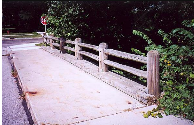
Figure 2.6.8.3-2 Timber Bridge Railing – Condition State 2
