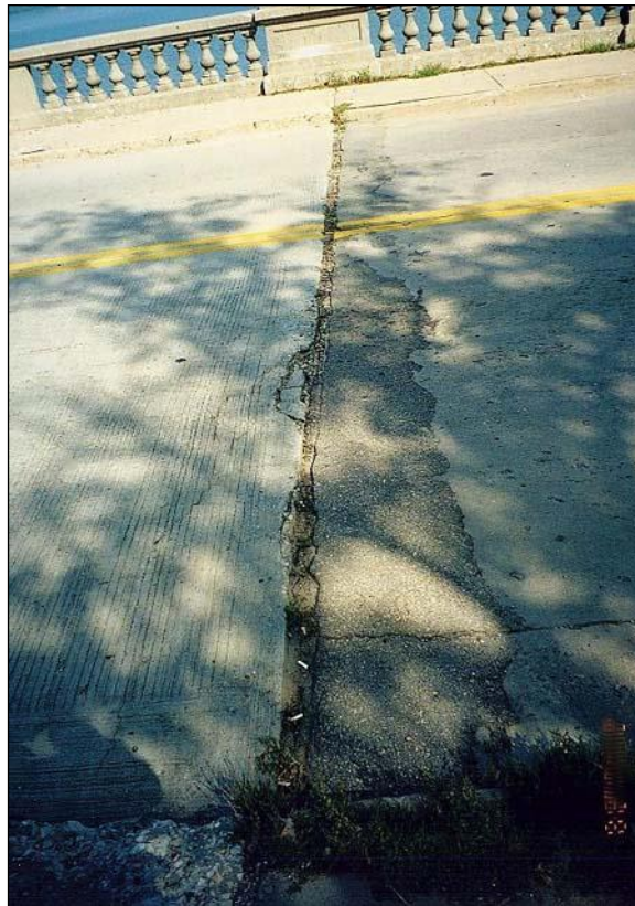
Figure 2.6.5.2-1 Poured Joint Seal – Condition State 3
