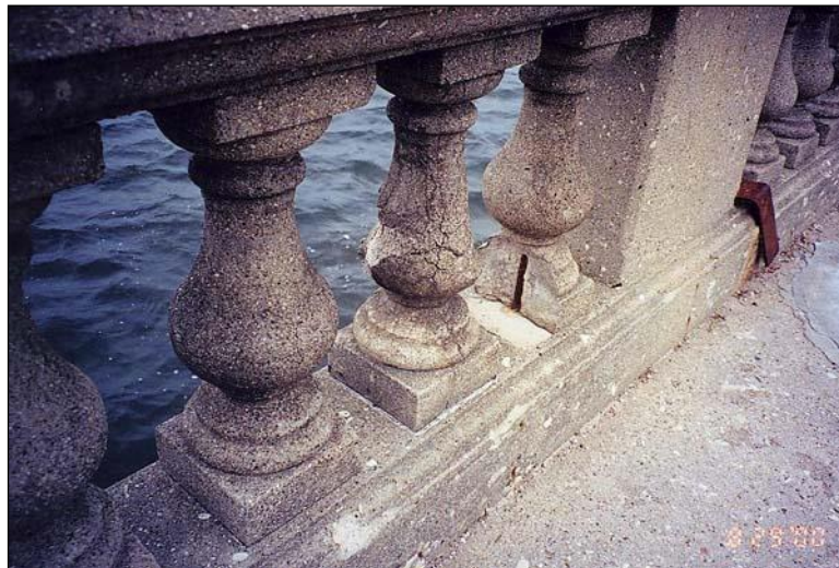
Figure 2.6.8.2-4 Ornamental Concrete Bridge Rail – Condition State 3
