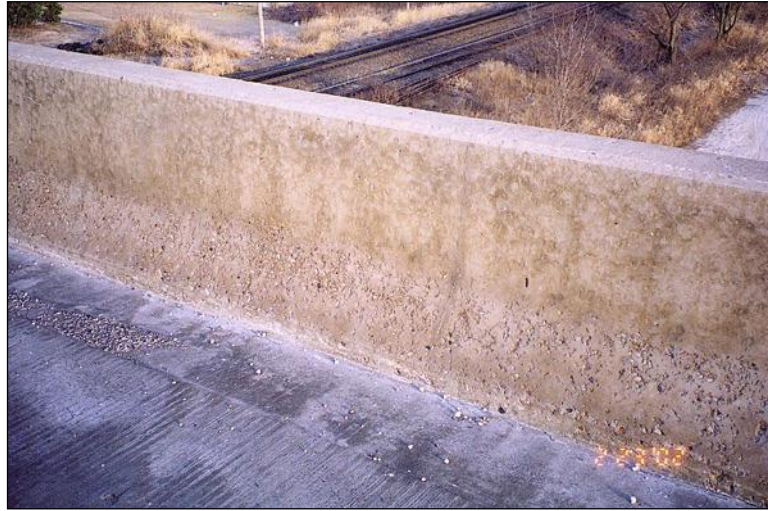
Figure 2.6.8.2-3 Scaling on the Lower Half of a Concrete Bridge Rail - Condition State 2
