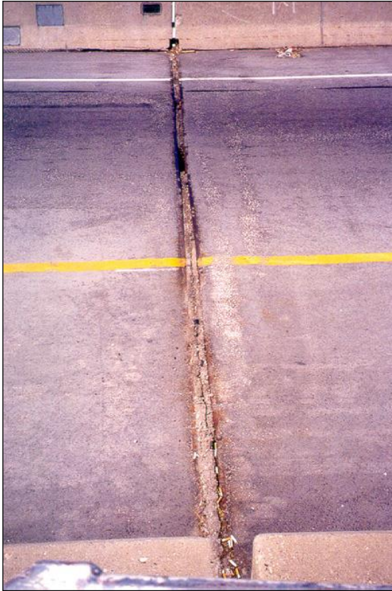
Figure 2.6.4.3-1: Compression Joint Seal Impacted with Debris and Pushed Down Into the Joint Opening (Far Lane)– Condition State 4.
