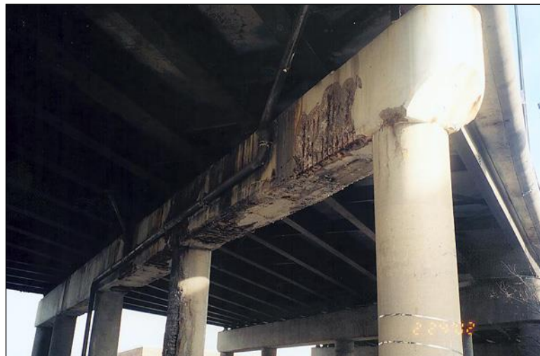
Figure 2.5.3.6-5: Pier Cap with Widespread Spalling – Condition State 3
