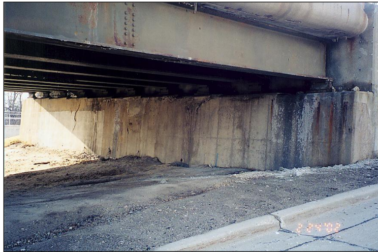
Figure 2.5.3.3-1: Reinforced Concrete Semi Retaining Abutment
