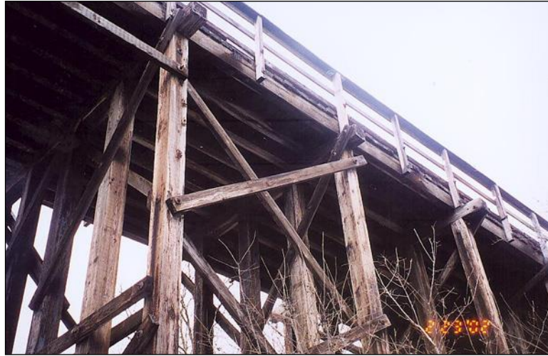
Figure 2.5.5.1-1: Timber Pier Columns
