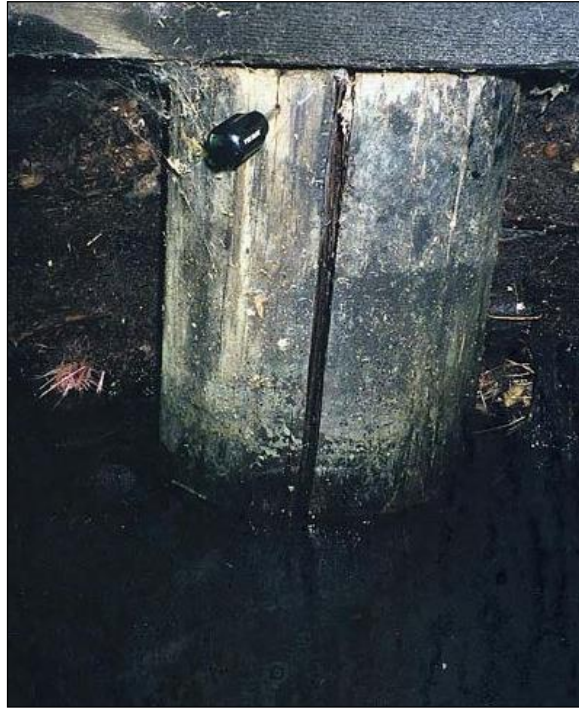
Figure 2.5.5.5-3: Split Timber Pile - Condition State 3
