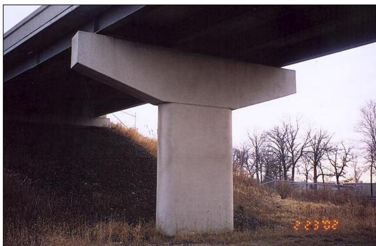
Figure 2.5.3.1-2: Hammerhead Pier Reinforced Concrete Column – Condition State 1 (The cap of the hammerhead pier is reported under Element 234).
