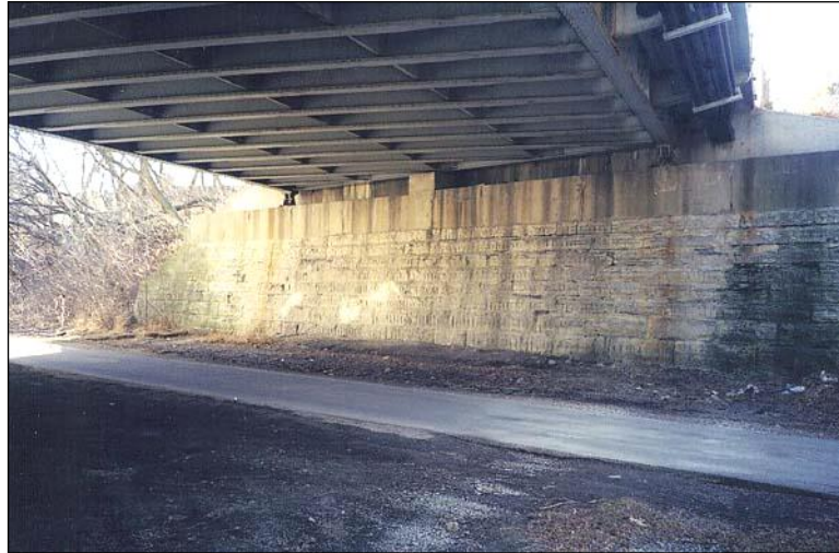
Figure 2.5.6.2-1: Masonry Abutment
