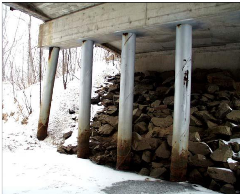
Figure 2.5.2.4-1: Heavy Corrosion at the Ground Line on Painted Steel Piles - Condition State 4
