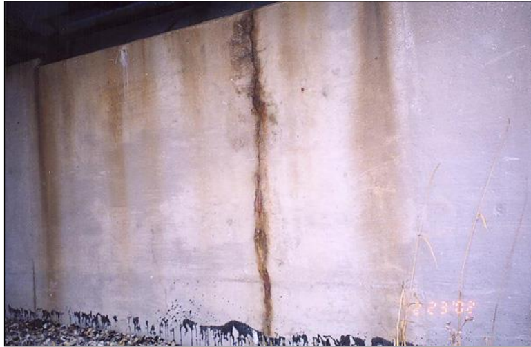
Figure 2.5.3.3-4: Vertical Crack in an Abutment – Condition State 2
