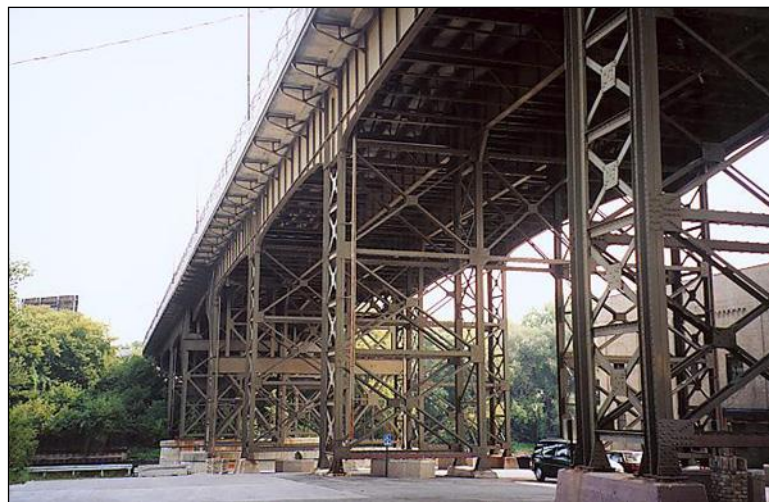
Figure 2.5.2.2-1: Steel Towers/Trestles – Condition State 1
