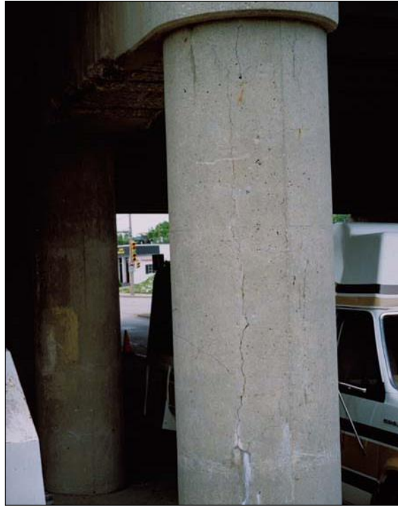
Figure 2.5.3.1-3: Concrete Column with Vertical Crack - Condition State 2
