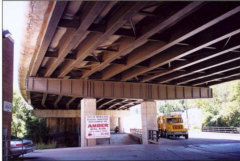
Figure 2.5.2.6-1: NSTM Riveted Steel Box Girder Pier Cap. Note that the superstructure girders bear on the pier cap's top flange by way of bearing devices
