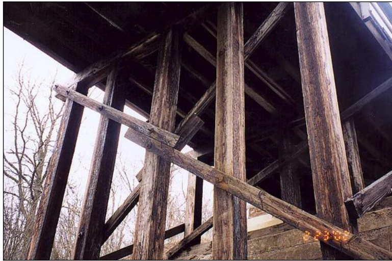
Figure 2.5.5.1-2: Timber Columns, Cap, and Cross-Bracing – Condition State 1
