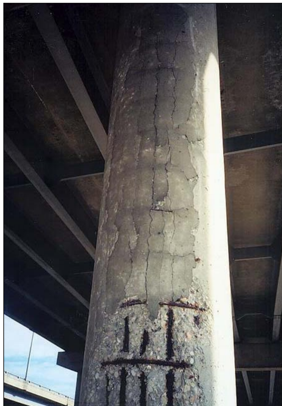
Figure 2.5.3.1-6: Delaminated and Spalled Column - Condition State 3
