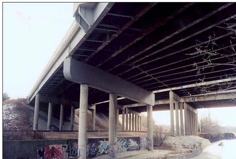
Figure 2.5.2.5-1: Steel Box Pier Cap
