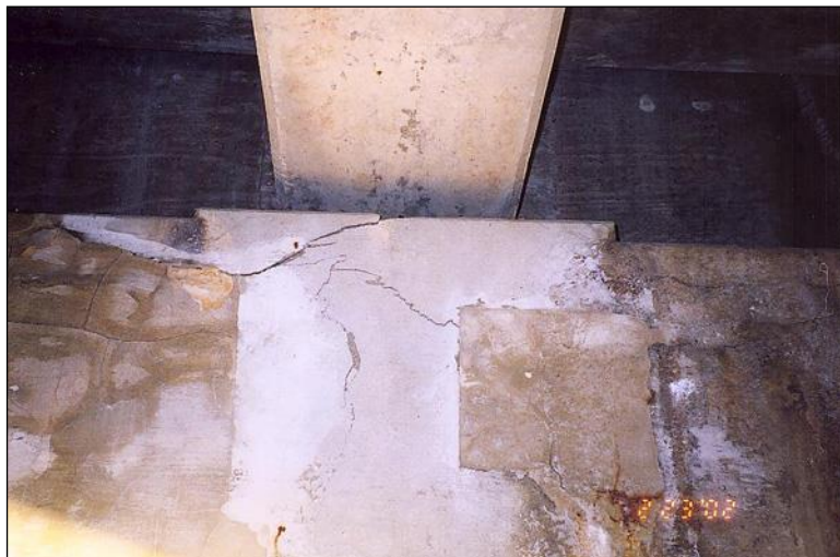
Figure 2.5.3.3-5: Abutment Delaminations Under the Bearing – Condition State 2
