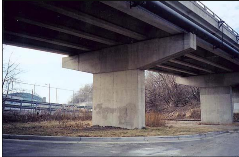
Figure 2.5.1.2-4: Hammerhead Pier
