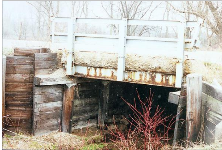
Figure 2.5.4.3-1: Timber Abutment and Wingwalls
