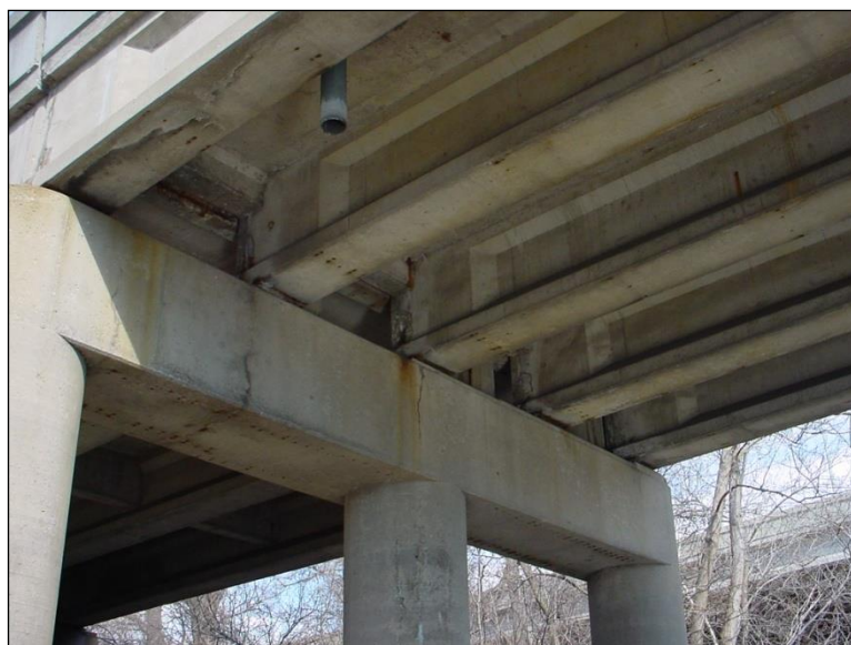
Figure 2.5.3.6-1: Reinforced Concrete Pier Cap
