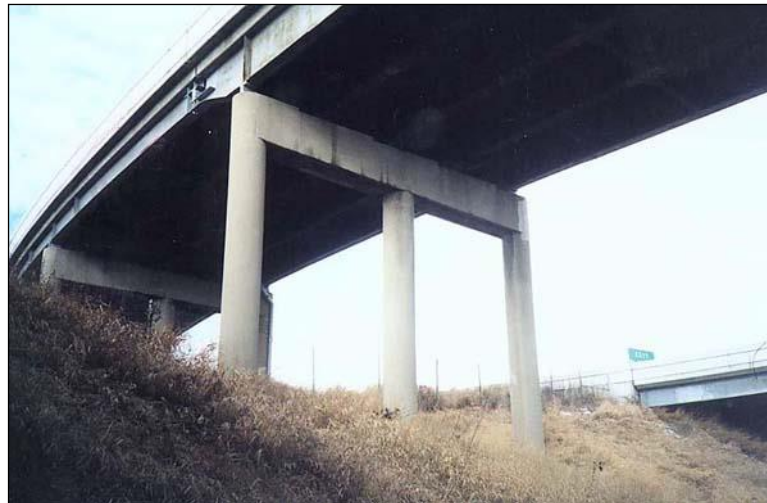
Figure 2.5.1.2-3: Reinforced Concrete Columns and Pier Cap
