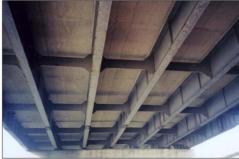
Figure 2.4.4-2: Steel Multi-Girder Bridge.
