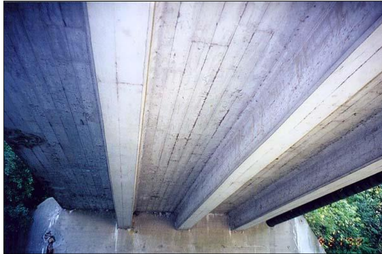
Figure 2.4.2.2-2: Reinforced Concrete Tee Beams – Condition State 1.
