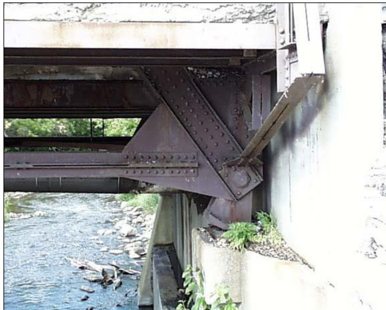
Figure 2.4.8.2-12: Rocker Bearing – Movement Condition State 3.
