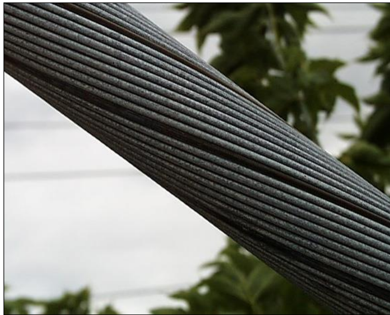
Figure 2.4.4.2-2: Galvanized Steel Cable – Condition State 1.
