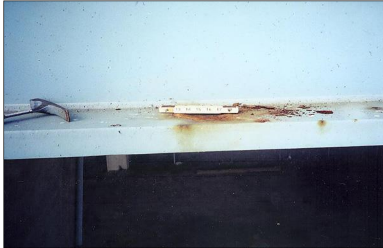
Figure 2.4.4.1-29: Pit Caused by Section Loss on Girder Bottom Flange – Corrosion Condition State 3.
