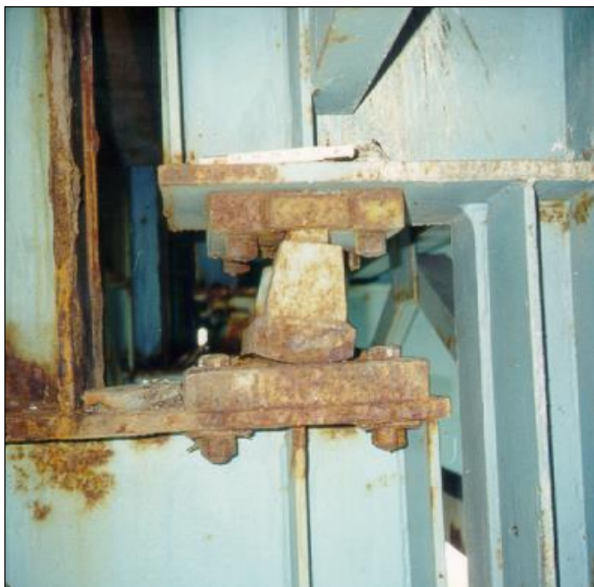
Figure 2.4.8.2-9: Rocker Bearing – Condition State 2.
