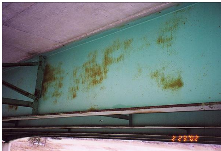
Figure 2.4.4.1-23: Girder – Corrosion Condition State 2.
