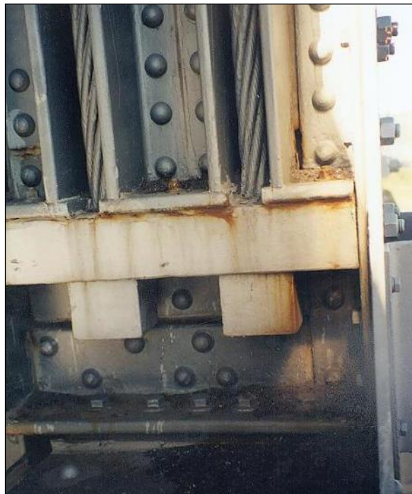
Figure 2.4.4.2-3: Cable Anchorage for a Tied Arch Bridge – Condition State 1.
