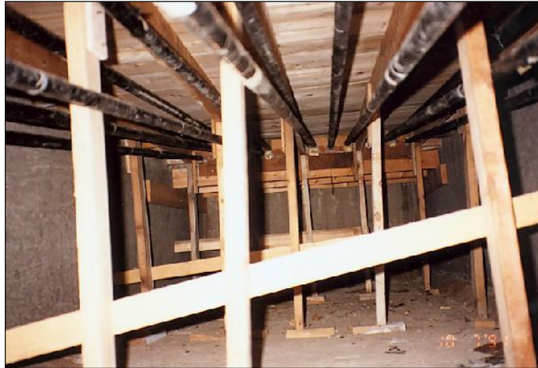
Figure 2.4.4.3-1: Exposed Post Tensioning Rods Inside of a Concrete Box Girder - Condition State 1.
