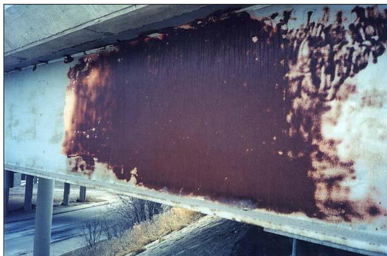
Figure 2.4.4.1-24: Steel Girder – Corrosion Condition State 2.
