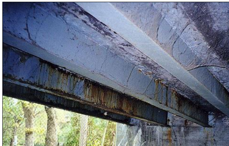
Figure 2.4.4-1: Rolled Steel Multi-beam Bridge.
