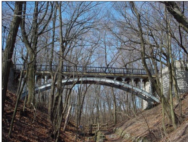
Figure 2.4.4-7: Steel Deck Arch Bridge.
