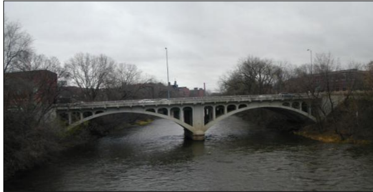
Figure 2.4.3-5: Open Spandrel Reinforced Concrete Arch.
