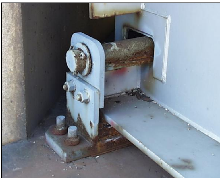
Figure 2.4.8.2-10: Hold-Down (Restraining) Bearing - Corrosion Condition State 2.
