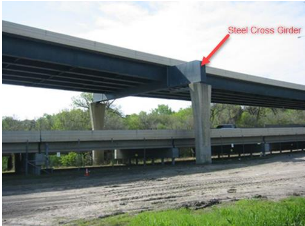
Figure 2.4.4.1-1: Steel Cross Girder – Closed Web/Box Girder
