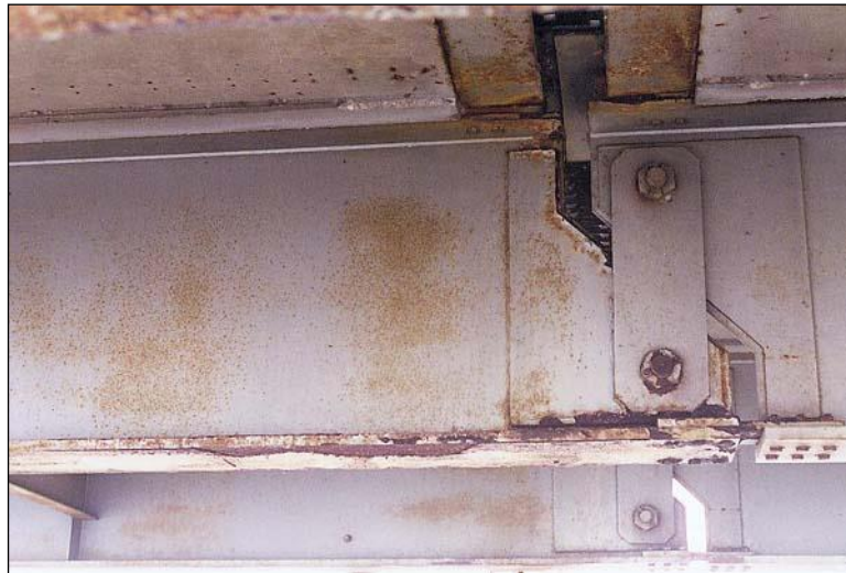
Figure 2.4.4.7-5: Girder, Pin, and Hanger – Corrosion Condition State 2.
