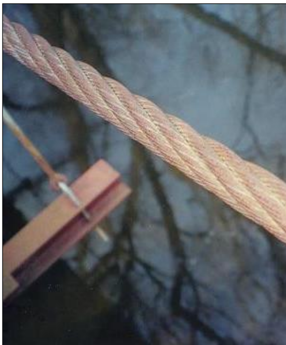
Figure 2.4.4.2-3: Cable Anchorage for a Tied Arch Bridge – Condition State 1.
