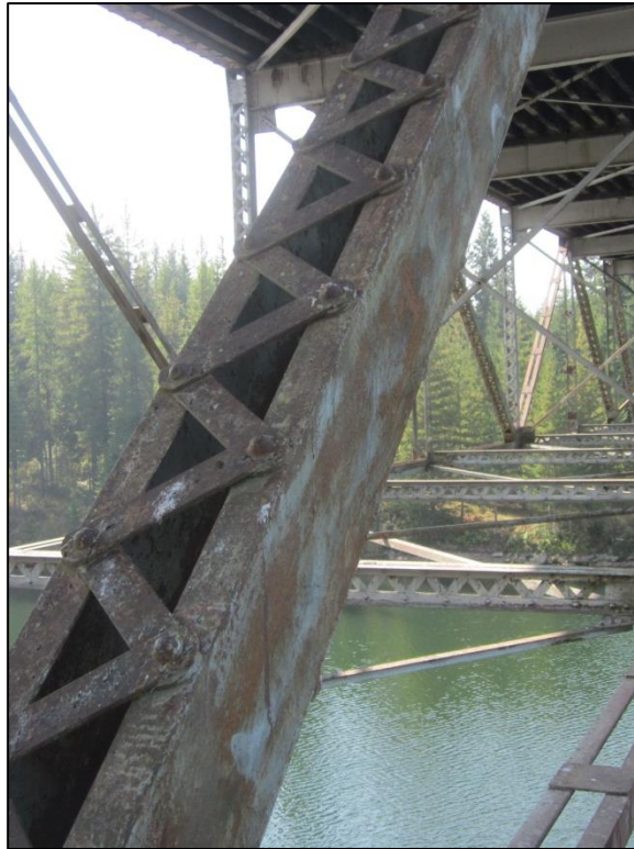
Figure 2.4.4.4-3: Diagonal Truss Member Exhibiting Rust with No Loss of Section – Corrosion Condition State 2.
