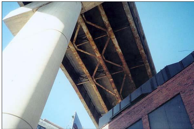
Figure 2.4.4.1-30: Steel Girders – Corrosion Condition State 3.
