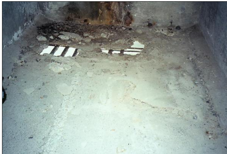
Figure 2.4.2.2-7: Reinforced Concrete Box Girder Bottom Flange Through Thickness Section Loss - Condition State 4.
