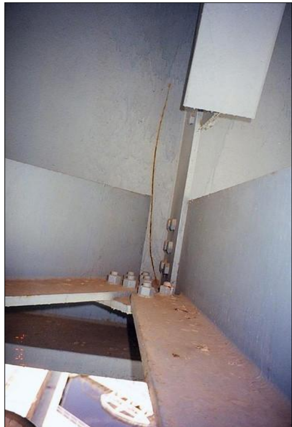
Figure 2.4.4.1-6: Same Crack as shown in Figure 4.75, Inside Face of Girder at Lower Lateral Shelf Plate - Condition State 4.
