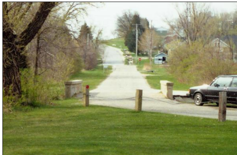
Figure 2.4.3-3: Reinforced Concrete Through Girder Bridge.
