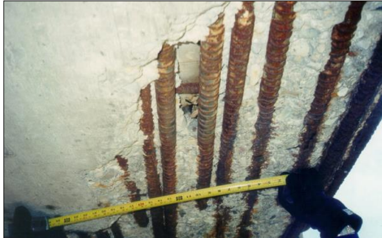
Figure 2.4.2.2-4: Corner of Reinforced Concrete Box Girder – Condition State 3.
