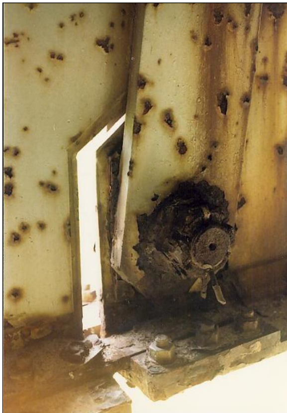
Figure 2.4.4.7-6: Pin and Hanger – Corrosion Condition State 4.
