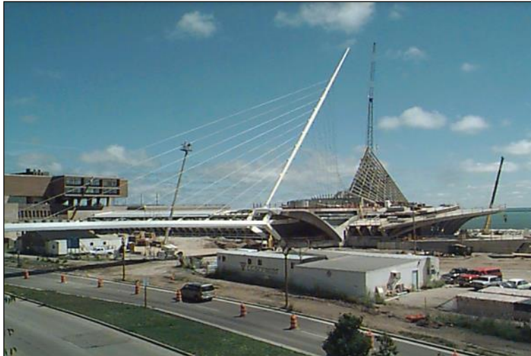
Figure 2.4.4-10: Cable Stayed Pedestrian Bridge.
