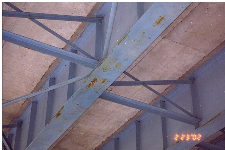
Figure 2.4.4.1-22: Steel Girders – Corrosion Condition State 2.
