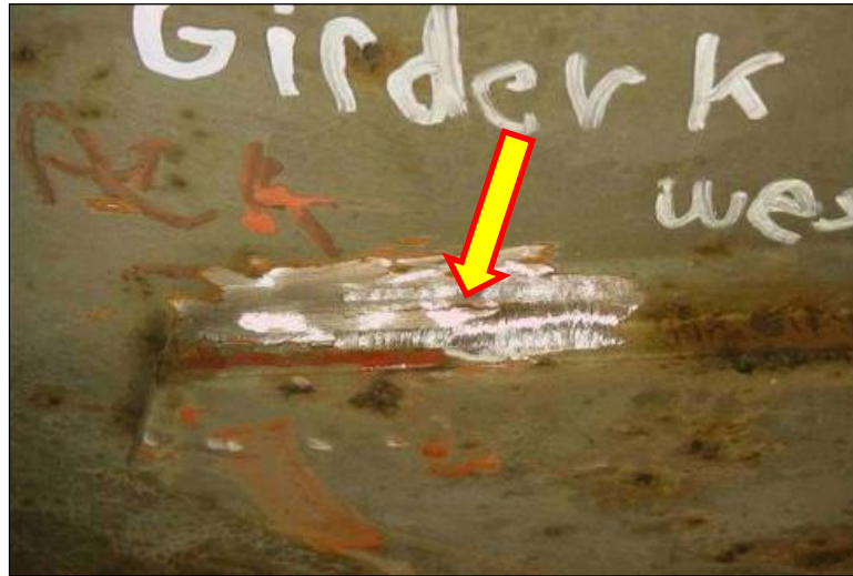
Figure 2.4.4.1-7: Fatigue Crack at a Welded Cover Plate End (Rust Line within the Ground Area).
