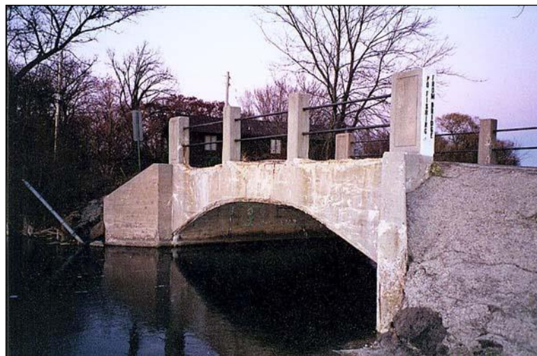
Figure 2.4.2.3-1: Reinforced Concrete Arch Bridge.
