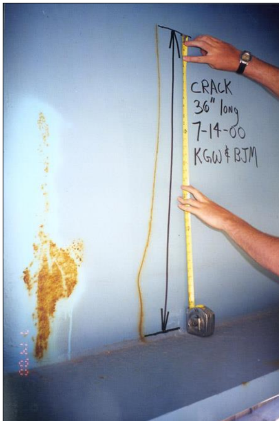
Figure 2.4.4.1-5: Brittle Crack 3 Feet Long in a Girder Web 10 Feet Deep, Opposite of Lower Lateral Shelf Plate - Condition State 4.
