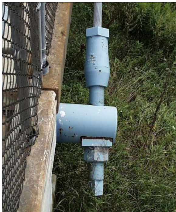
Figure 2.4.4.2-3: Cable Anchorage for a Tied Arch Bridge – Condition State 1.
