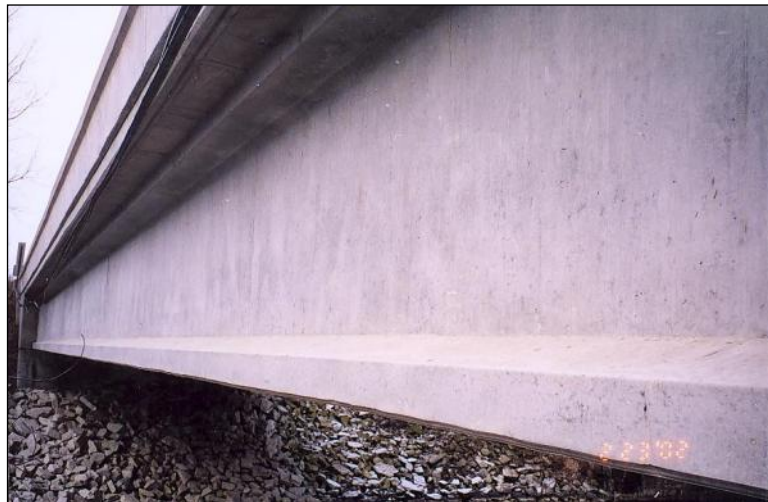
Figure 2.4.3.1-2: Prestressed I-Beam – Condition State 1.
