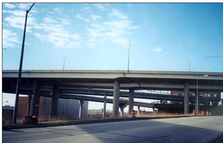
Figure 2.4.3-3: Conventionally Reinforced Box Girder Bridge.
