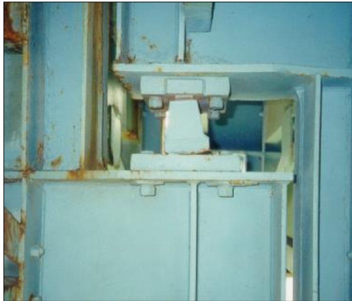
Figure 2.4.8.2-6: Rocker Bearing – Condition State 1.
