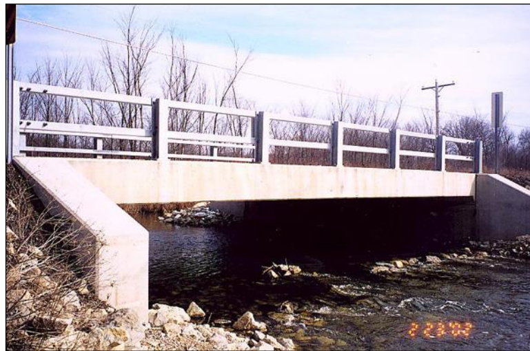
Figure 2.4.2-1: Single Span Flat Slab Bridge.
