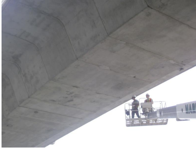
Figure 2.4.3-4: Segmental Box Girder Bridge.
