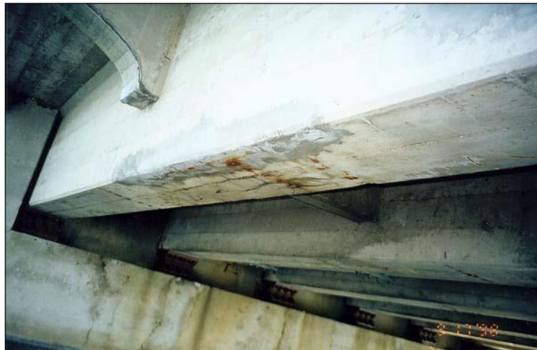
Figure 2.4.2.2-3: Reinforced Concrete Tee Beam – Condition State 2.
