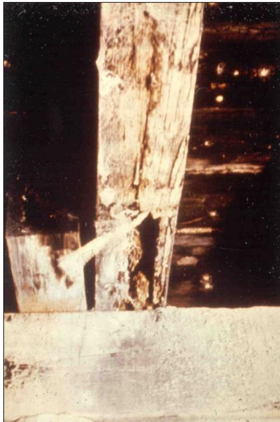
Figure 2.4.5.1-4: Timber Beam – Decay/Section Loss Condition State 4.
