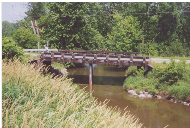
Figure 2.4.5-1: Solid Sawn Multi-Beam Bridge.
