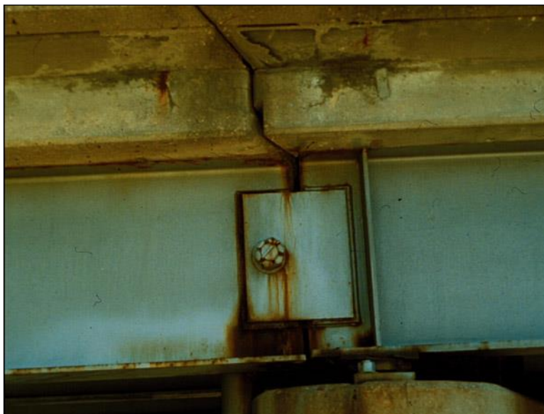
Figure 2.4.4.7-2: Single Pin and Plate Assembly.
