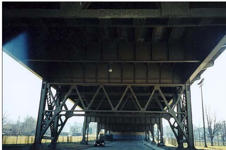
Figure 2.4.4-3: Two Girder System Bridge.
