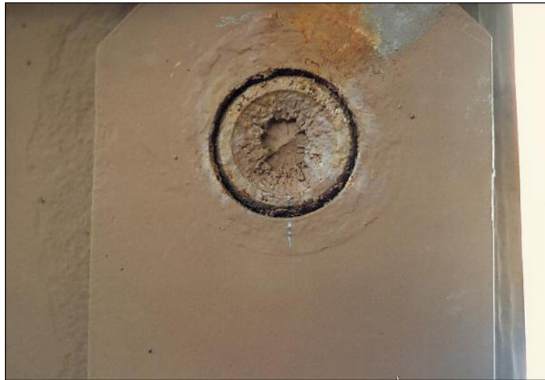
Figure 2.4.4.7-3: Pin Shear Failure.
