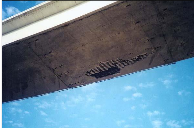
Figure 2.4.2.2-6: Reinforced Concrete Box Girder Bottom Flange Through Thickness Section Loss - Condition State 4.
