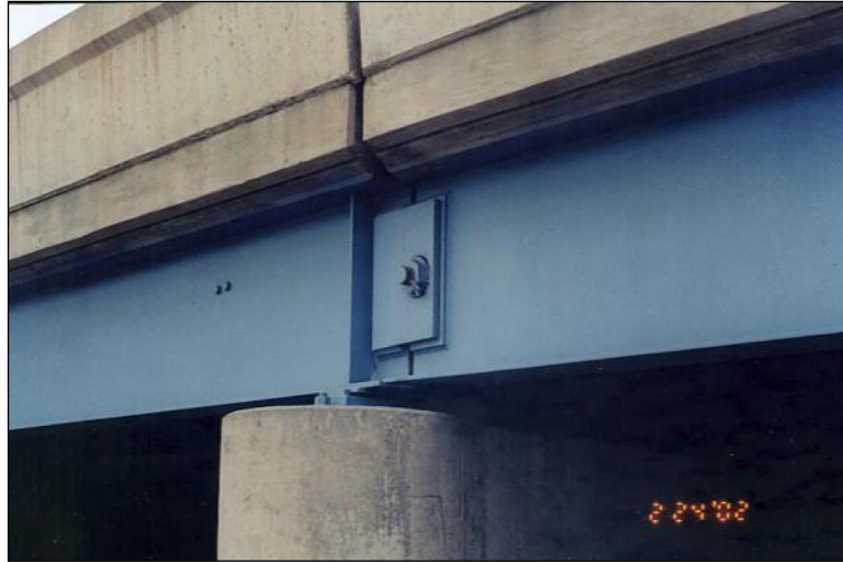
Figure 2.4.4.7-4: Steel Girders, Pin and Plate – Condition State 1.
