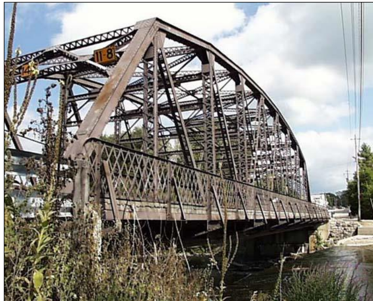
Figure 2.4.4-6: Steel Truss Bridge.
