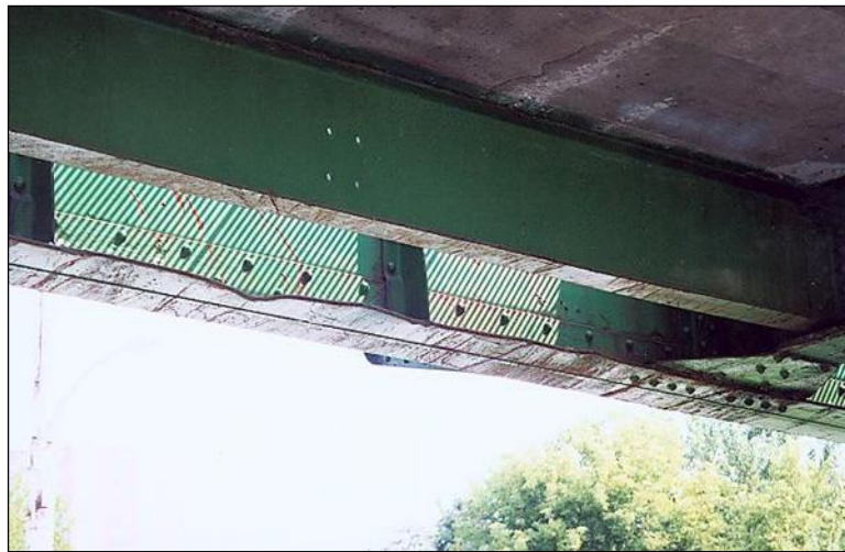
Figure 2.4.4.1-28: Impact Damage to Bottom Flange of a Two-Girder Bridge – Distortion Condition State 2.
