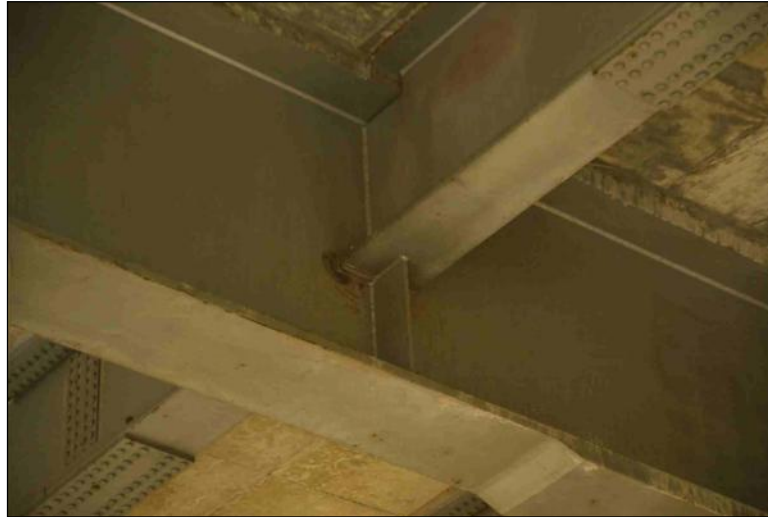
Figure 2.4.4.1-9: Welded Girder to Cross Girder Connection Detail.
