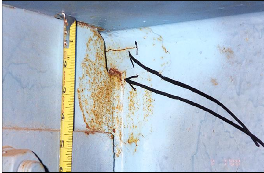
Figure 2.4.4.1-15: Double Fatigue Cracks in Girder Web, Top of Connection Plate – Condition State 3.
