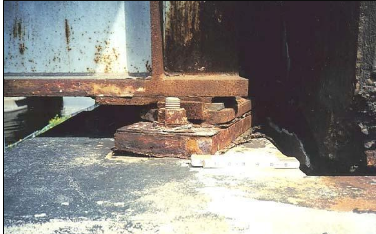
Figure 2.4.8.2-13: Masonry Plate Walking Out Due to Failed Anchor Bolt – Connection Condition State 3.
