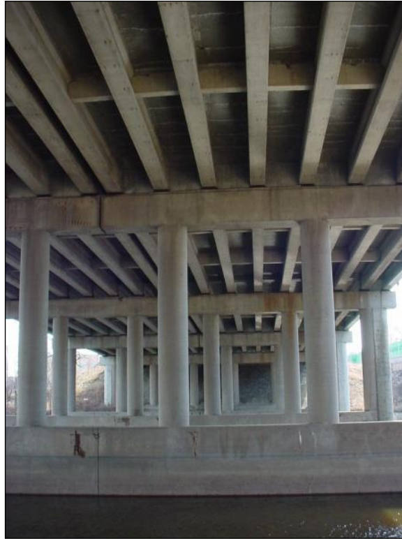
Figure 2.4.3-1: Prestressed I-beams.
