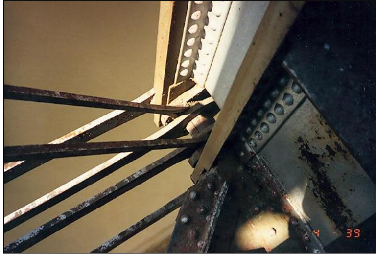
Figure 2.4.4.4-2: Multiple Eyebars Connected with a Pin.
