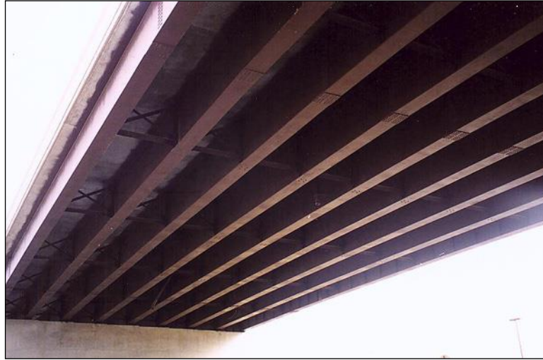
Figure 2.4.4.1-2: Fabricated Girders and Rolled Cross-Frame Members.
