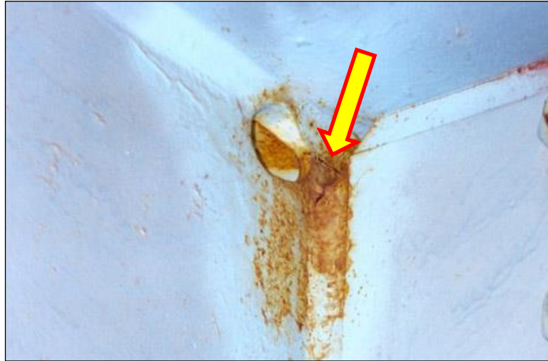
Figure 2.4.4.1-11: Fatigue Crack Through Girder Web Arrested with a Drilled Hole, Top of Connection Plate - Condition State 2.
