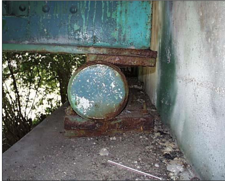
Figure 2.4.8.2-11: Critically Misaligned Roller Bearing – Alignment Condition State 3.
