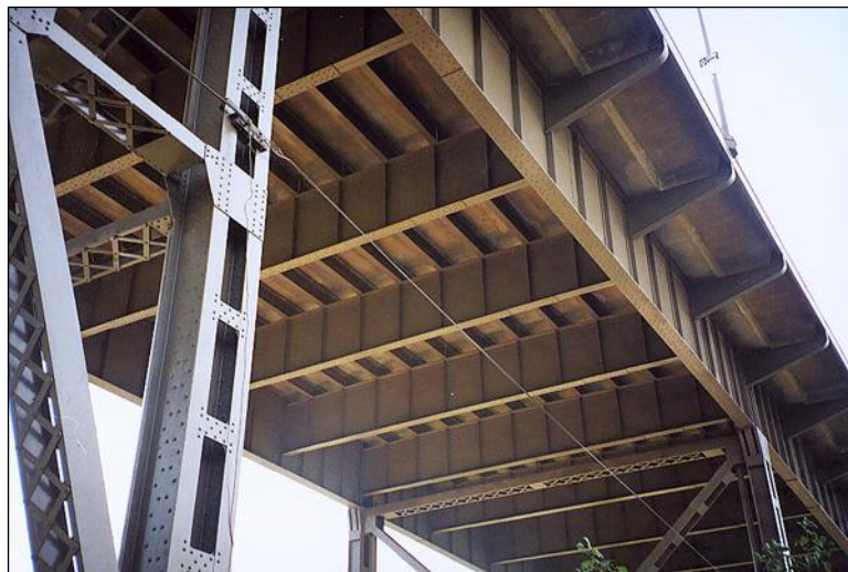
Figure 2.4.4.8-1: NSTM Two-Girder Bridge.
