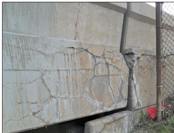
Figure 2.3.2.1-4: Typical Reinforced Concrete Slab Distress.
