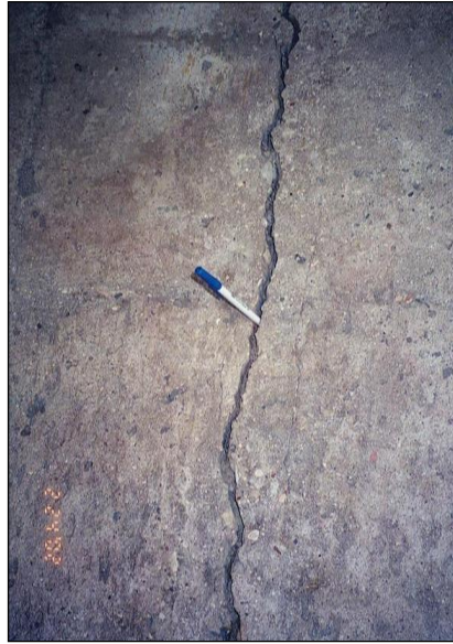
Figure 2.1.4.1-3: Wide Vertical Crack in an Abutment.
