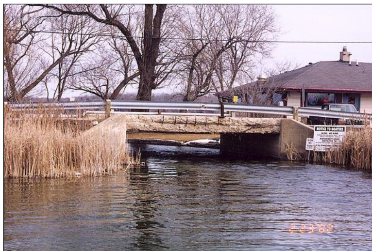
Figure 2.1.5.1-1: Heavily Deteriorated Single Span Concrete Slab.
