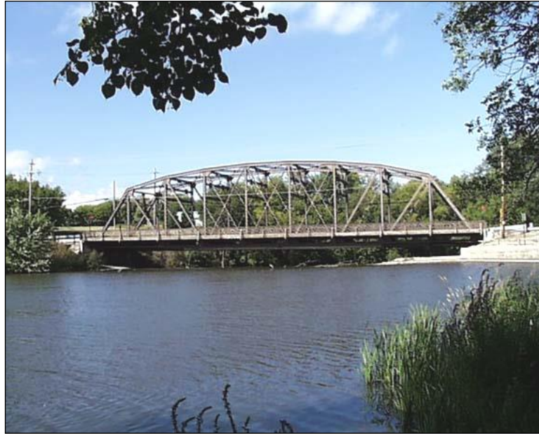
Figure 2.1.5.3-1: Parker Truss Bridge.
