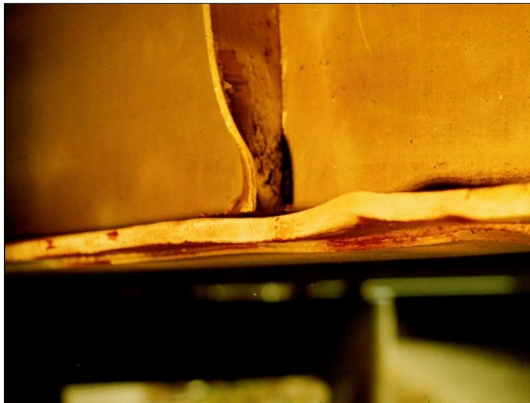
Figure 2.1.4.2-8: Girder Bottom Flange Impact Damage.
