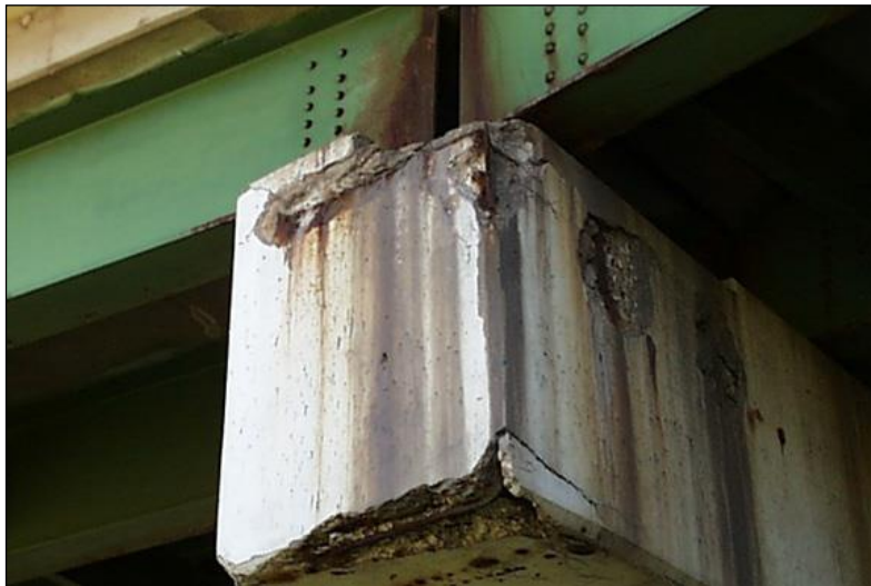
Figure 2.1.4.1-6: Spalled Concrete on Pier Cap.
