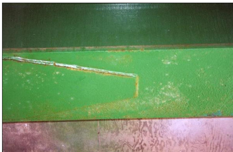
Figure 2.1.4.2-2: Transverse Weld at a Cover Plate End.
