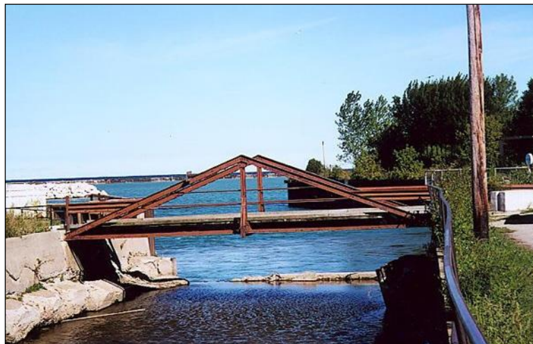
Figure 2.1.5.3-2: King Post Truss Bridge.
