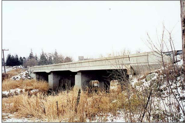
Figure 2.1.5.1-2: Three-Span Concrete Slab with Haunches.
