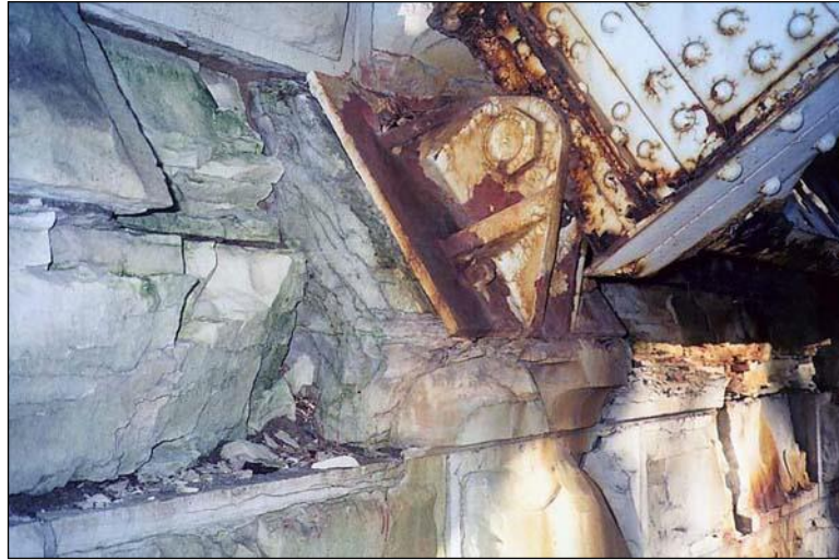
Figure 2.1.4.4-1: Masonry Deterioration/Spalls at an Arch Bearing.
