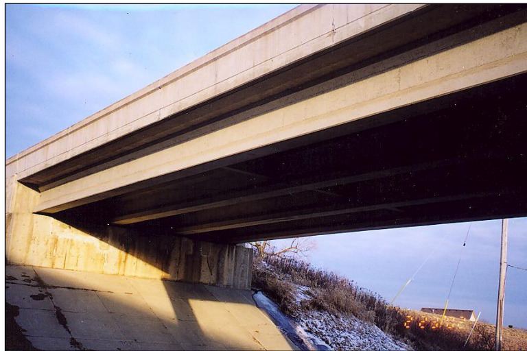
Figure 2.1.5.2-2: Prestressed Concrete Multiple Girder Bridge.
