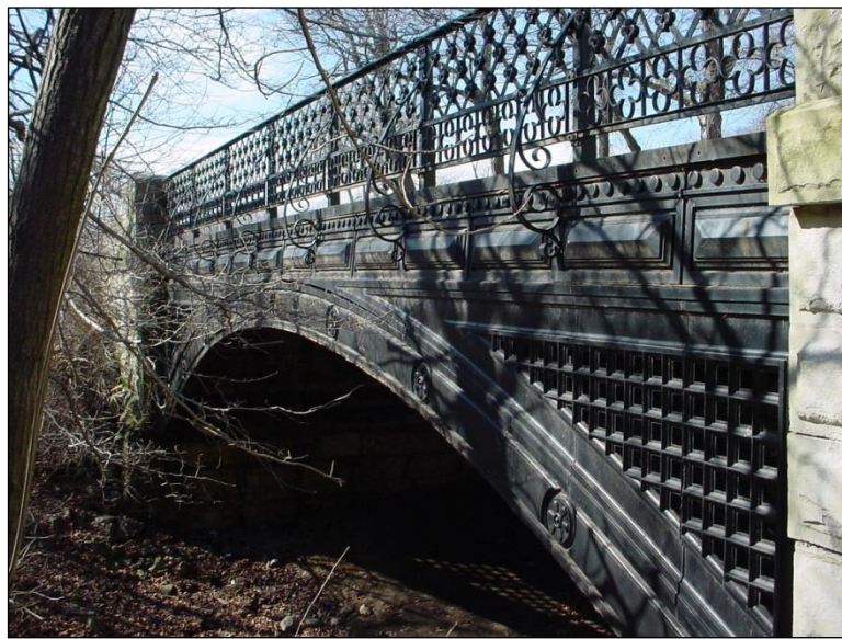
Figure 2.1.4.4-3: Cast Iron Arch.
