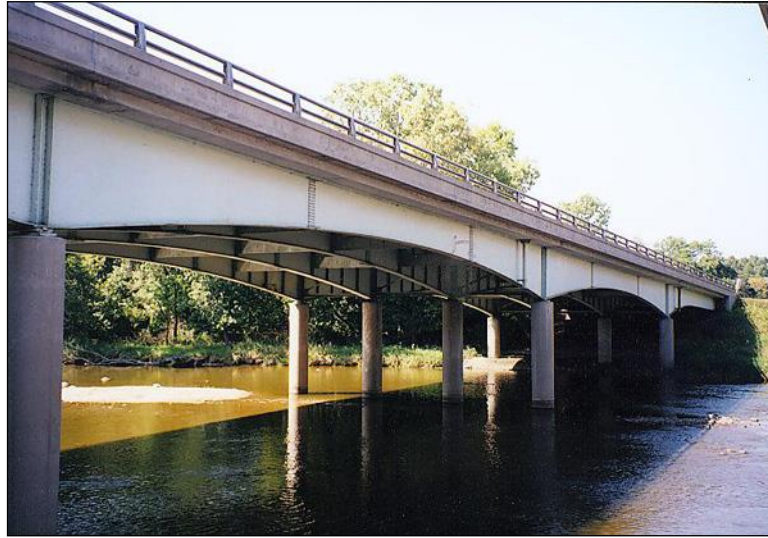
Figure 2.1.2.3-1: Continuous Spans – Steel Girders.
