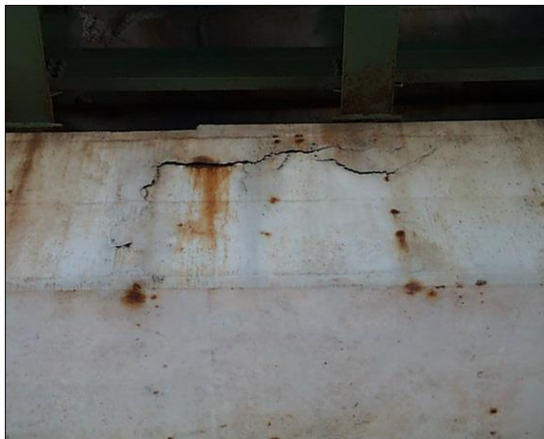
Figure 2.1.4.1-5: Delaminations on Concrete Pier.
