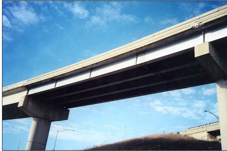
Figure 2.1.5.2-1: Steel Multiple Girder Bridge.
