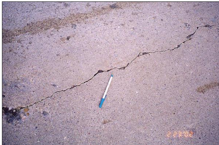
Figure 2.1.4.1-2: Moderate Longitudinal Crack in a Concrete Deck.
