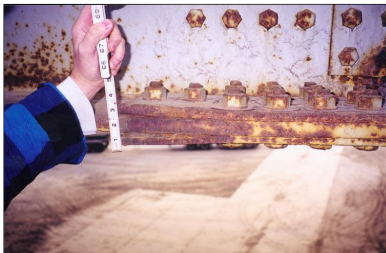
Figure 2.1.4.2-7: Pack Rust Prying Apart Flange Splice Plates.
