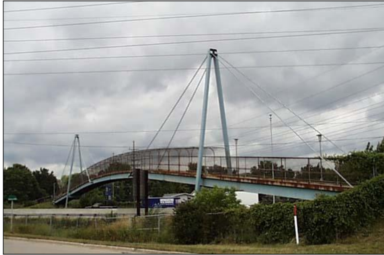
Figure 2.1.5.6-1: Cable-Stayed Pedestrian Bridge.
