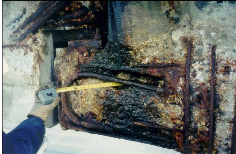
Figure 2.1.4.1-7: Reinforcing Steel Corrosion.
