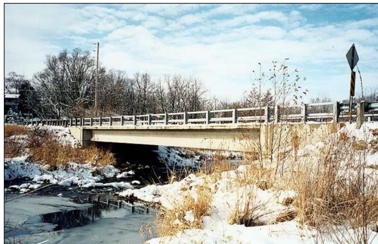
Figure 2.1.2.2-1: Simply Supported Span – Prestressed Concrete Girders.
