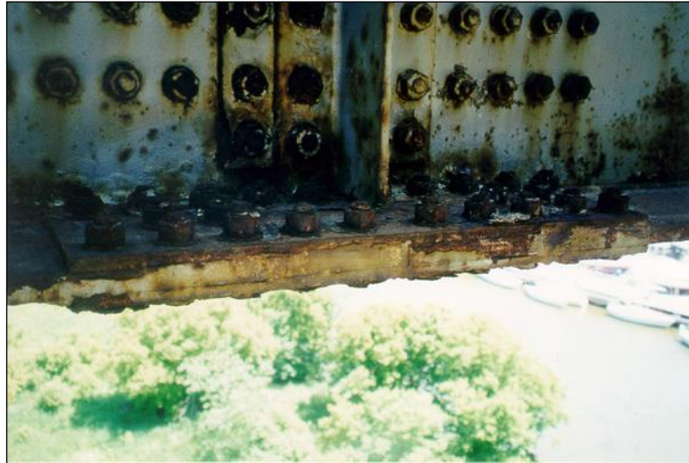
Figure 2.1.4.2-5: Steel Corrosion at Girder Splice.
