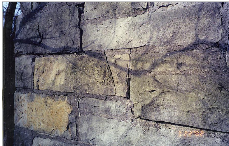
Figure 2.1.4.4-2: Split Masonry Unit with Failing Mortar Joints.
