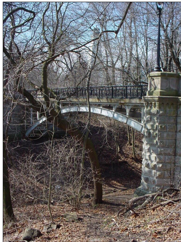
Figure 2.1.5.4-2: Steel Open Spandrel Arch.
