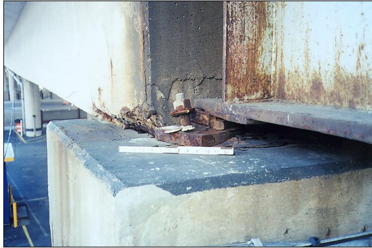
Figure 1.4.3.3-2: Failed Bearing at Pier.
