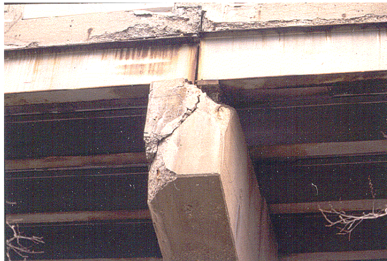
Figure 1.4.3.3-3: Damage Resulting From Failed Joint.
