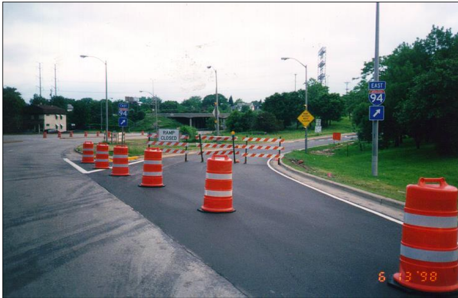
Figure 1.4.8.1-1: Barrels Channel Traffic Away From Work Zone.
