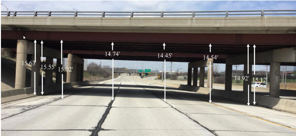
Figure 1.3.19.1-1: Vertical Clearance Photo
