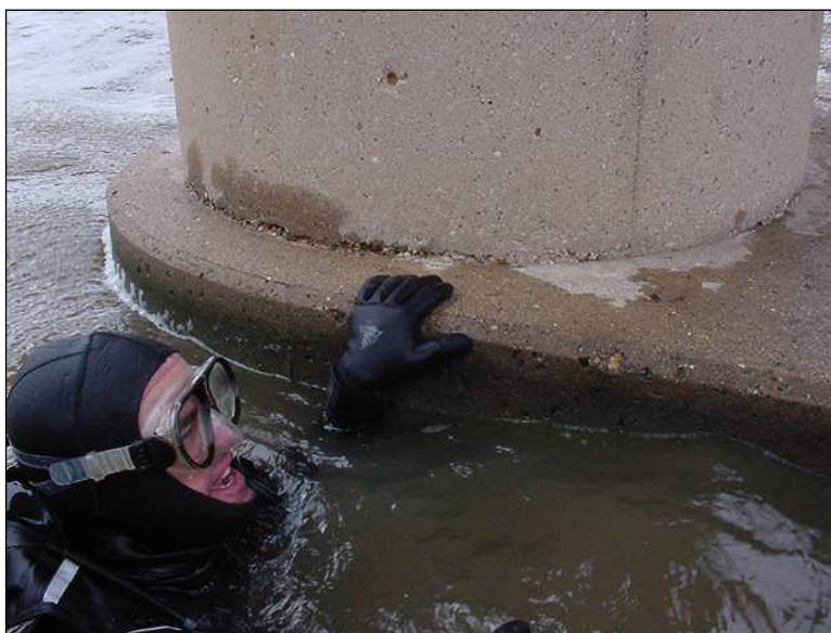
Figure 1.3.8.2-2: Inspector Conducting a Level I Inspection Effort.
