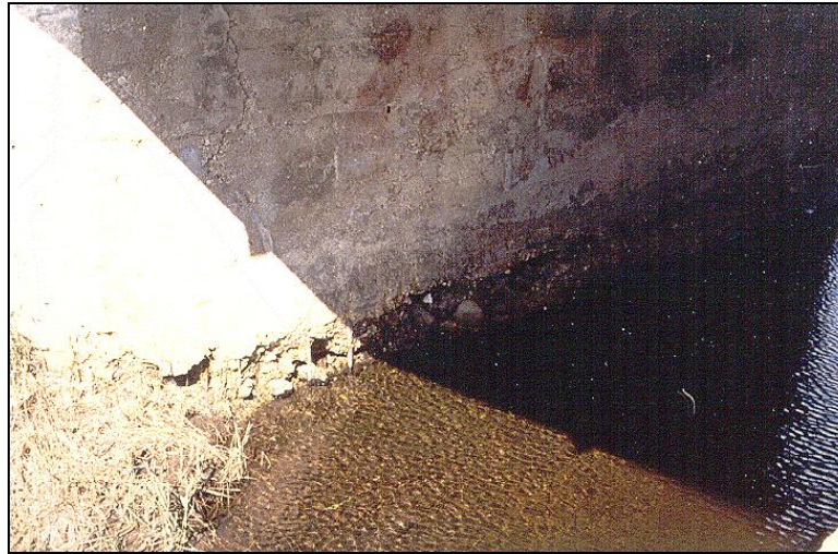
Figure 1.3.6.1-1: Local Scour at the Base of an Abutment.
