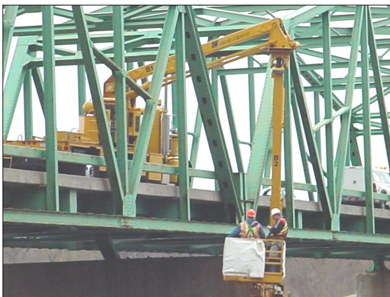
Figure 1.3.5.1-1: Inspectors Performing a NSTM Inspection
