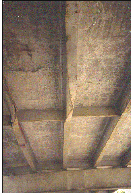
Figure 1.3.12.1-1: Impact Damage to a Steel Girder Bridge.
