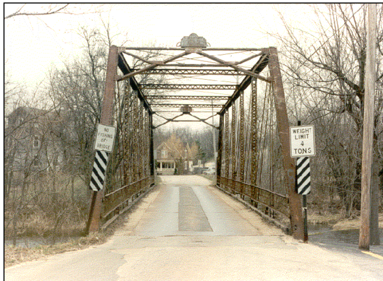
Figure 1.3.16.1-2: Load Posted Truss Bridge.
