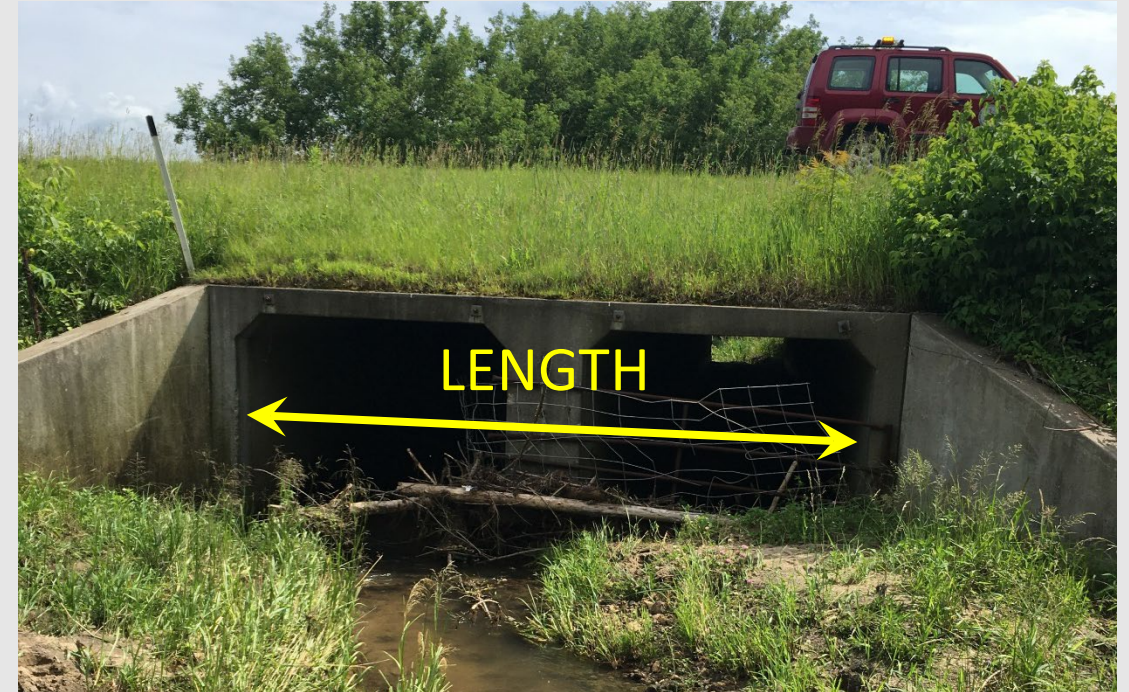
Double Barrel (multicell) Box Culvert
