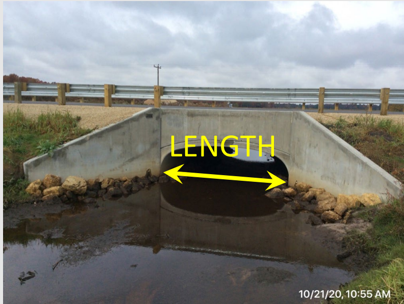
Precast Concrete Arch
