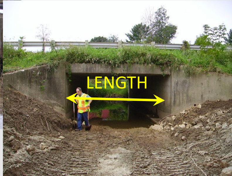
Buried Rigid Frame (no floor)
