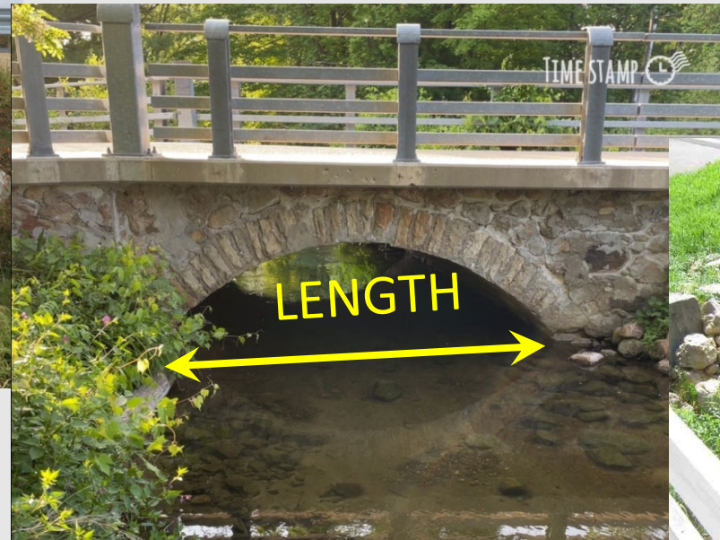
Masonry Arch
