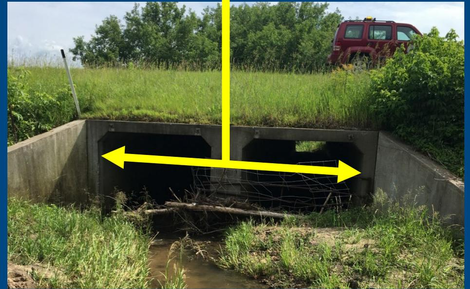
Multi-Cell Concrete Box Culvert
