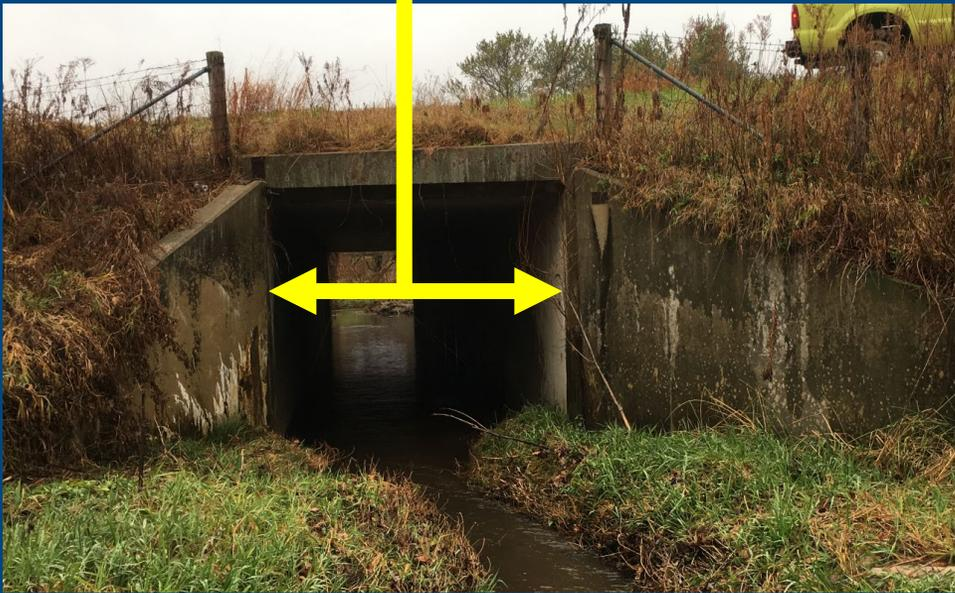
Single-Cell Concrete Box Culvert
