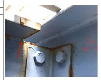
Note: *If* a 1" min. cope is provided, the detail is a Category C, as seen in the 3<sup>rd</sup> photo. Small radii (1<sup>st</sup> photo) or flame cut copes are unclassified but can be less than an E' detail.
