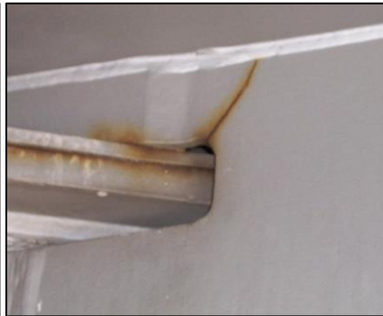
Cracking (1010)
