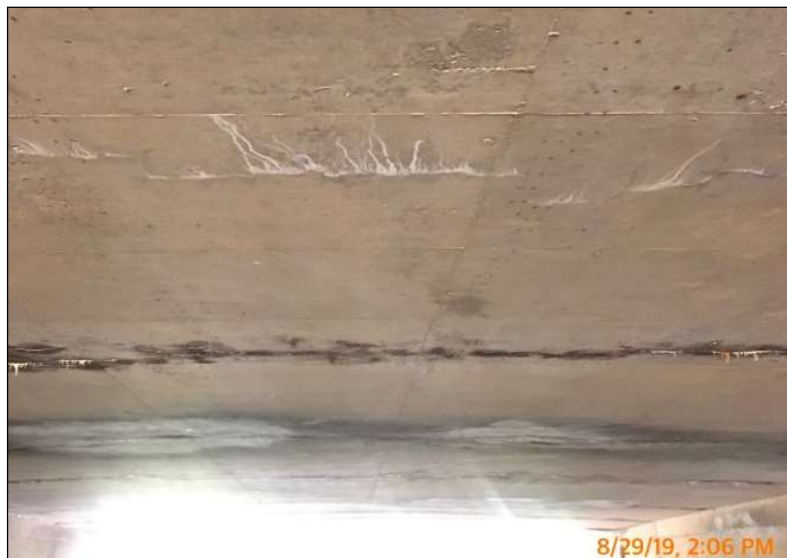
Figure 1.1.1.4-1: Example of exposure adjustment to capture details under structure, resulting in overexposed area at bottom of photo. Better framing to avoid outside area or changing direction photo is taken would improve photo.
