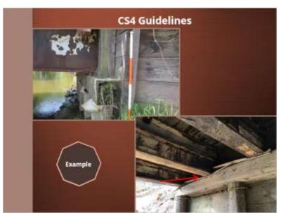
Here are a couple examples of timber pile caps that have crushed.
