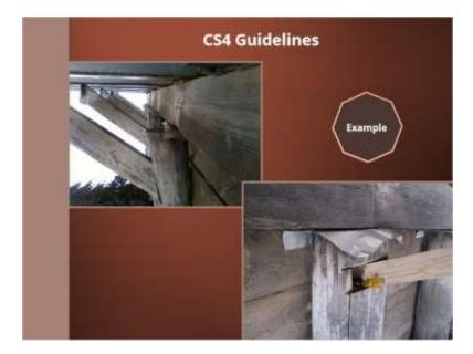
Sometimes this tipping is mitigated by providing braces up to the superstructure. However, this repair introduces other problems. Specifically, a pathway for water infiltration into the interior of the pile has been created. This should be identified as a location susceptible to decay and should be closely inspected.
