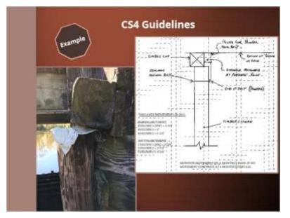
Here is a good example of documentation provided for tipping timber abutment piles. In this example, the inspector has noted measurements and provided a template for taking future measurements to monitor movement.
