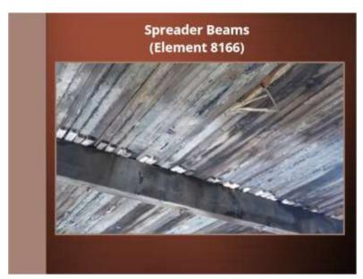
In general, if the inspector feels a spreader beam can or should be tightened and shimmed to improve bridge performance, it should be a recommended maintenance item and the spreader beam should be placed in Condition State 4.
