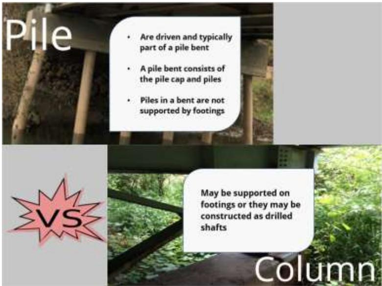
Structural piles are an example of an element commonly miscoded during bridge inspections throughout Wisconsin. Although structural piles function similarly to columns, they need to be coded separately in the element inspection.
