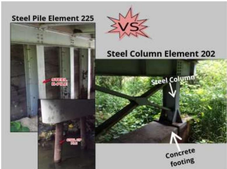
Element 225, Steel pile, and Element 202, Steel Column, are commonly miscoded on inspection reports.
