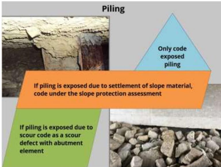
Covered piling, located under an abutment body, should not be reported unless it is exposed.
