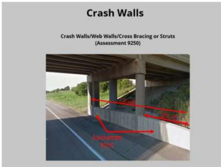
All web walls and most crash walls attached to a pier shall be assessed 20' from exterior columns and coded under (Assessment 9250) The quantity is 1 each per substructure unit.
