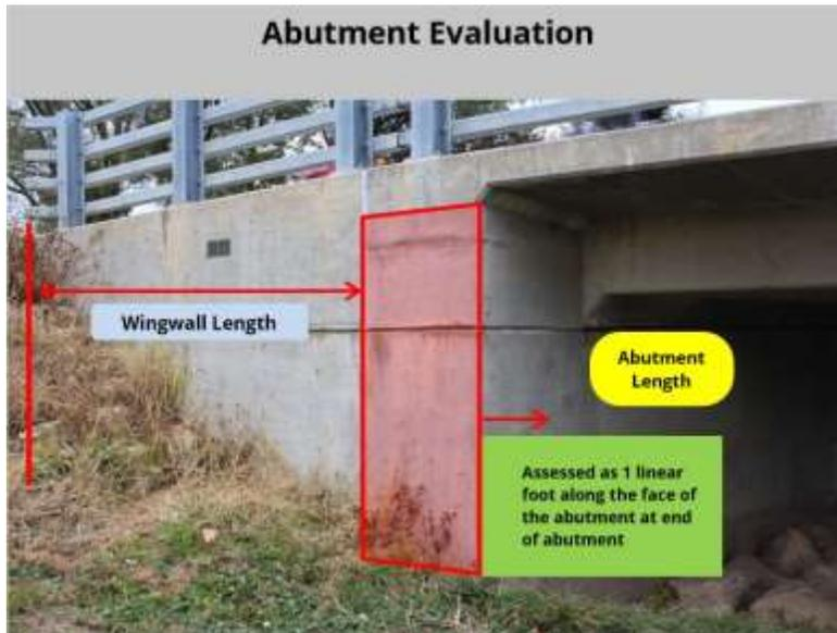
The abutment end shown in the red rectangle above, should be assessed as 1 linear foot along the face of the abutment at each end of abutment, regardless of actual thickness of the abutment.
