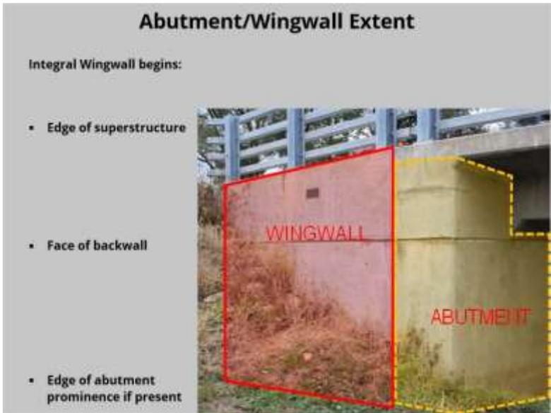
Integral wingwalls begin either at the edge of superstructure, face of backwall or the edge of abutment prominence, if present. For the example shown, the abutment is a sill abutment with an integral concrete wing attached with no joint between the two.
