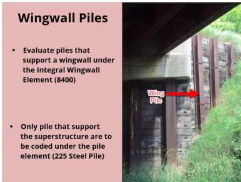
When a bridge has piles supporting the wingwalls, evaluate these piles under the Integral Wingwall Element (8400). Only piles that support the superstructure are to be coded under element 225 Steel Pile.
