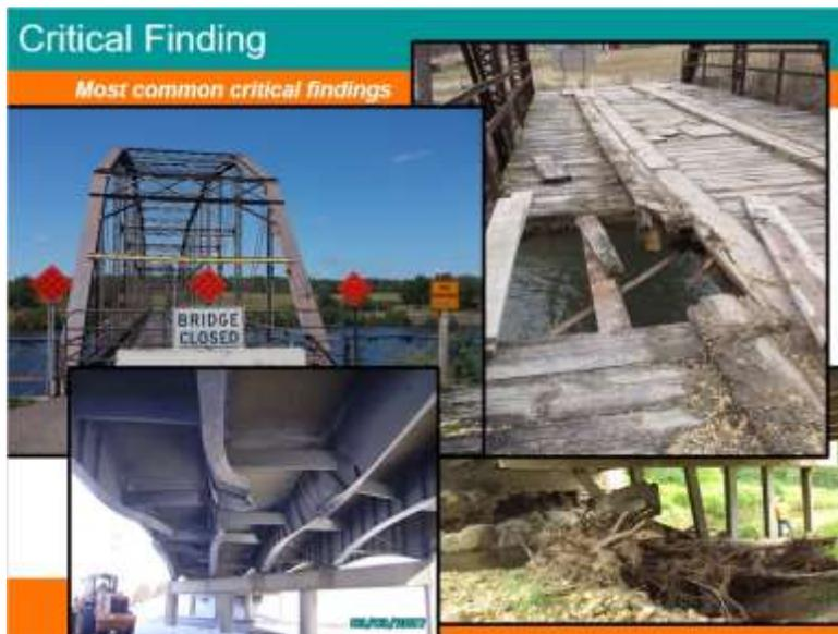
The most common critical findings involve vehicular impact on bridge substructures and superstructures.
