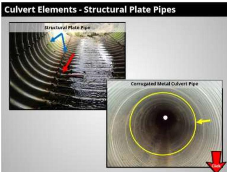
Structural plate culverts could be either steel or aluminum circular or arch culverts. They are field assembled, built-up of several pre-curved corrugated plates. The field assembled plate sections are fastened together with bolts to form a continuous pipe. Fastened plate edges oriented along the barrel length are called seams, while plate edges transverse to the barrel are called joints (blue arrows - note for animation only).
