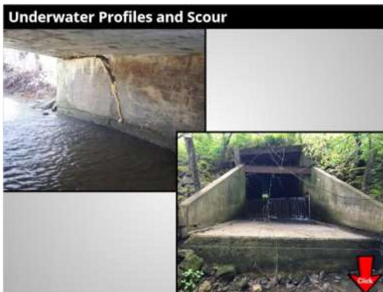
Underwater profiles are generally not needed for box and pipe culverts, as the floor is part of the structural system. Box culvert settlement due to scour or loss of fill can cause serious problems. While underwater profiles are not required for C-structures with structural floors (box culverts), the flow lines, inlets and outlets should be probed for irregularities during inspections and after major flood events to determine if undermining and scour are present.
