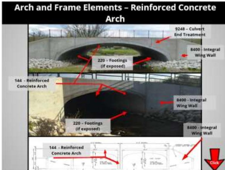
Reinforced concrete arches are the most common arch structures. These can be cast in place, but are generally precast. They can have sloped or vertical walls connecting to the main arch, but are coded the same. Elements for a reinforced concrete Arches are:
