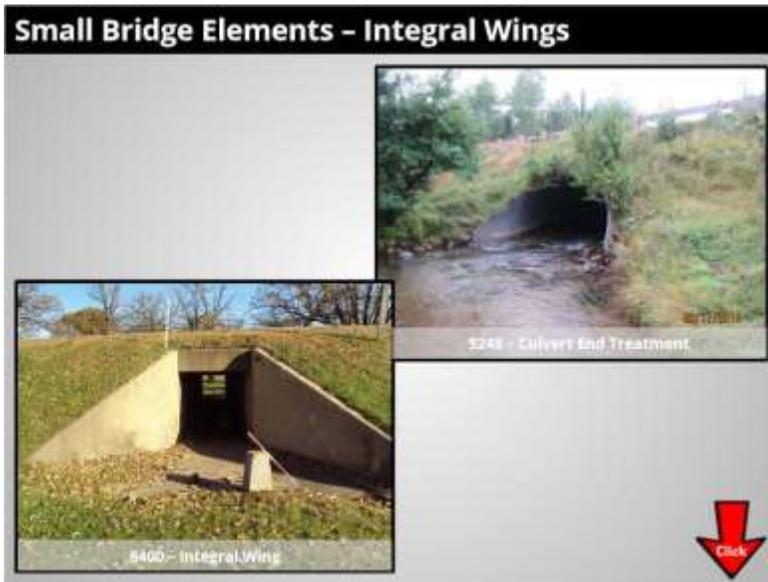
Element 8400 for integral wing walls are anchored to any combination of barrel, apron and/or headwall. Integral wings are typically reinforced concrete, but may be any material with a vertical or near vertical face.
