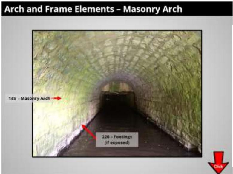
Masonry arch elements are stone or brick structures formed into the form of an arch. These structures rest on a footing, which may or may not be exposed, and have head walls and wings to retain fill.
