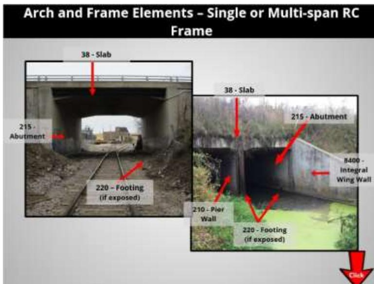
The first type is the single or multiple span rigid concrete frame. Similar to arches in that they are 3-sided structures, rigid frames have vertical walls connected by slabs with haunches and are similar to slab bridge structures. They do not have a structural floor slab.
