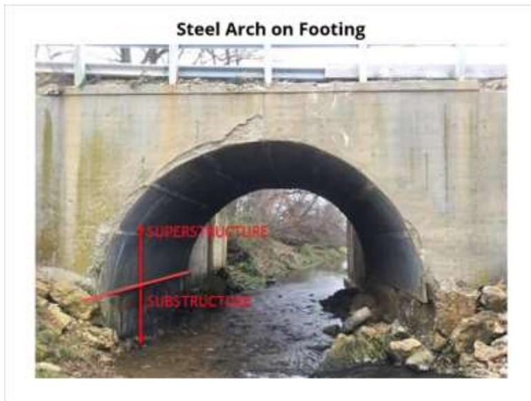
For a steel arch on a footing, the concrete footings, if exposed, are considered the NBI substructure and everything above is considered NBI superstructure. For any of these cases when the footing is not exposed rate the substructure the same as the superstructure.
