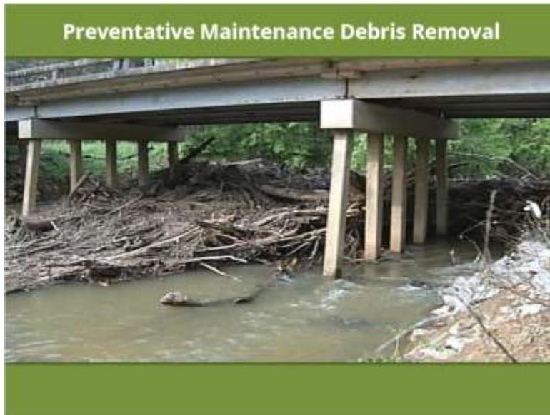
Not all preventative maintenance actions are cyclical. Some are based on external conditions that occasionally pop up on structures. One common action is removal of debris after significant flooding of a waterway. Often bridge abutments and piers can “catch” floating debris.
