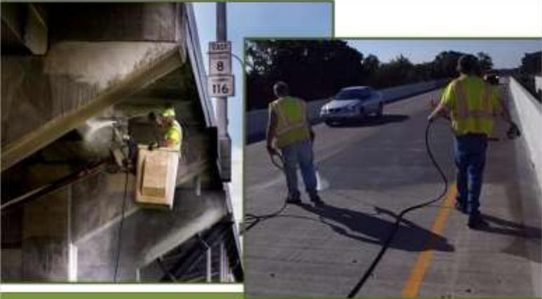
One of the most common preventative maintenance actions used by WisDOT is bridge washing. Washing is important due to the quick build-up of debris, bird droppings, and chlorides on critical components of the bridge. In a short period of time, those items can accelerate the deterioration of both concrete, steel, and timber bridge members.
