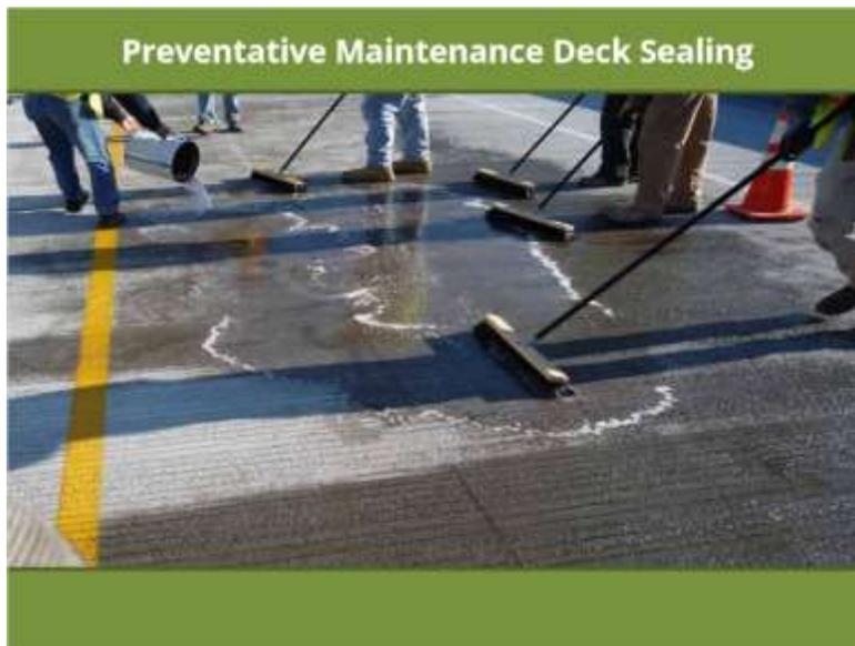
In addition to crack sealing, an important activity to maintain a bridge structure involves deck sealing. Deck sealing involves flooding the deck with an approved sealing product that works to significantly slow the ingress of chloride ions into bridge-deck concrete, thus slowing deterioration of the structure.
