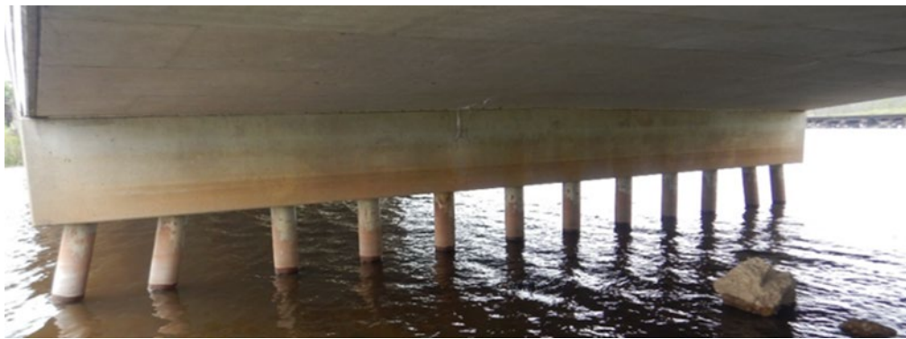
Figure 1 – Typical pile bent pier
