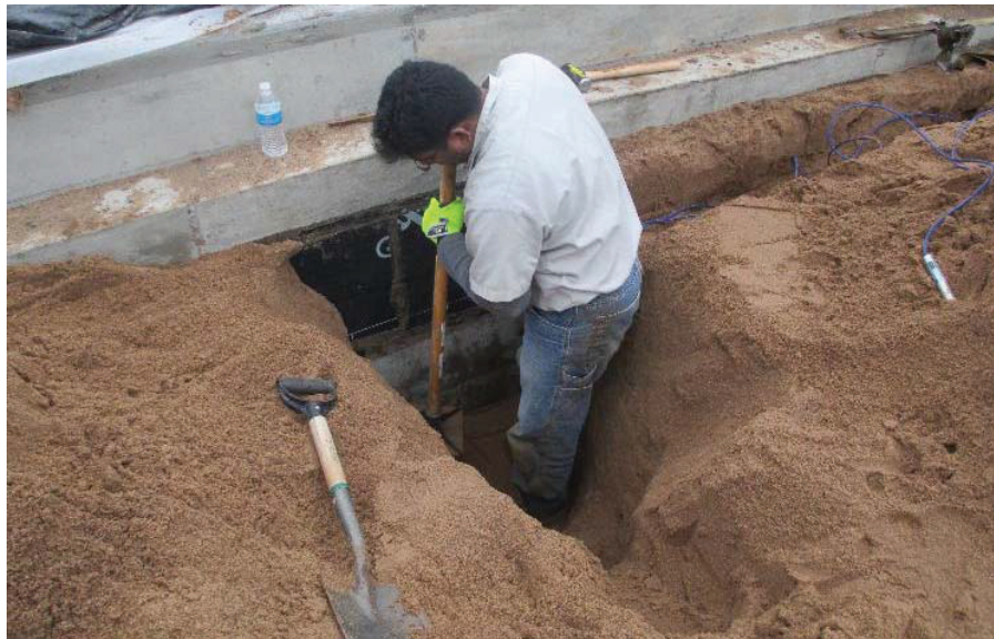
Figure 88. Compaction of backfill material in thin layers after installing PP and EPC sensors at multiple depths
