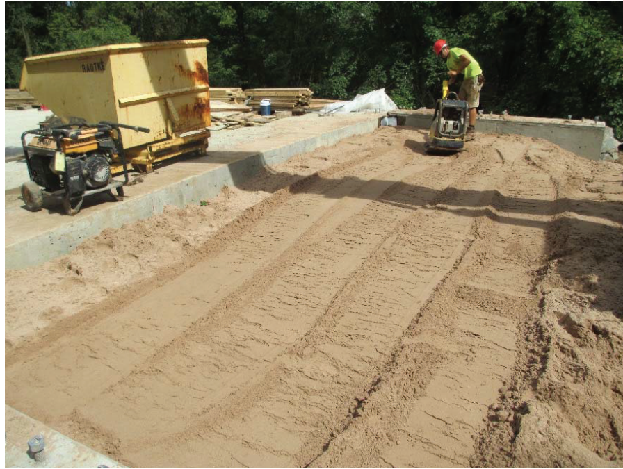
Figure 102. Compaction of backfill at Schwartz Road Bridge
