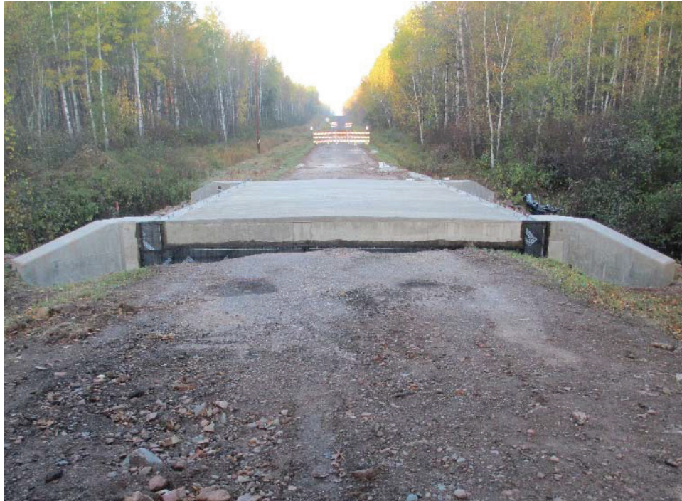
Figure 116. Hobbles Creek Bridge west abutment before backfilling
