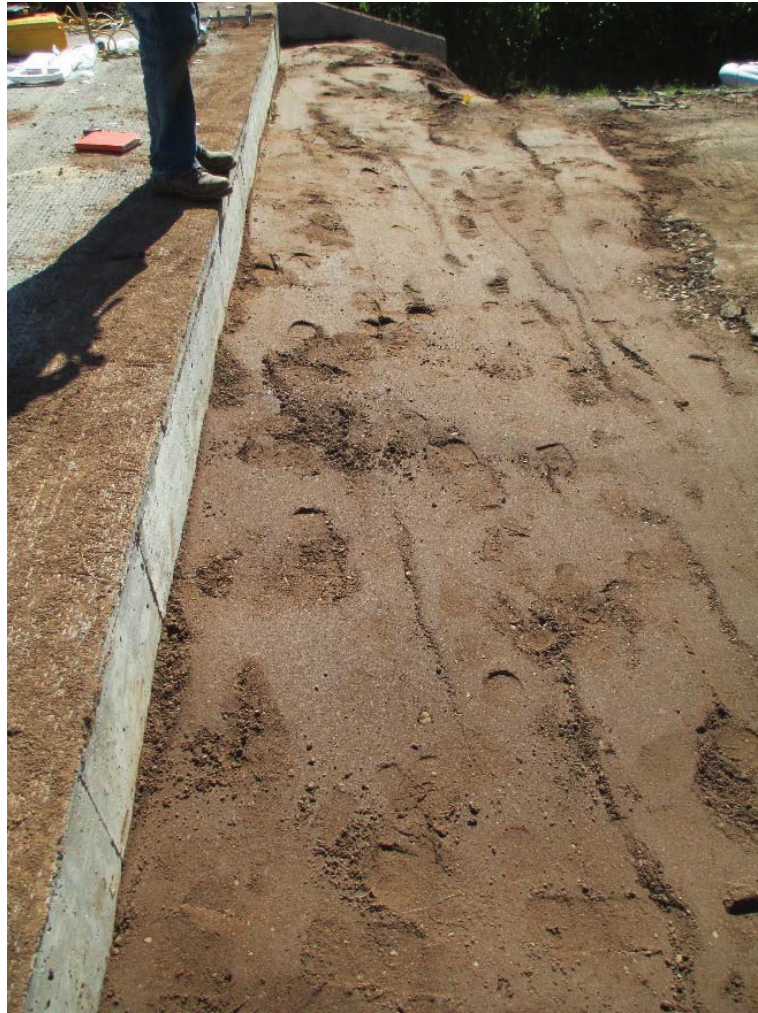
Figure 118. Hobbles Creek Bridge after backfilling
