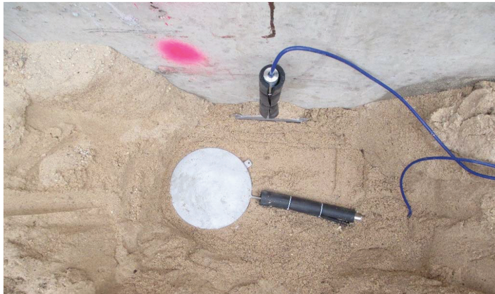
Figure 140. Sensor installation behind Badger Road Bridge
