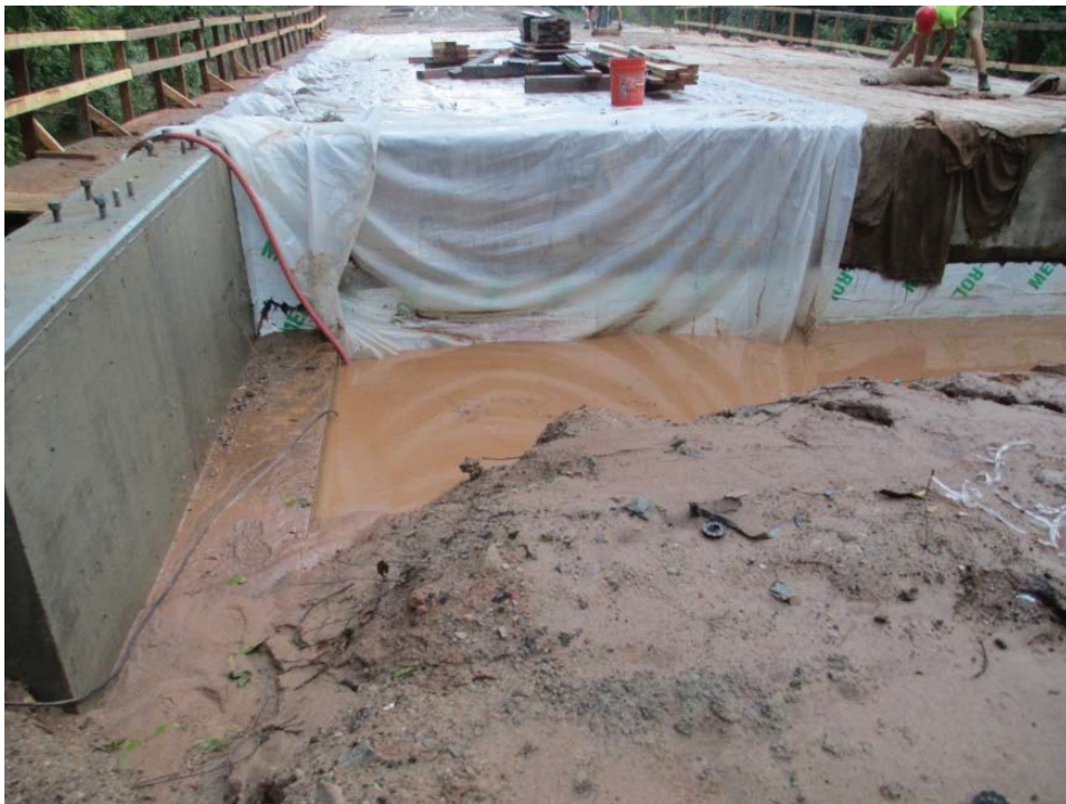
Figure 100. Ponded water in the abutment excavation at Schwartz Road Bridge
