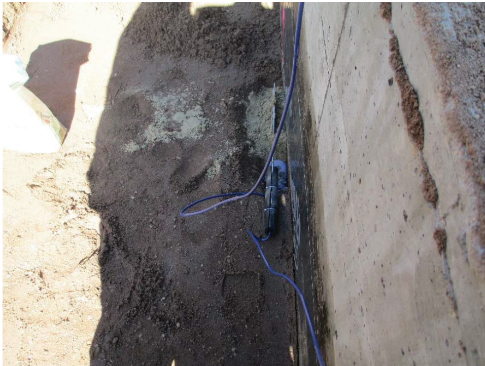
Figure 126. Lateral EPC installation at Hobbles Creek Bridge
