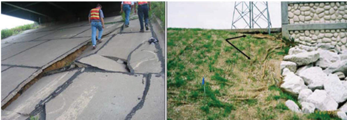
Figure 2. Examples of (left) severe damage of concrete slope protection due to erosion on I-380 bridge over Hwy 6 in Iowa (White et al. 2005), and (right) slope instability on West Beloit Road Bridge over Root River in Wisconsin (Helwany et al. 2007)
