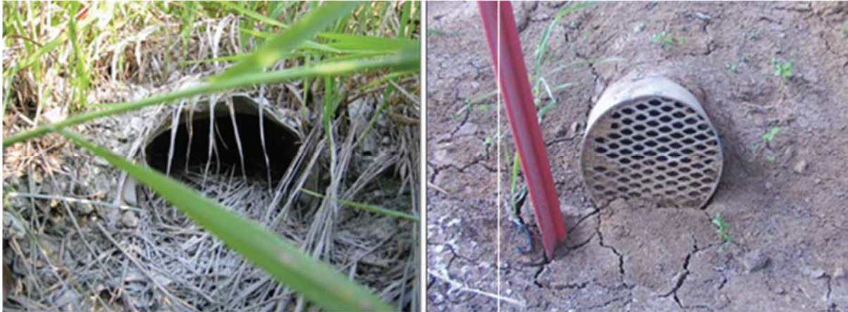
Figure 1. Examples of clogged end drains at I-80 bridge over McPearson Avenue (left) and the bridge on US 218 over South Skunk River (right) (White et al. 2005)
