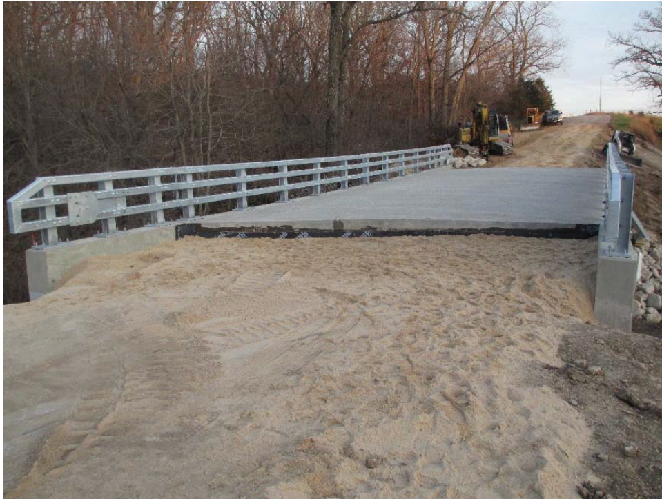
Figure 134. Badger Road Bridge after backfilling abutment
