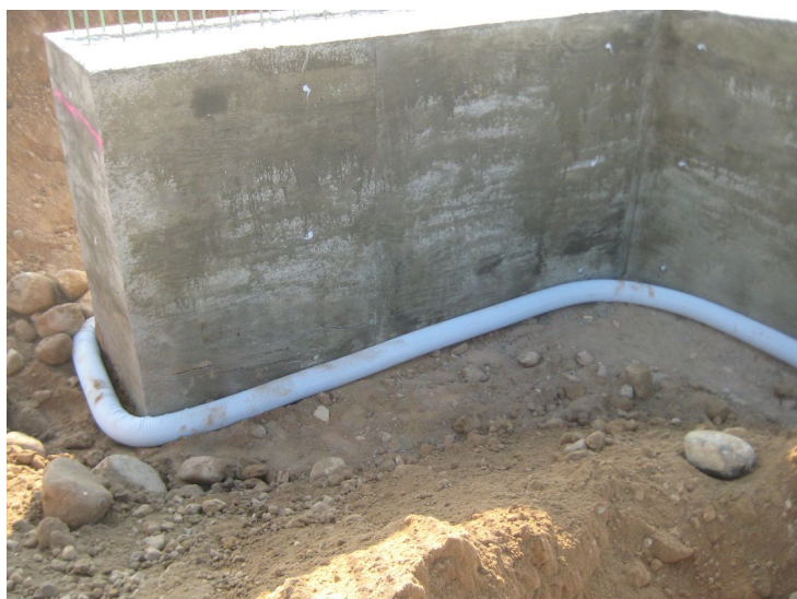
Figure 5.5. Perspective of Fissured Flooded-Compacted Backfill (right). Drain Tile at the Base of the Abutment Wing Wall (left).
