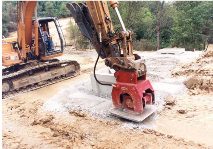
Figure 1.1. Backhoe Outfitted with Vibrating Plate Compacting Fill. Often this type of operation is performed hastily before an inspector can arrive at the site to check the quality of the compaction.
