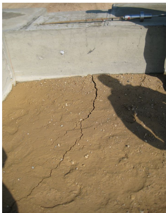
Figure 5.5. Perspective of Fissured Flooded-Compacted Backfill (right). Drain Tile at the Base of the Abutment Wing Wall (left).
