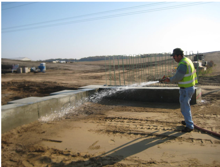
Figure 5.2. Flooding the Backfill to Initiate Compaction by Drainage. Just one water truck and one member from the contractor team was needed for the operation.
