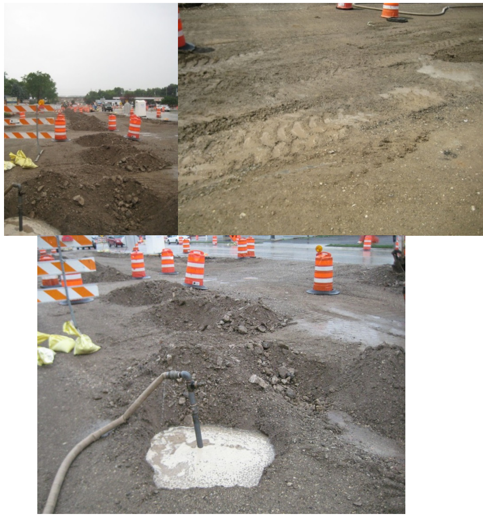
Figure 5.17. Pictures of Jetting Operation at Greenfield Avenue. Excavated Application Points (top left). Truck Compaction Treads After Filling Application Points (top right). Rigid Cast Iron Pipe Jetting Below Top of Subgrade (bottom).
