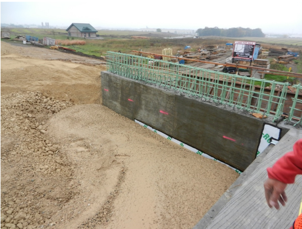
Figure 5.9. Complete flooding of the backfill. Please note that the stone are now visible soon after the completion indicating the drainage characteristics of the solid material in the slurry.
