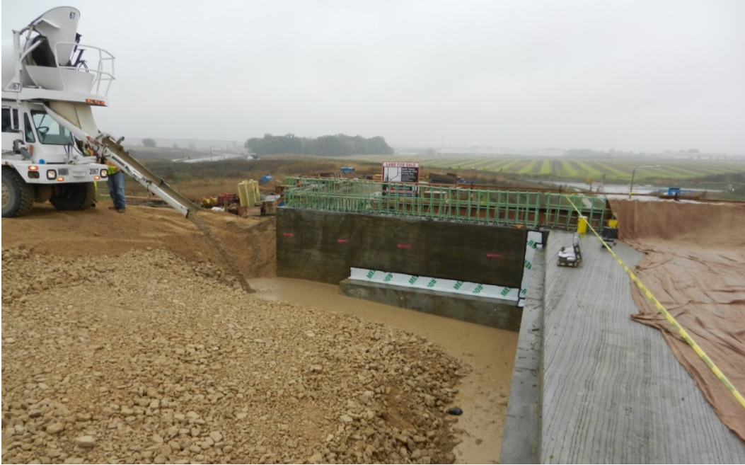
Figure 5.8: Construction of the backfill using slurry flooding compaction technique.
