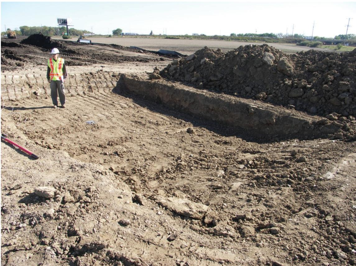
**Figure 4.27:** View of the testing site in the town of Sylvania west of Interstate 94 near Racine, WI. At the site, the WisDOT contractor dug out a trench where the different soil lifts thicknesses were tested.
