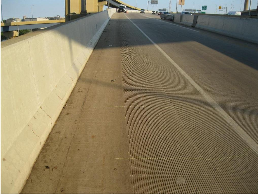
**Figure 128. IH 43 northbound to Michigan Avenue Span 1 transverse cracks**
