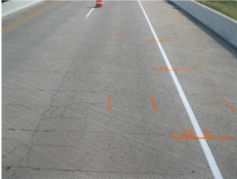
**Figure 56. US 151 northbound over STH 26 Service Road bridge deck surface cracking**
