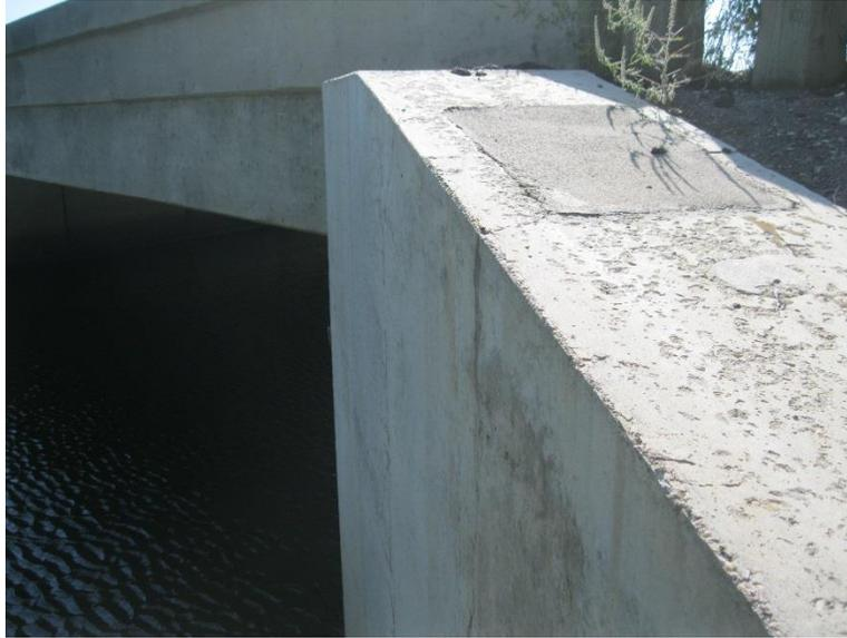
**Figure 142. US 63 over the Rush River wingwall cracking at grout pocket vertical surface**
