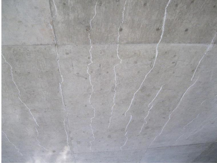
**Figure 50. SH 40 over Hay Creek transverse cracking on superstructure underside**
