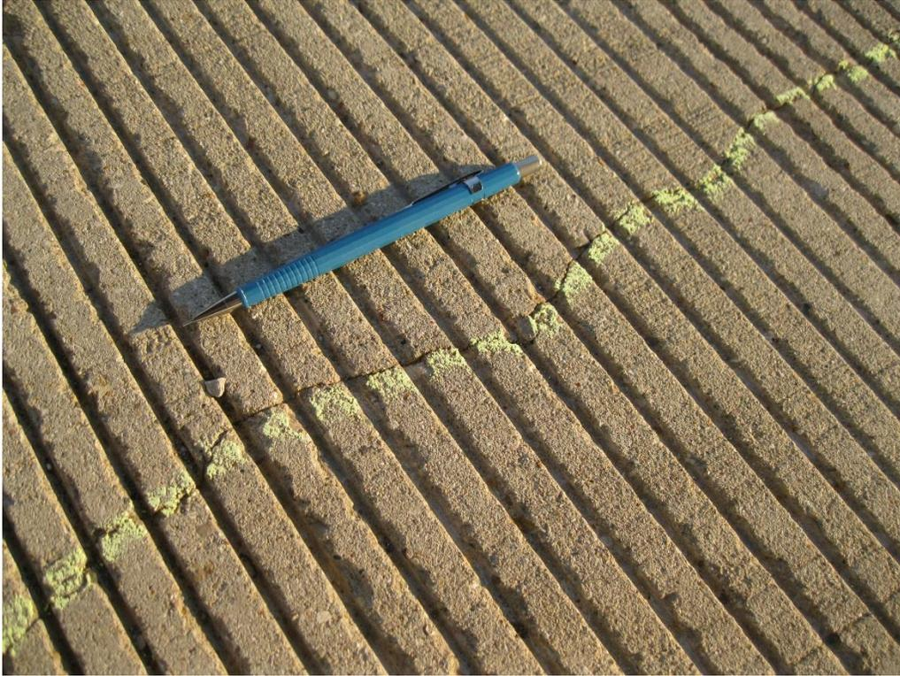
**Figure 127. IH 43 northbound to Michigan Avenue typical transverse crack size**
