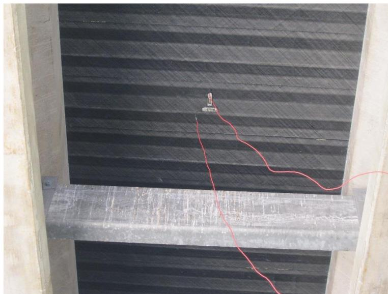
**Figure 60. US 151 northbound over STH 26 Service Road deck strain gage pairing**
