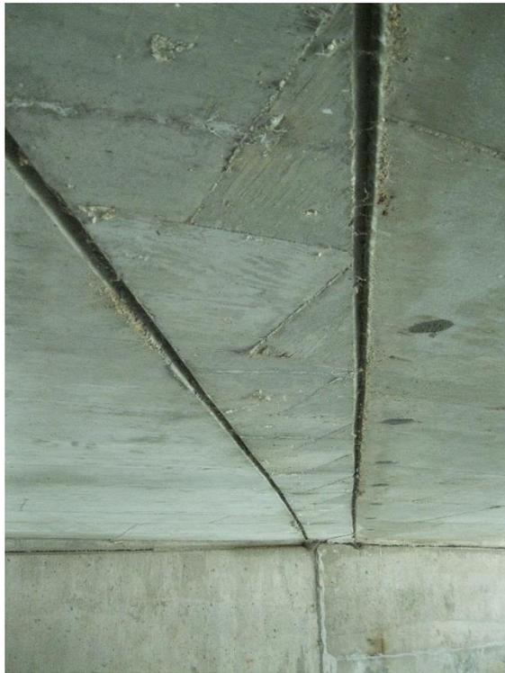
**Figure 124.STH 33 over the Milwaukee River closure pour close-up**
