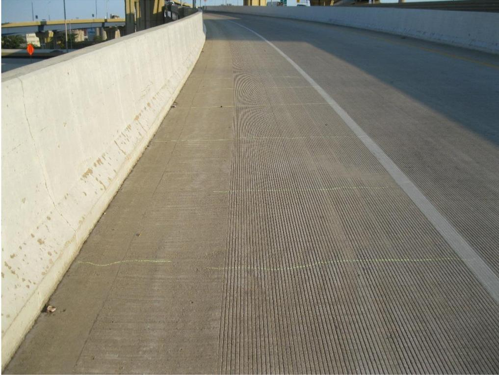
**Figure 130. IH 43 northbound to Michigan Avenue Span 3 transverse cracks**
