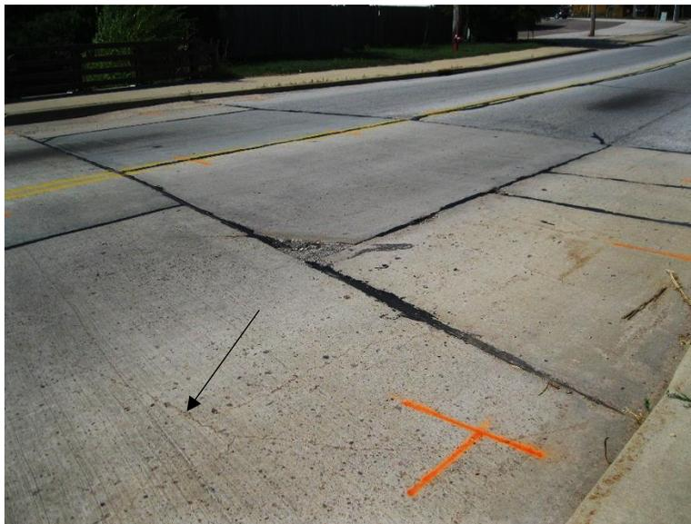
**Figure 105. US 12 over Coffee Creek deck crack – 3**
