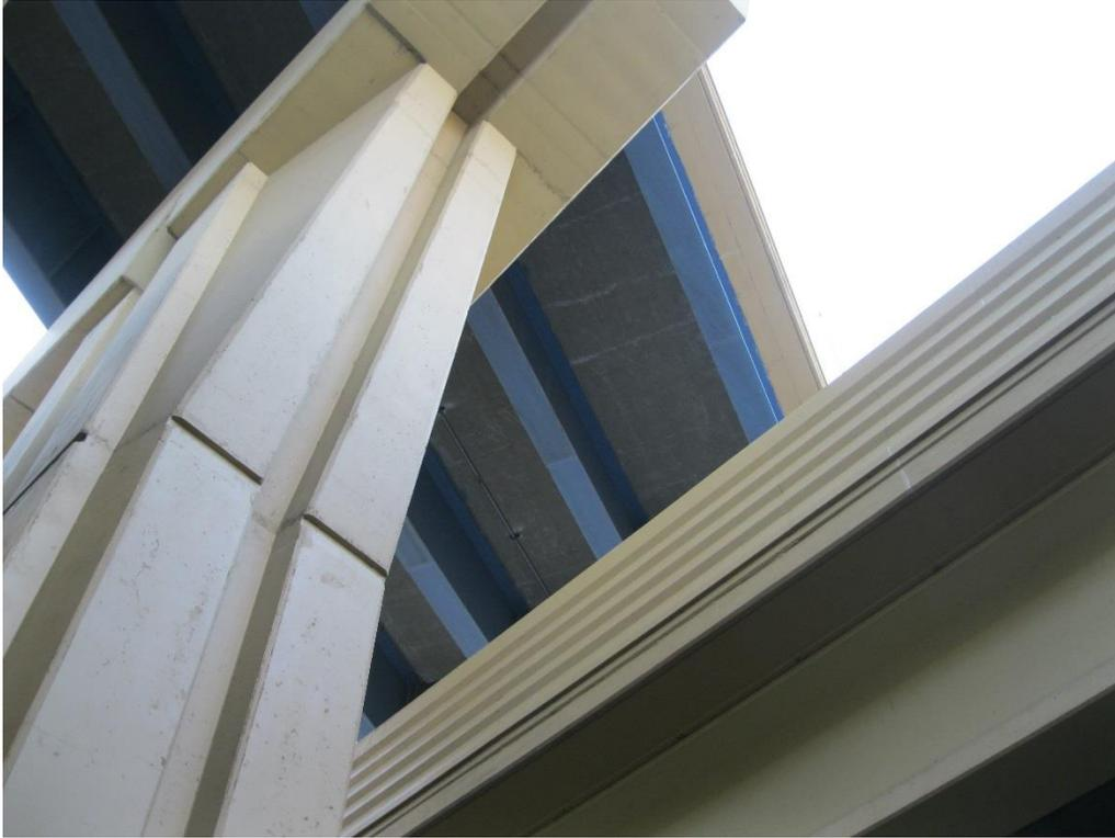
**Figure 134. IH 43 northbound to Michigan Avenue chloride staining on deck underside – 1**
