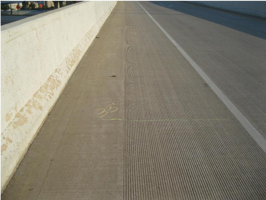
**Figure 131. IH 43 northbound to Michigan Avenue Span 4 transverse cracks**
