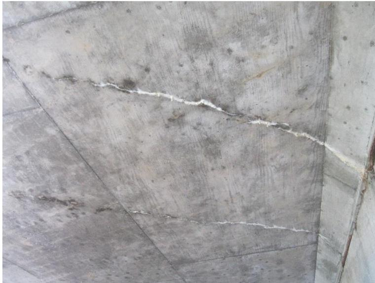
**Figure 139. US 63 over the Rush River cracking in cast-in-place deck at abutment**
