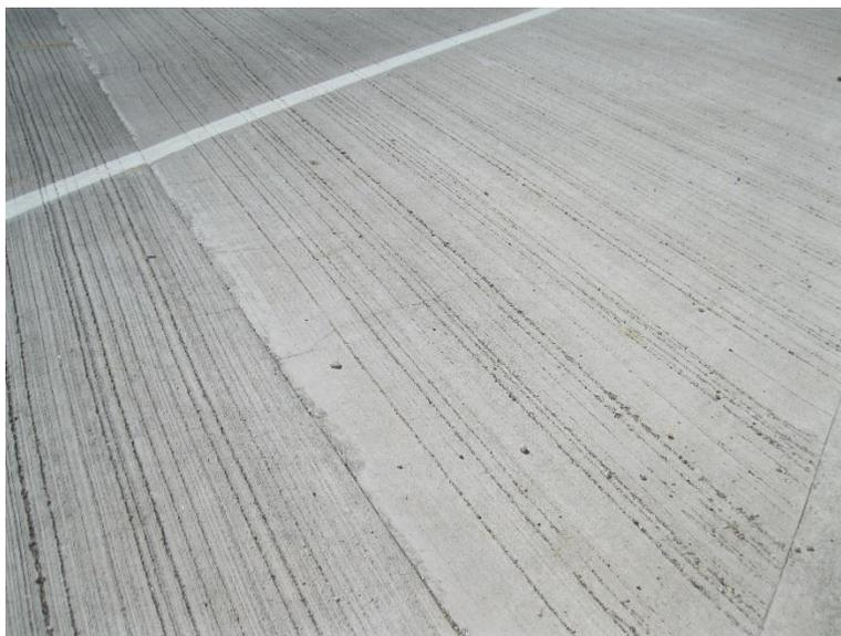
**Figure 3. STH 19 over Token Creek Tributary minor cracking at bridge entrance**
