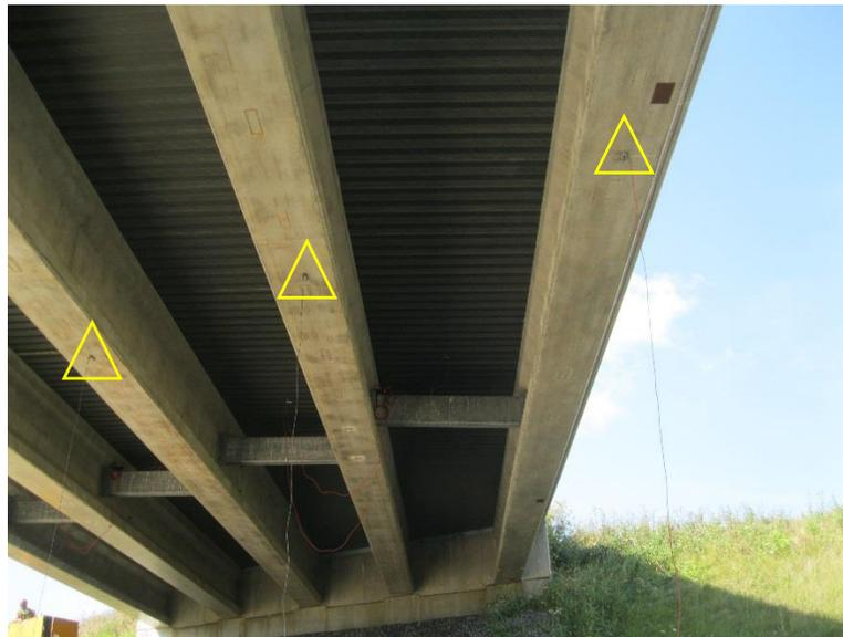
**Figure 59. US 151 northbound over STH 26 Service Road girder strain gages**
