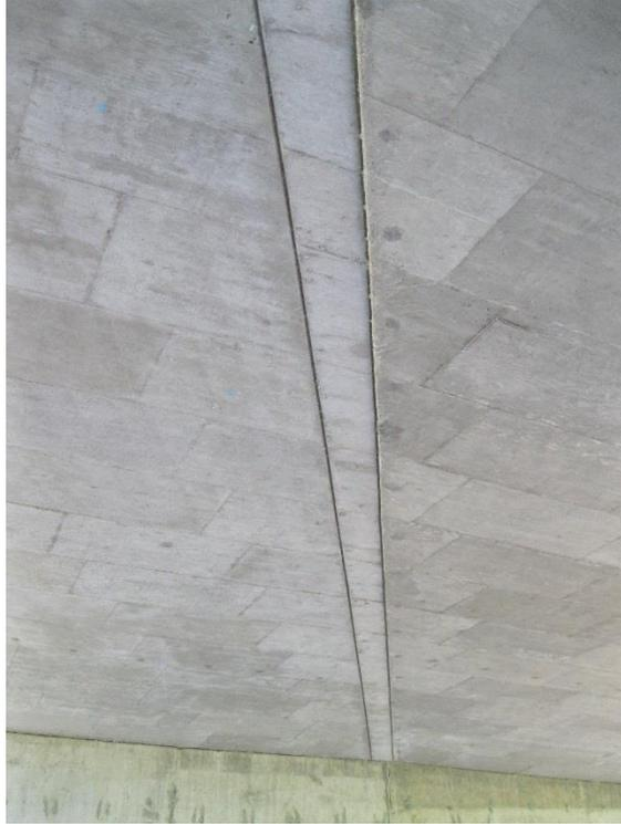
**Figure 123.STH 33 over the Milwaukee River closure pour condition**
