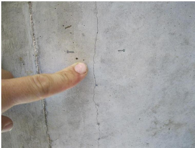
**Figure 51. SH 40 over Hay Creek typical size of transverse cracking**
