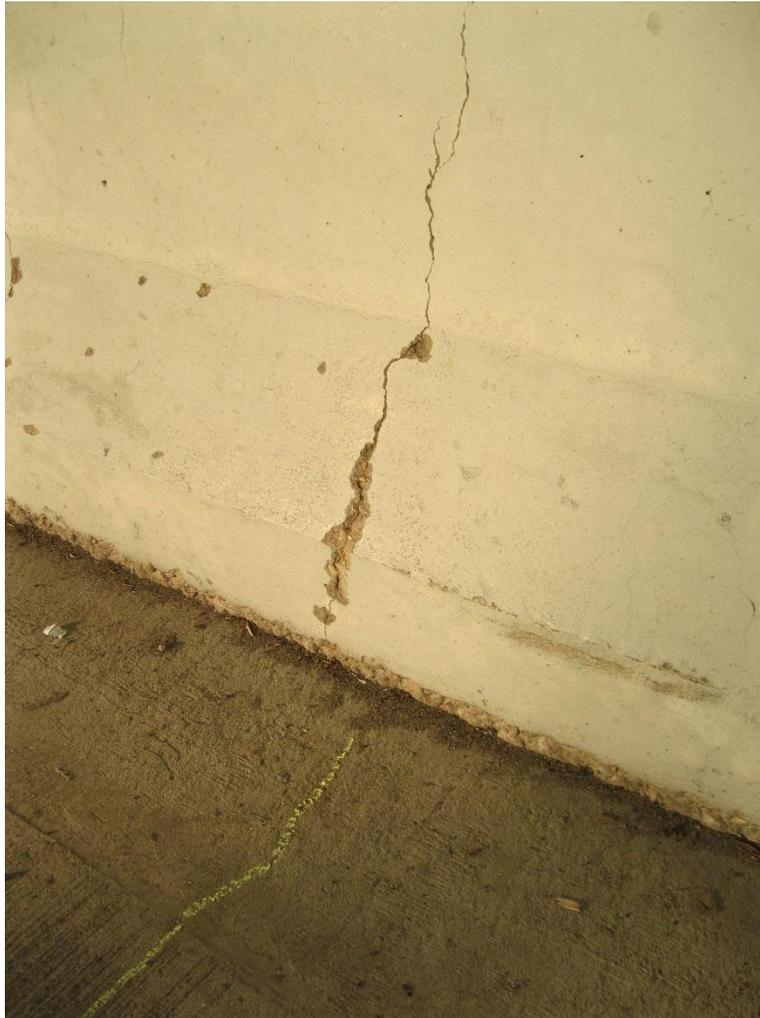
**Figure 132. IH 43 northbound to Michigan Avenue parapet wall crack**
