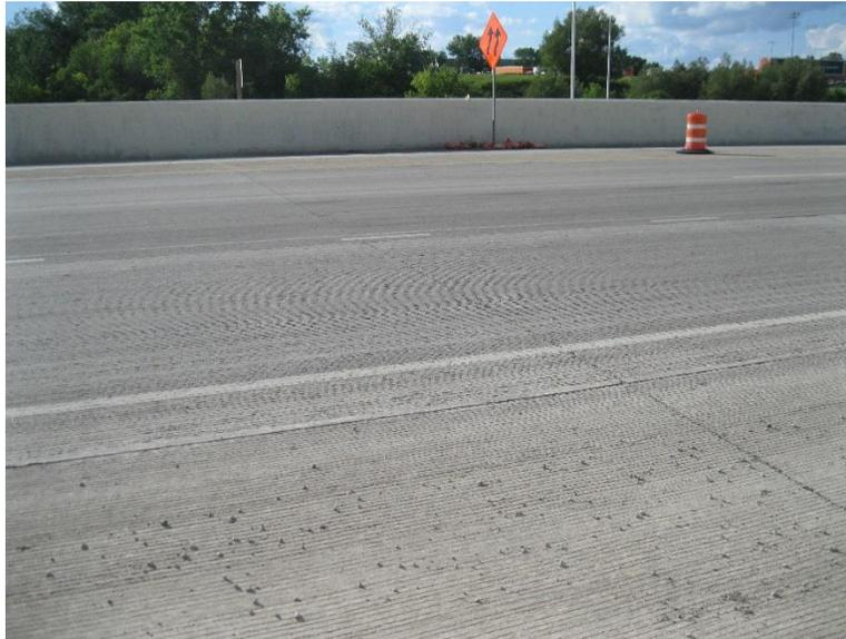
**Figure 26. US 41 over Ashwaubenon Creek roadway surface condition**
