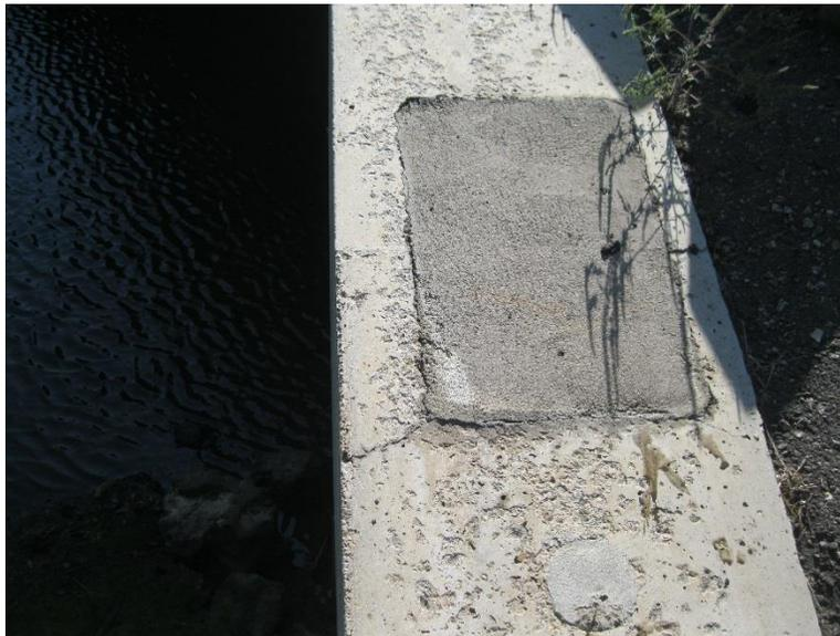
**Figure 141. US 63 over the Rush River wingwall cracking at grout pocket top surface**
