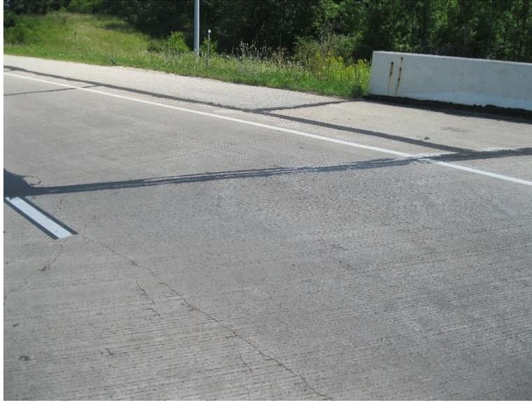
**Figure 92. US 151 over De Neveu Creek deck surface condition – 7**
