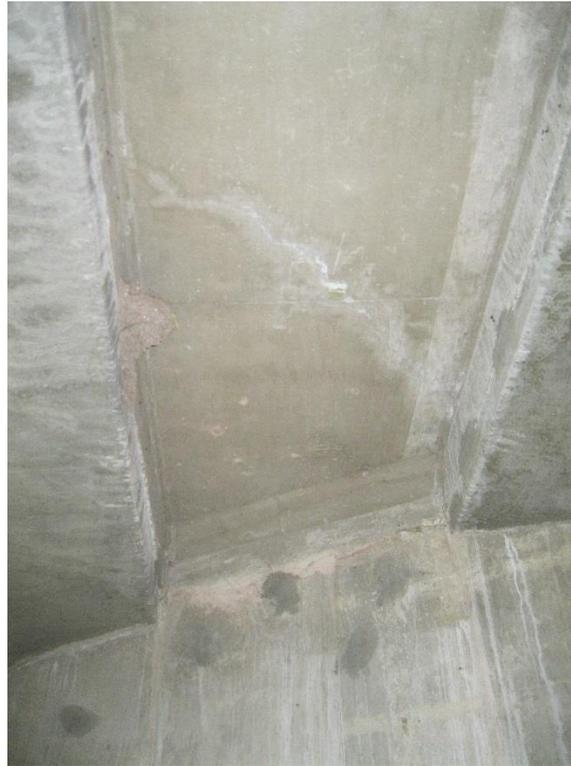
**Figure 94. US 151 over De Neveu Creek hairline cracking at bridge end**
