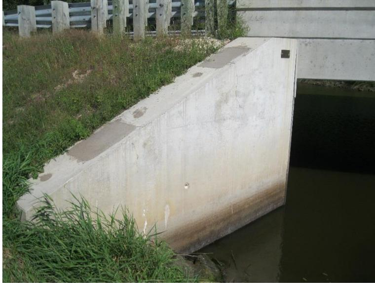
**Figure 140. US 63 over the Rush River wingwall-exposed grout pockets**
