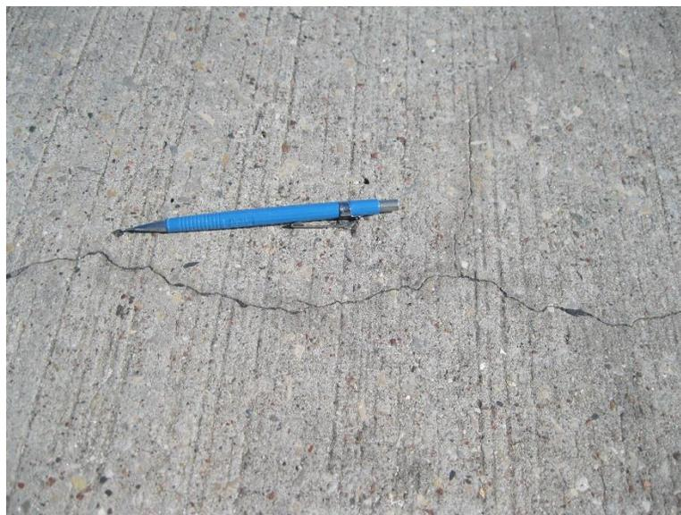
**Figure 39. US 141-Main Street over the Fox River typical crack size observed**
