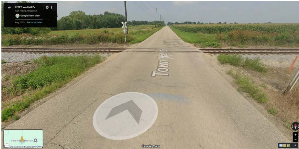
Figure 14. An example of a Wisconsin railroad crossing that lacks safety shoulders.
