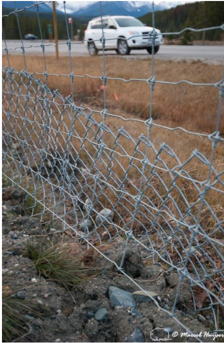
Figure 111. Wildlife fence and dig barrier (or “apron”), mostly for canids and bears ( Ursus sp. ), Trans-Canada Highway, Banff National Park, Alberta, Canada. The dig barrier angles away from the road.
