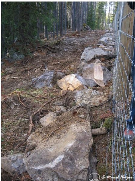
Figure 112. If a dig barrier cannot be dug into the soil, angling it away from the road and covering it with soil and rocks and boulders may be an option. Trans-Canada Highway, Banff National Park, Alberta, Canada.
