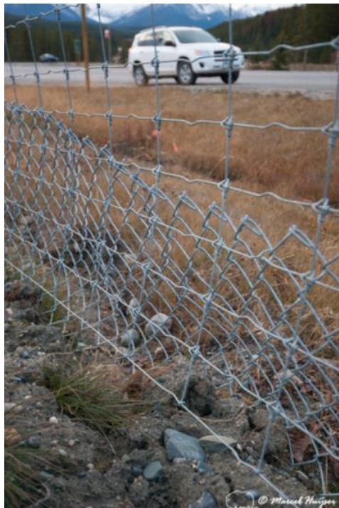
Figure 81. Wildlife fence and dig barrier ("buried fence" or "apron"), Trans-Canada Highway, Banff National Park, Alberta, Canada. The dig barrier in the soil angles (45°) towards the safe side or habitat side; it angles away from the fence and the road on the other side (Clevenger and Huijser 2011). The dig barrier keeps animals from digging under the fence. The dig barrier may consist of a 4-5 ft (1.0-1.2 m) wide galvanized chain-link fence that is attached to the bottom of the actual fence. The buried fence should extend approximately 3.5 ft (1.1 m) under the ground (Clevenger & Huijser, 2011).
