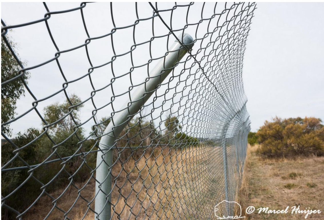
Figure 115. Fence designed to keep koala ( Phascolarctos cinereus ) off the highway, M79, between Harcourt and Faraday, Victoria, Australia. This fence is about 2.1 m high, and the top 50 cm or so angles away from the road. The last 30 cm or so is not supported by the post and forms a 'floppy top' making it difficult to cross by species that climb well.
