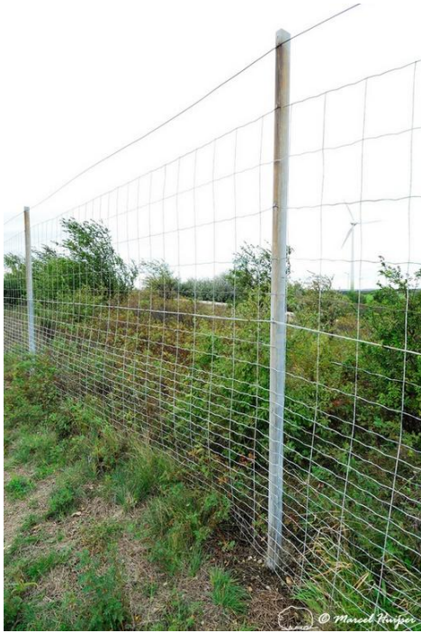
Figure 109. Mesh wire wildlife fence with metal poles on top of multifunctional overpass (wildlife, bicyclists, pedestrians; about 100 m wide), across A4 motorway, Parndorf, Austria. The overpass is designed for farmers, agricultural machinery, hunters and wildlife including roe deer ( Capreolus capreolus ) and European hare ( Lepus europaeus ). Mesh size is small towards the bottom.
