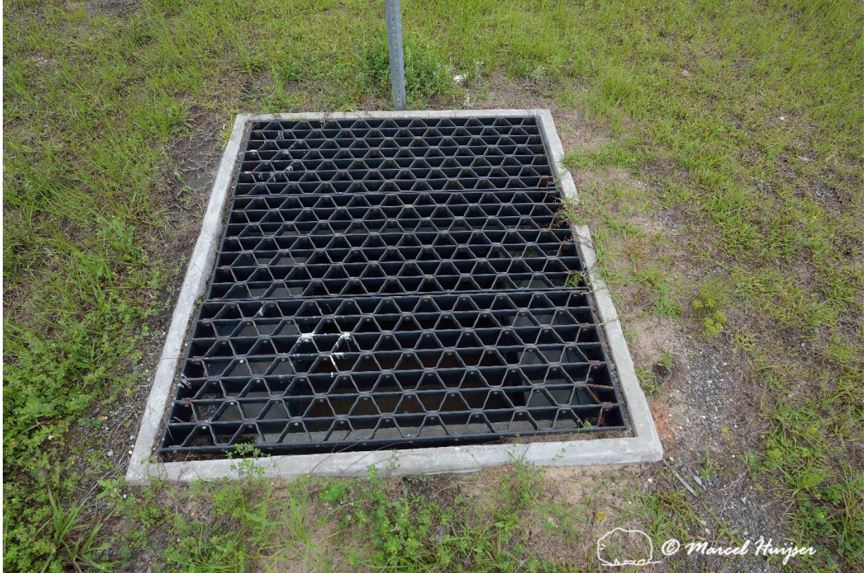
Figure 138. Opening (with bridge grate cover) in median to allow light and moisture in the wildlife underpass Hwy 331 Hwy 83 near Freeport Florida USA.
