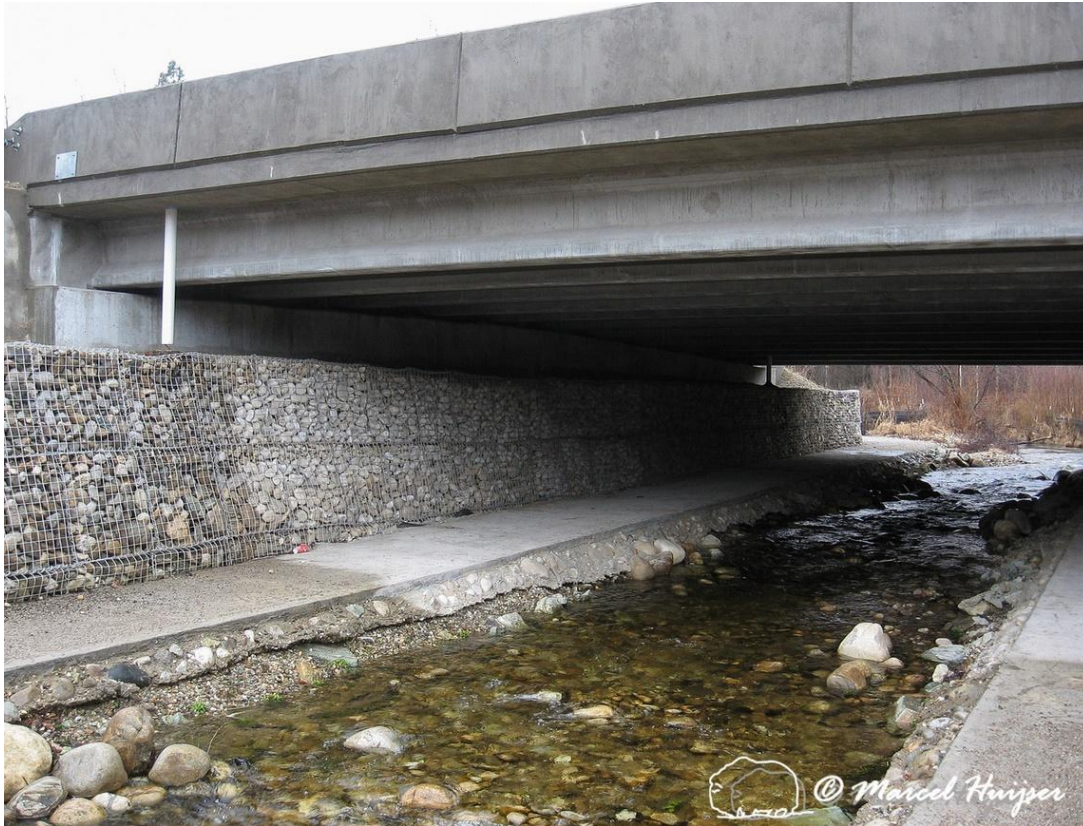
Figure 133. Pathway for large mammals in an underpass (bridge) primarily designed for water (stream), US Hwy 93 S, Bitterroot Valley, Montana, USA.
