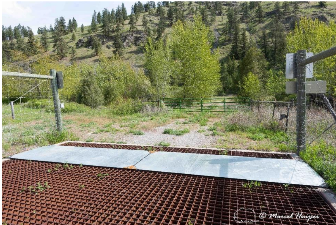
Figure 89. Electrified barrier, designed for low traffic volume and low traffic speed, on top of a wildlife guard at an access road to US Hwy 93S, near Ravalli, Montana, USA.
