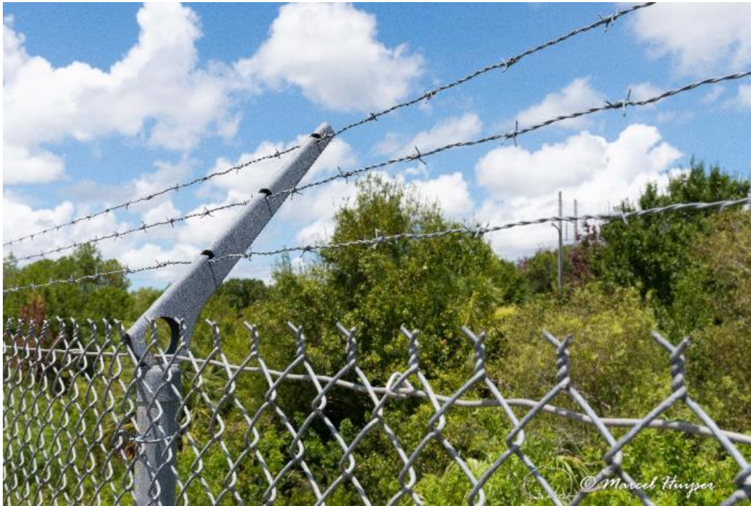
Figure 82. Outrigger or overhang on a fence for Florida panther ( Puma concolor coryi ), SR 29, Florida, USA. Note that the outrigger faces the safe side, the habitat side of the fence. One may consider a longer overhang from chain-link fence material.
