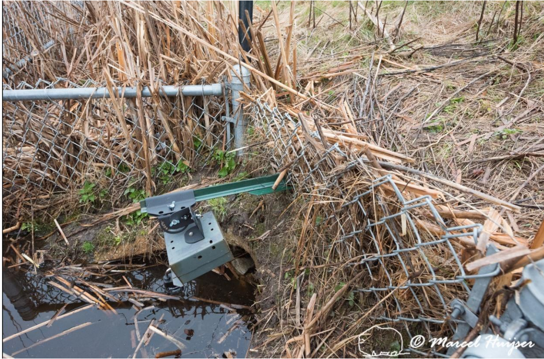
Figure 139. Turtle fence tied into an existing culvert for hydrology, US Hwy 83, Valentine National Wildlife Refuge, Nebraska. The camera monitors potential turtle crossings at the culvert.
