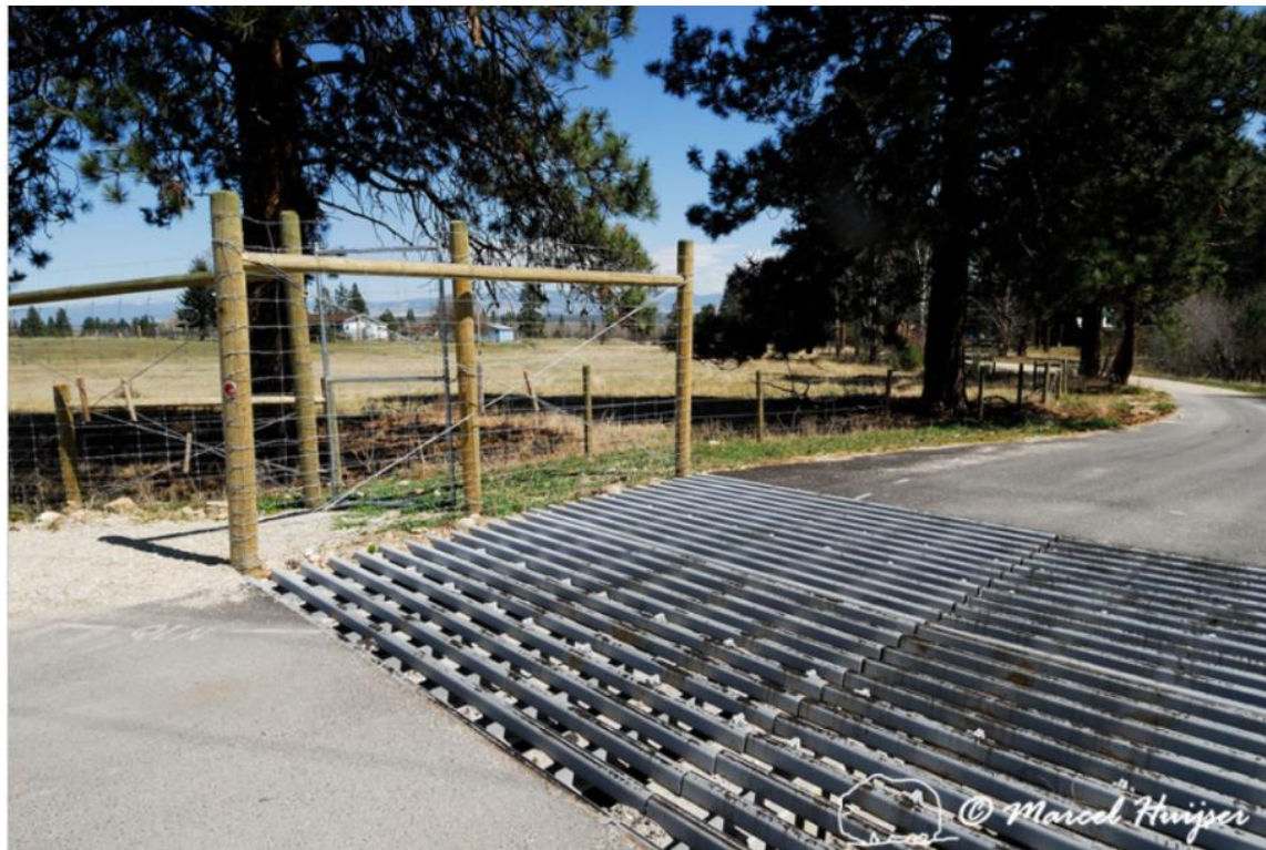
Figure 88. Wildlife guard at an access road to US Hwy 93S, near Victor, Montana, USA. This type of wildlife guard is less suited for pedestrians and cyclists.
