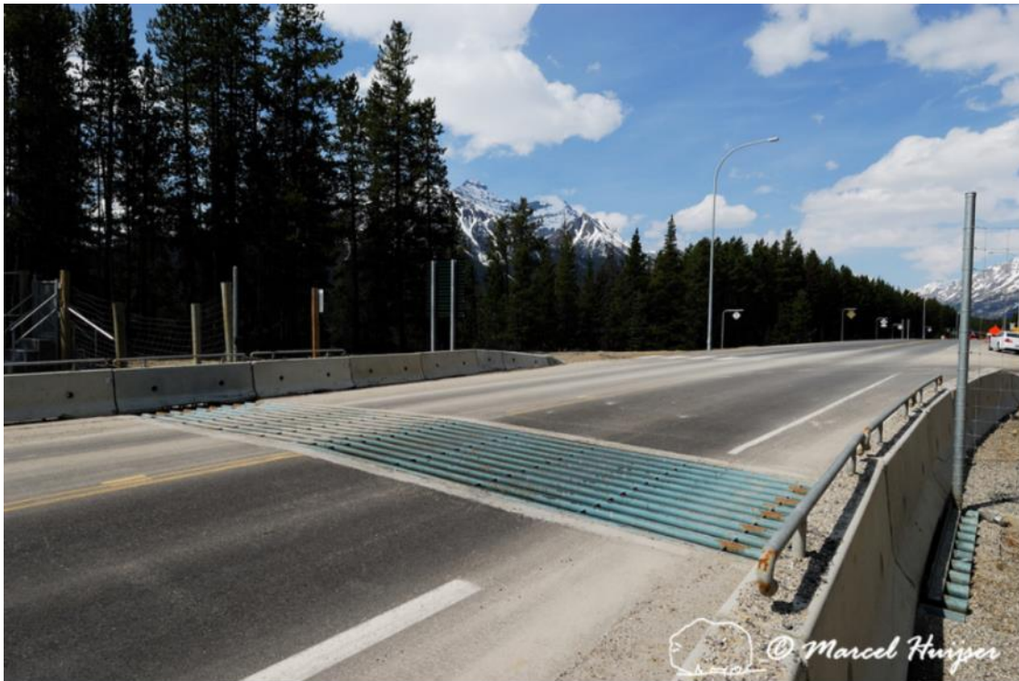
Figure 86. Fence-end brought close to the edge of the pavement, protected by Jersey barriers. Also note that there is a wildlife guard embedded in the travel lanes, Alberta, Canada.
