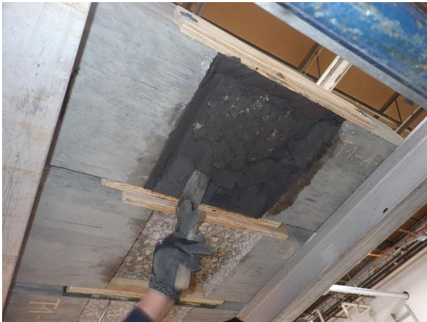
Figure C1.15. Hand-application of repair material using a trowel
