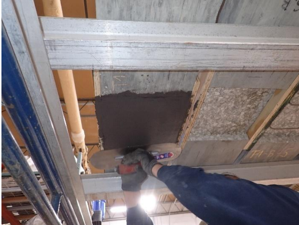
Figure C1.17. Finishing hand-applied patch
