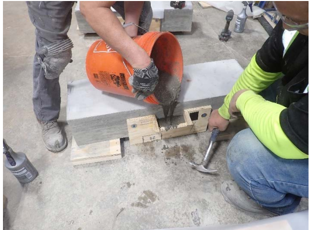
Figure 10. Form-and-pour in overhead orientation
