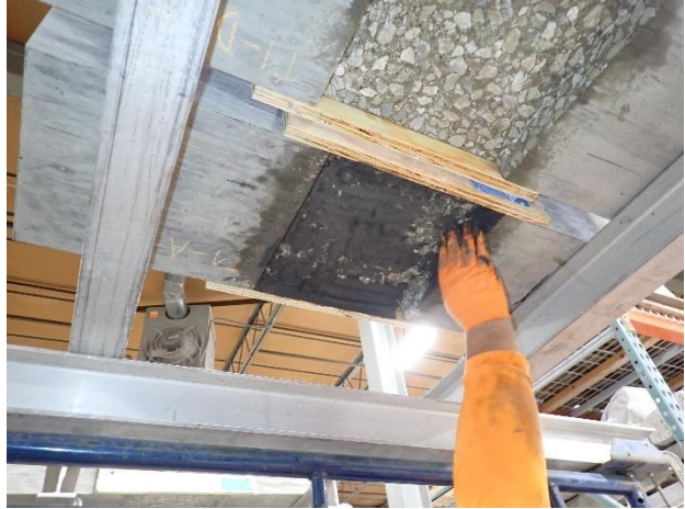
Figure C1.14. Hand-application of repair material
