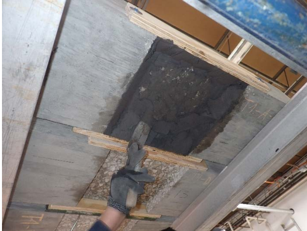
Figure 7. Hand-applied patch in overhead orientation
