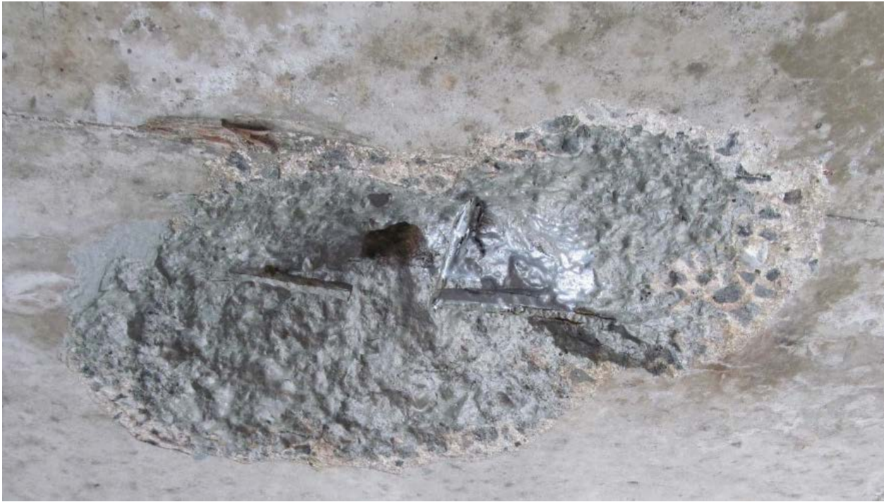
Figure E.1. Example of coating exposed reinforcement
