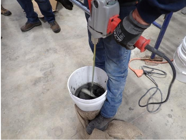
Figure C1.13. Mixing hand-applied repair material
