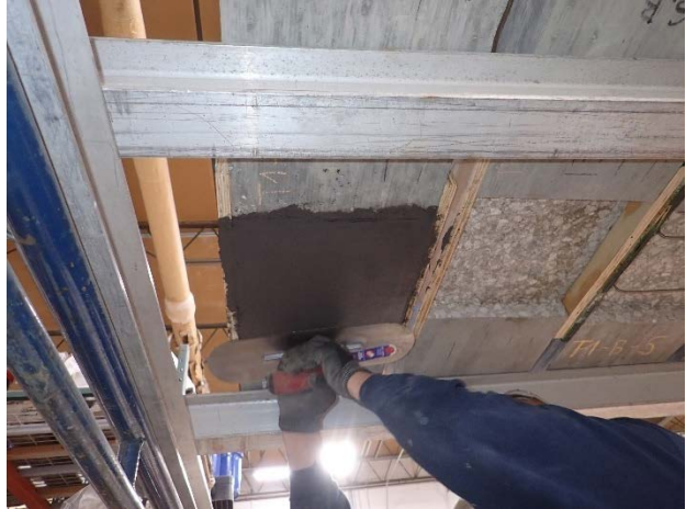
Figure 8. Finishing of a hand-applied patch in overhead orientation
