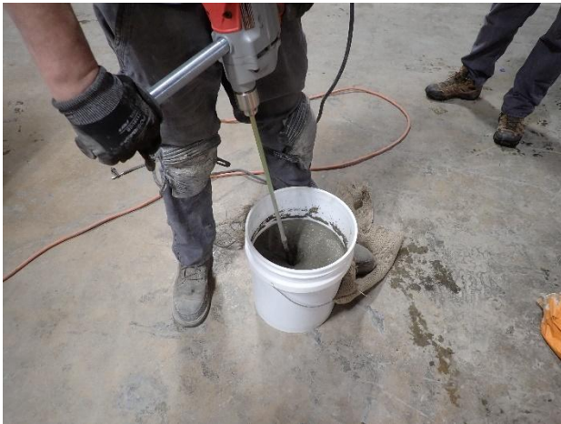
Figure C1.19. Mixing form-and-pour repair material
