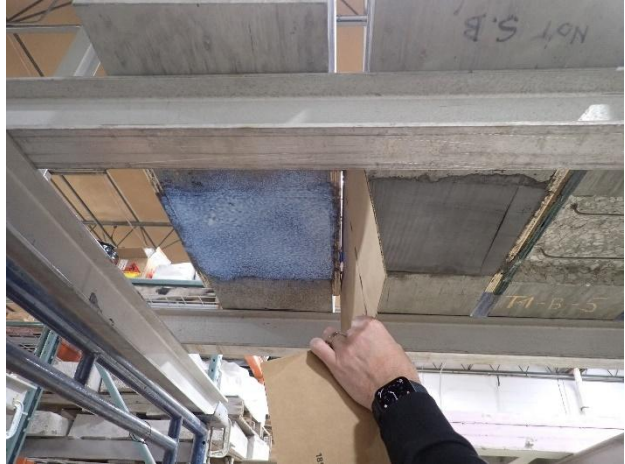
Figure C1.18. Apply curing compound to patch
