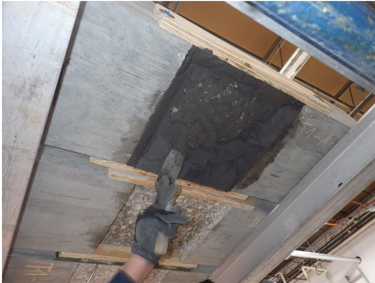
Figure A.1. Example of trowel-applied concrete repair.
