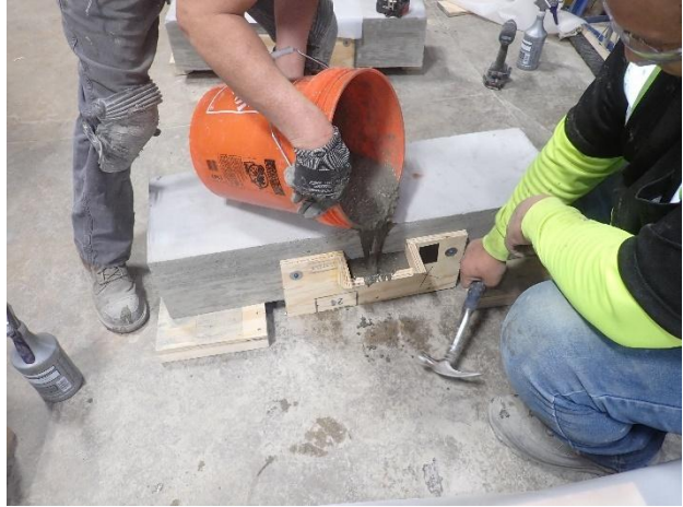
Figure C1.22. Form-and-pour in overhead orientation (patch on the underside)
