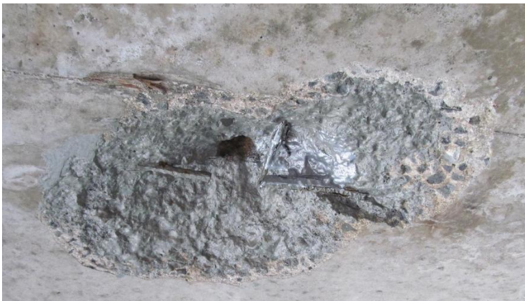
Figure A.5. Coating of exposed reinforcement.
