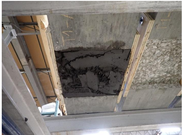
Figure C1.16. Hand-applied patching in progress
