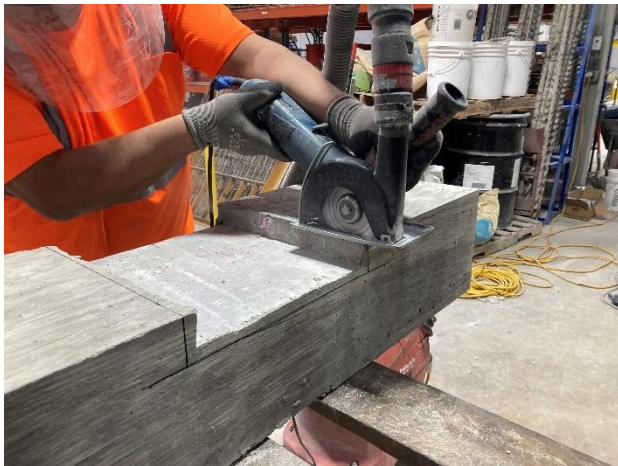
Figure C1.3. Sawcut edges of repair area
