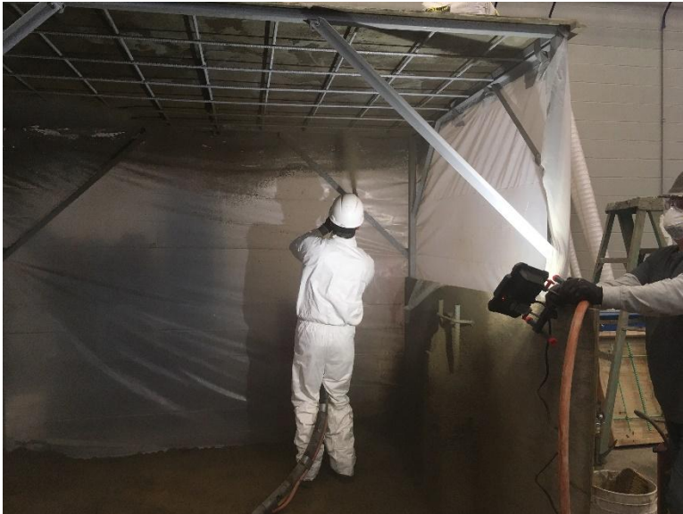
Figure A.3. Illustration of shotcrete repair
