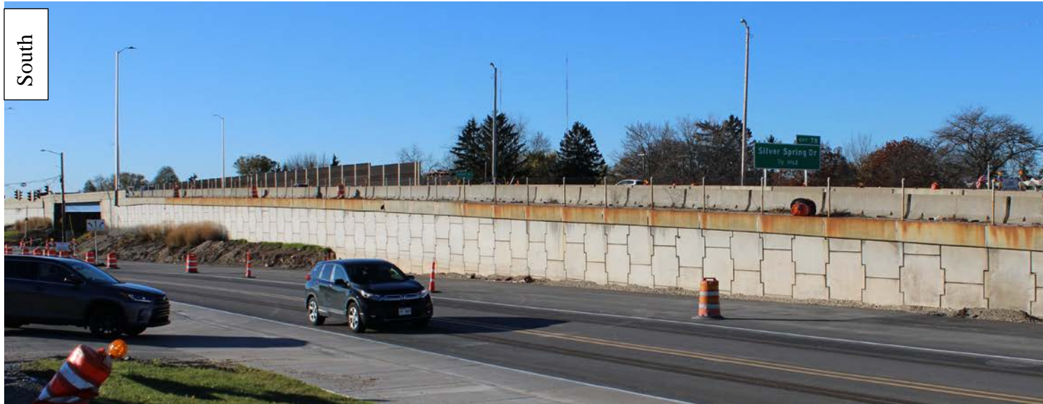
Figure 11. Photograph taken in November 2023 showing the MSE wall facing.
