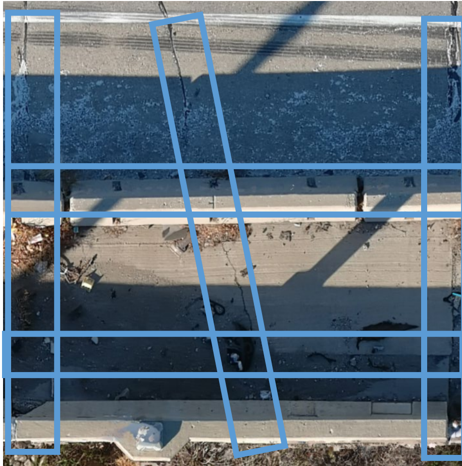
Figure 35. Cracks and concrete joints considered for calculation of crack infiltration rate in Section 1.
