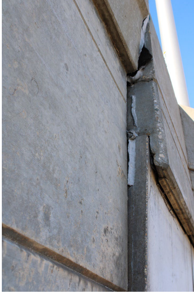
Figure 14. Relative movement of the concrete coping and concrete panel at the south end of the MSE wall to the bridge abutment wing.
