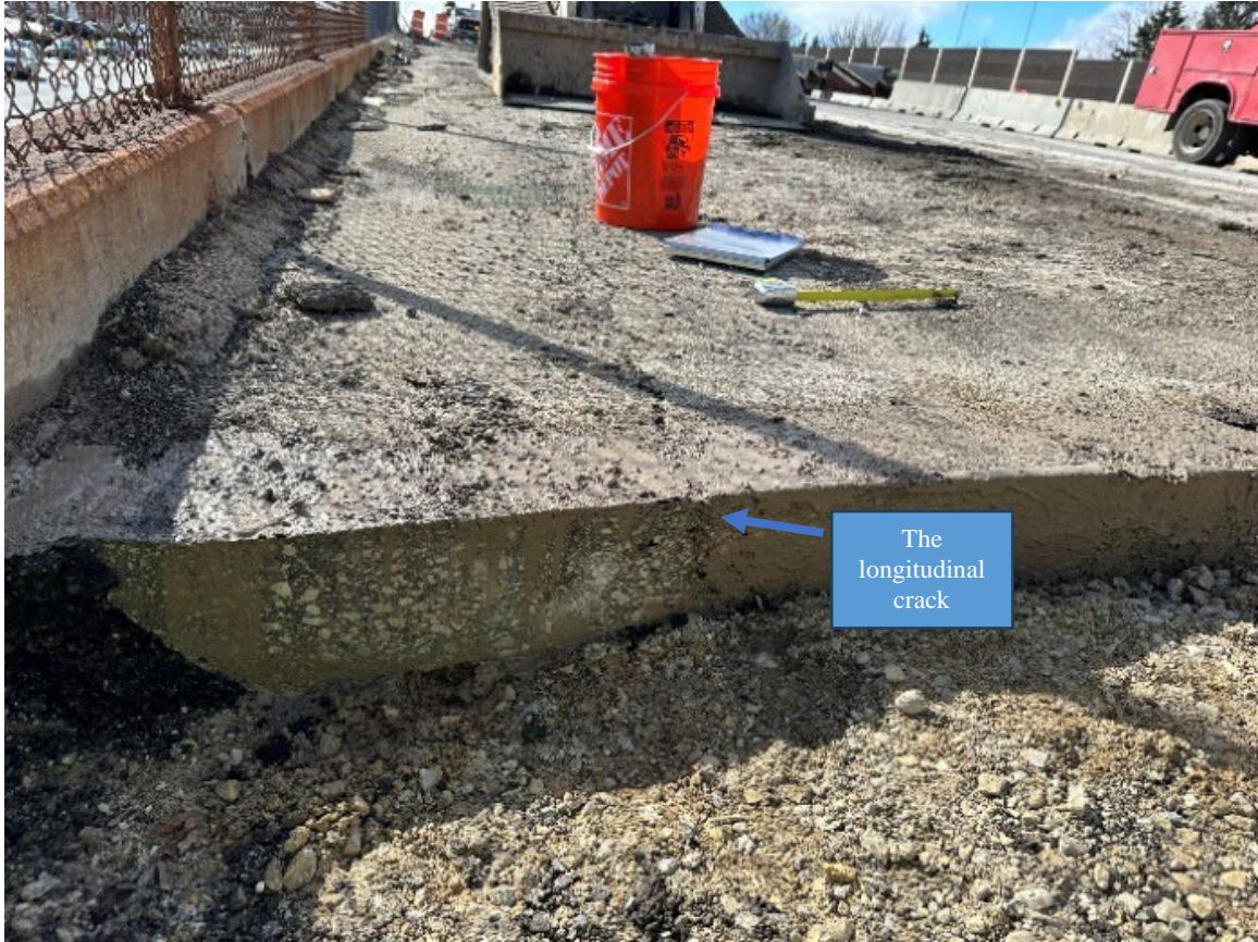
Figure 21. The longitudinal crack on the shoulder pavement along the MSE wall at Section 3.
