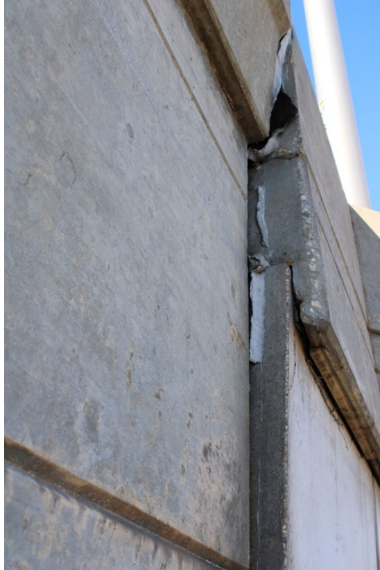
Figure 45. The 4-inch outward displacement of the top panel immediately next to the bridge abutment.
