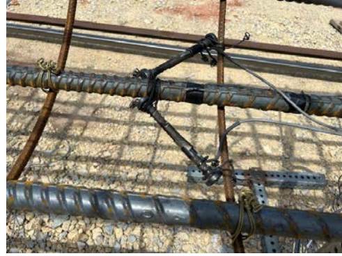
Figure 3-8. Installation of headed bars on the reinforcement cage
