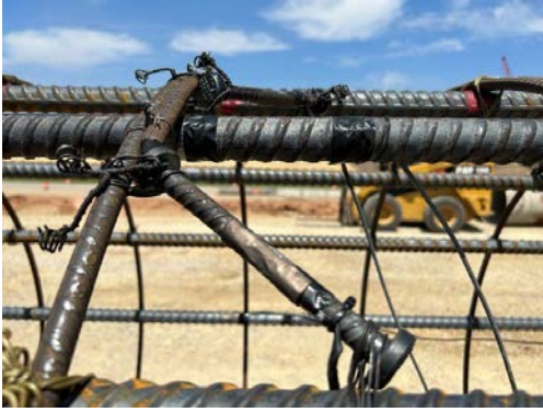
Figure 3-8. Installation of headed bars on the reinforcement cage
